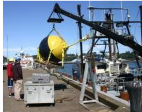
Figure 45: Surface buoy load with onboard crane (Hellin 2013-a)
