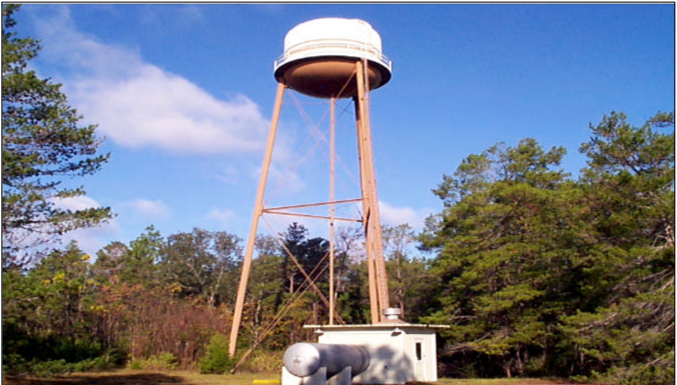
Water Tower and Pump House facing Northeast from Building 8777, Site C-1
