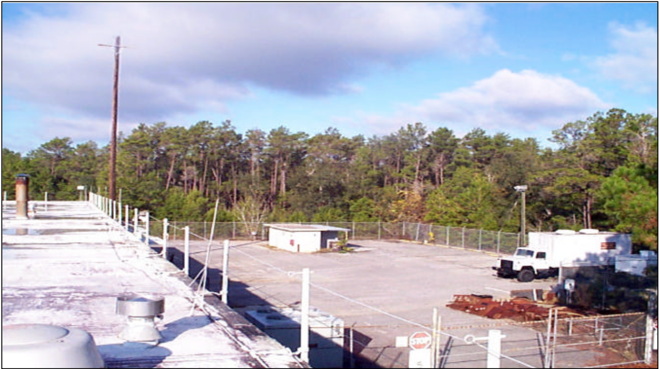
Facing Northwest from the Roof of Building 8777, Site C-1
