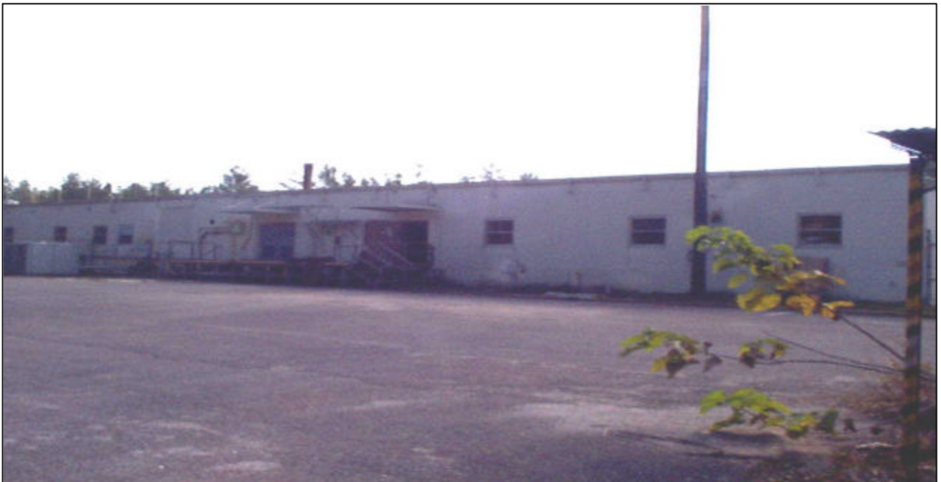
View of the Back of Building 8777 from the North Fence line
