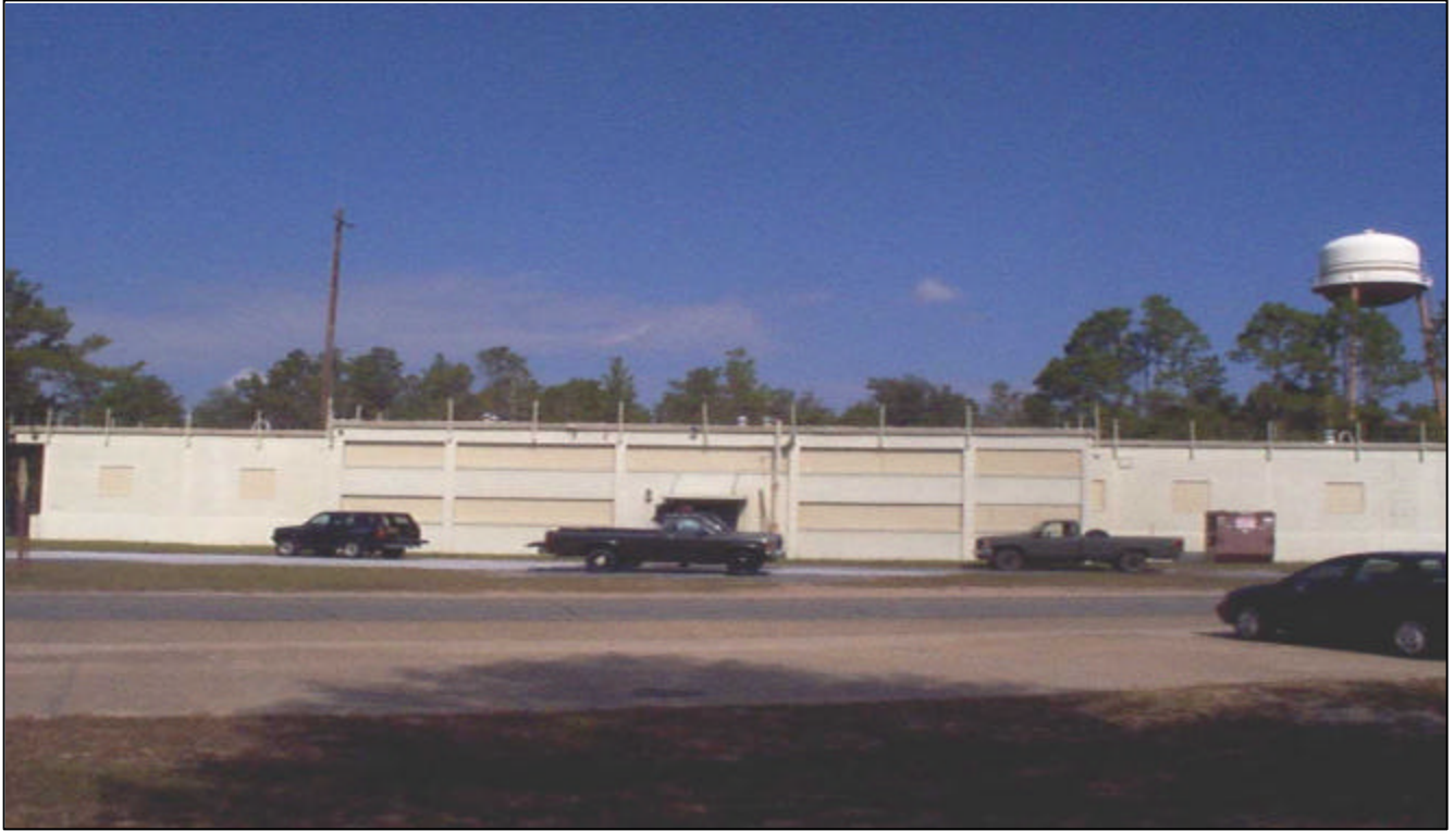
View of the Front of Building 8777 from Range Road 218
