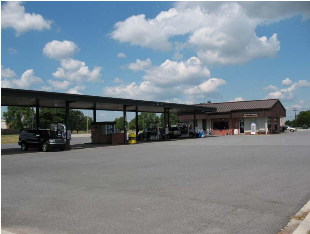
1) Preferred Alternative Site: Existing Shoppette (Building 517).
