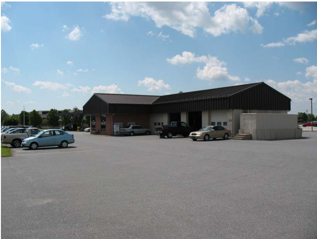
2) Preferred Alternative Site: Existing Shoppette (Building 517).
