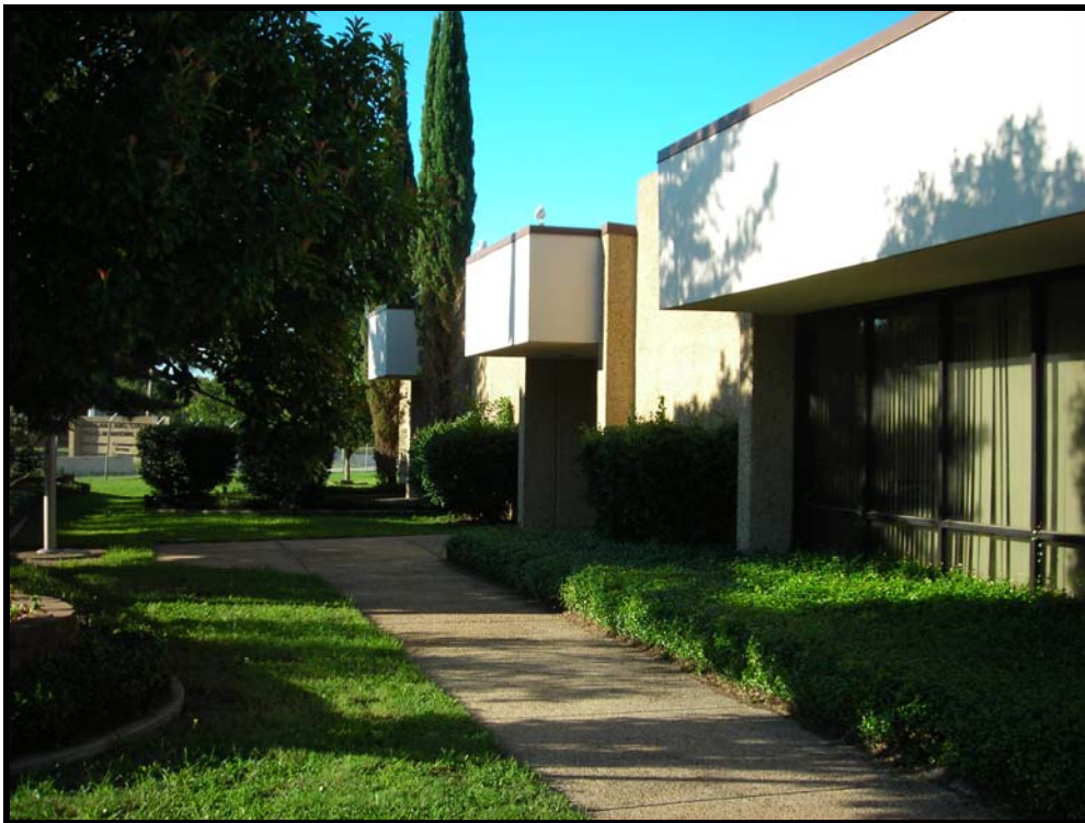
Photo 1: Building 1 – East Facade
