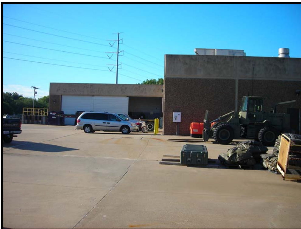
Photo 5: Building 5 – North Side
