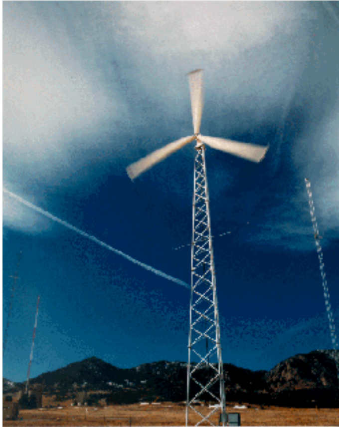
Photo 1 – Typical 50-kW Wind Turbine
