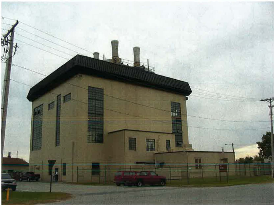
Figure 1-3. Central Heat Plant
