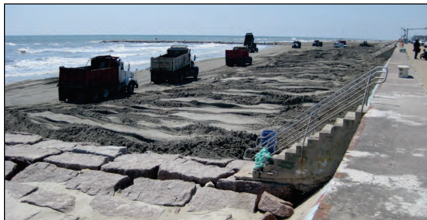
b. Mining of Big Reef and back-passing sand to the south (20 March 2009).
