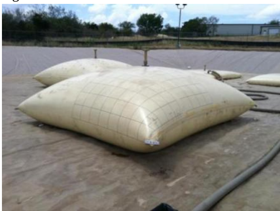
Figure 4.2.2 – Corner View of Typical Standard Design Tank
