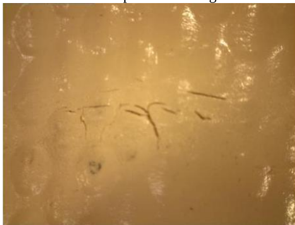
Figure 6.2.79 – Close up of external face showing compound cracking
