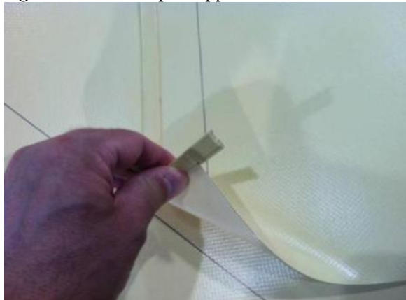
Figure 4.5.9 – Cap-Stripped End of Curved Panel
