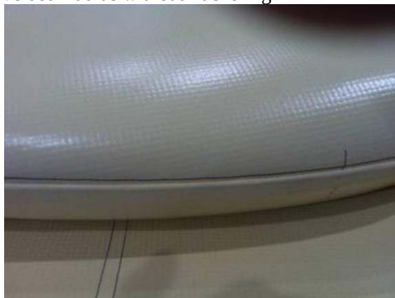
Figure 4.5.11 – Completed Welded Radius without Puckering
