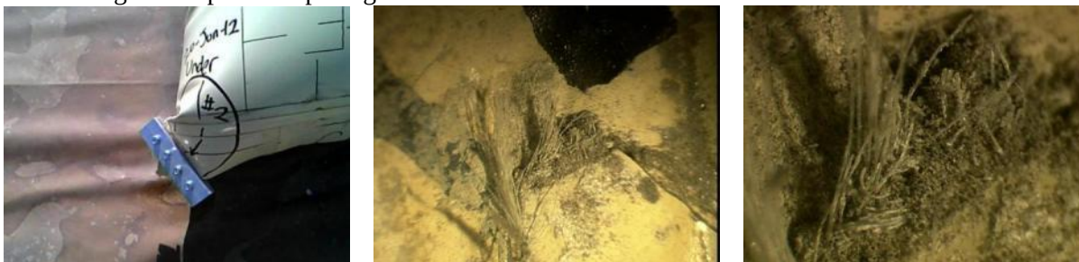
Figure 5.4.80 – Class II – T20-2 – Corner – 20 JUN 12 Over welding of compound exposing scrim in corner
