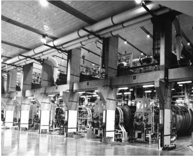
Figure 9-AI-1. View of the Enrichment Plant before Dismantlement. 9
