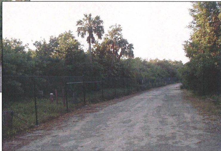
Looking south along Rescue Road. Landfill No. 5 is the area beyond the fence along the left (east) side of the road.
