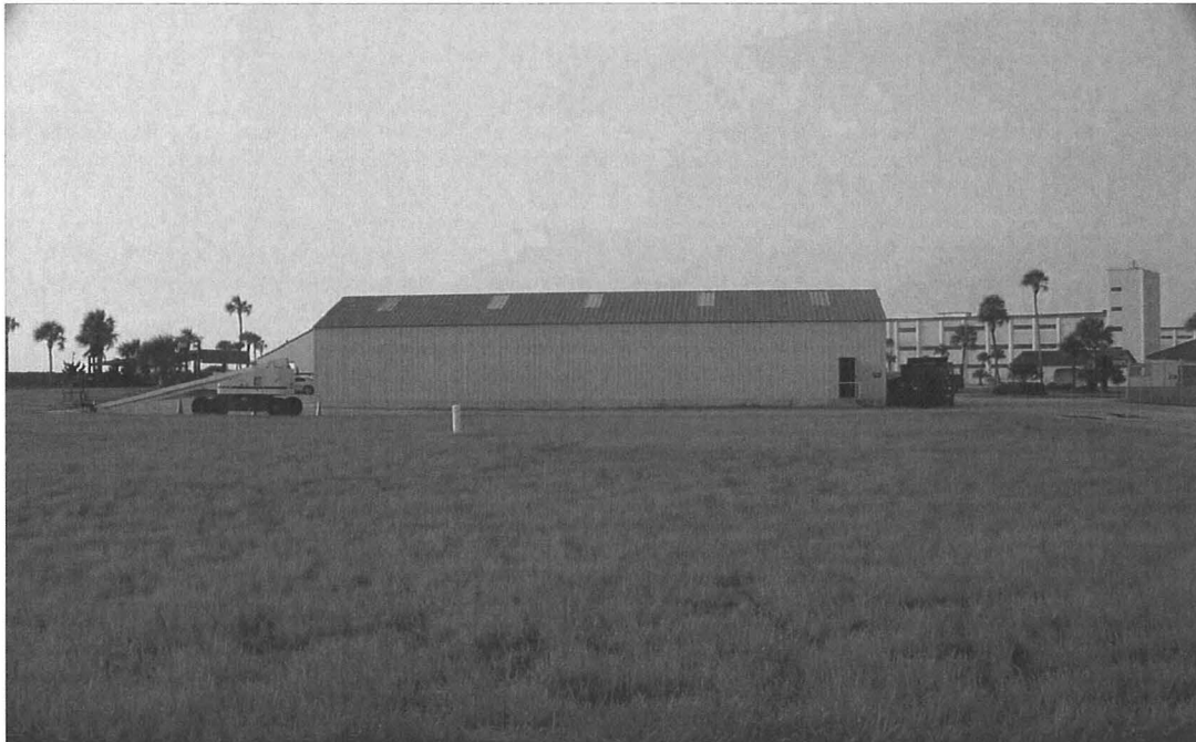
The grassy area in this photo is the former location of the Paving and Grounds Facility. As part of the IM the building was demolished. This photo was taken from near the corner of South Patrick Drive and Maintenance Road facing south toward Building 960.
