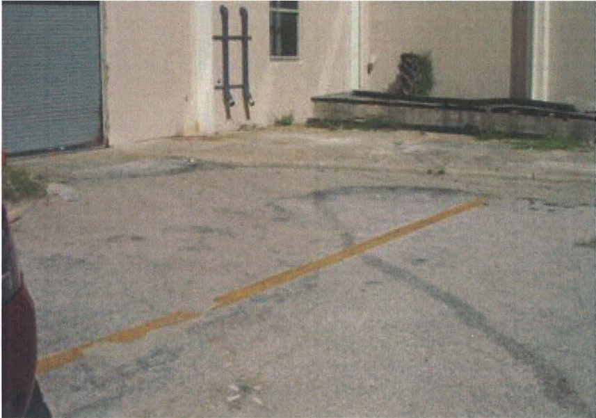
Current site conditions at the location of the former transformer.
