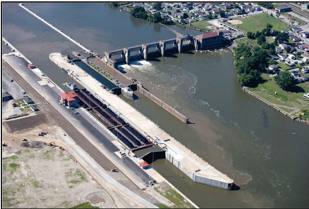
Figure 2. Marmet Locks and Dam, Kanawha River, West Virginia.
