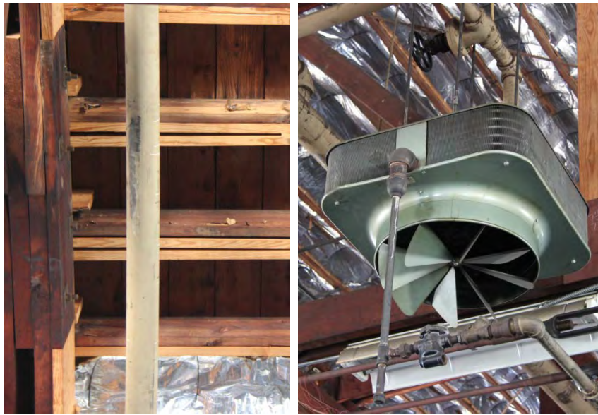
Hot water pipe hung from the roof (left) and ceiling hung hot water heater (right).
