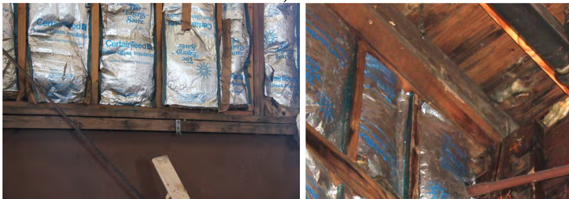
Exterior wall framing details, note column (left) and window header detail (right).
