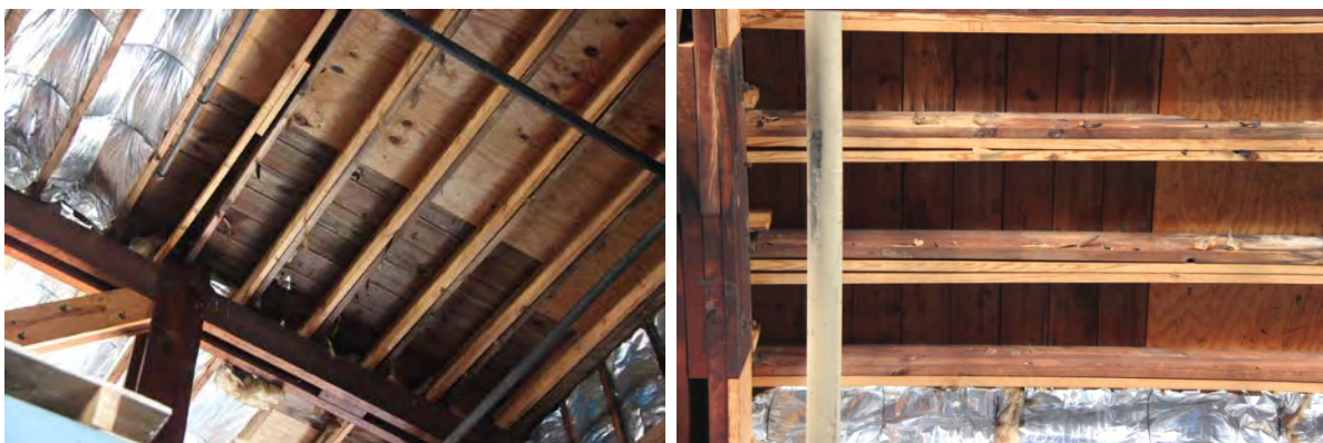
Roof frame and deck repair/replacement (Note: multiple new rafters "sistered" into existing rafters).
