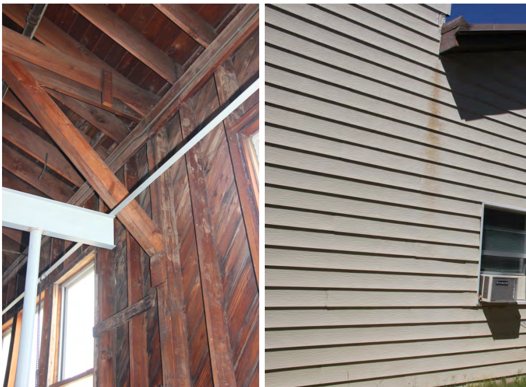
Exterior wall framing and sheathing (left, note 6x6 column and 2x8 ledger) and exterior steel siding.
