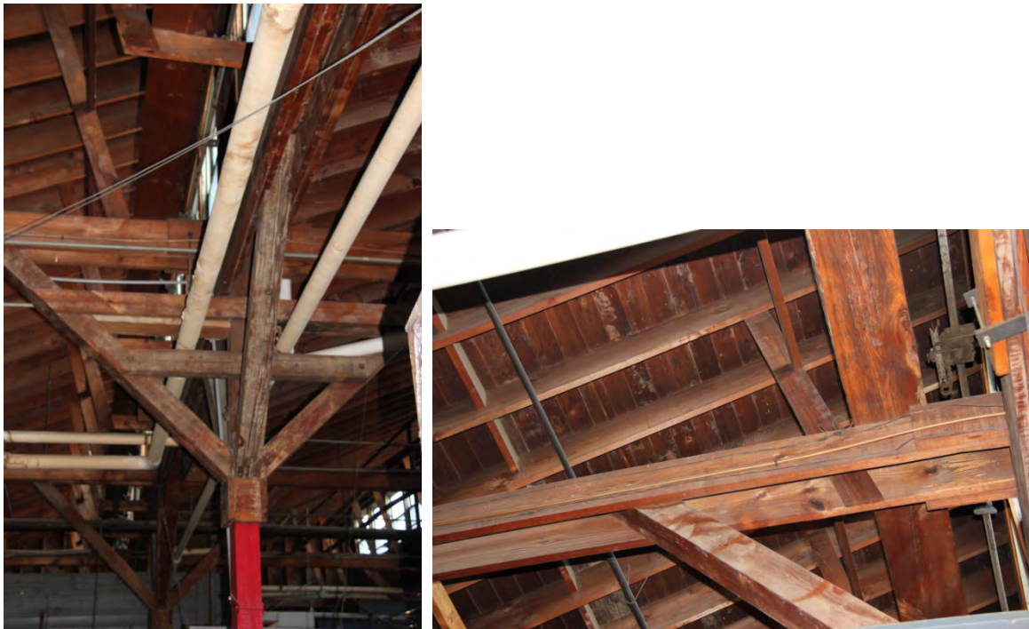
Diagonal bracing (left) and horizontal bracing (right) at columns.
