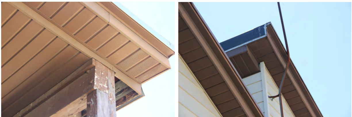
Aluminum soffit and fascia at loading dock (left) and at clerestories (right).
