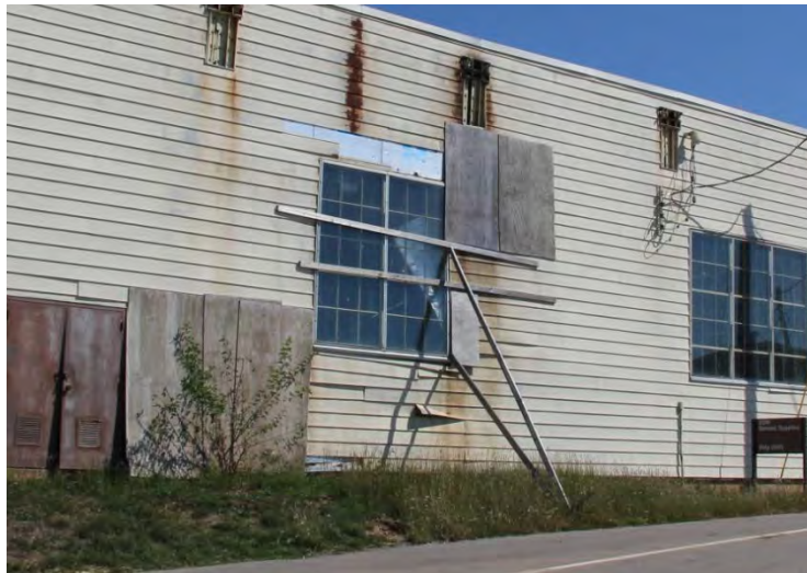
Shoring at the south wall.
