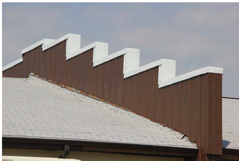
Aluminum soffit, gutters and exterior cover panels.
