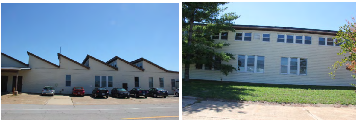
Building 2352 west (left) and north (right) elevations.
