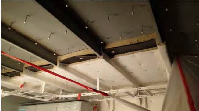
Mass Loaded Vinyl in Eng Space Overhead – Sally Ride
