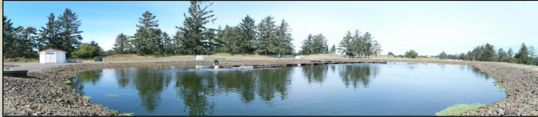
Primary Lagoon for WWTP
