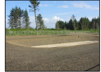
WWTP rapid infiltration basin #1 (of 4)
