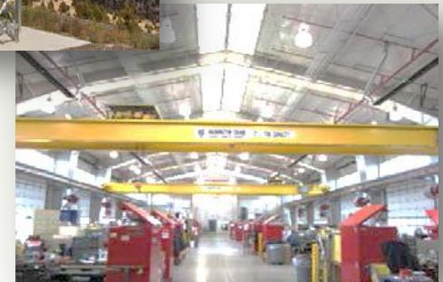
Camp Withycombe Industrial Lighting
