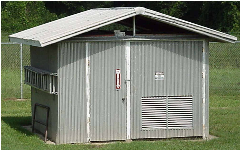
Photo 2: Hazardous Materials Storage Shed to be Demolished
