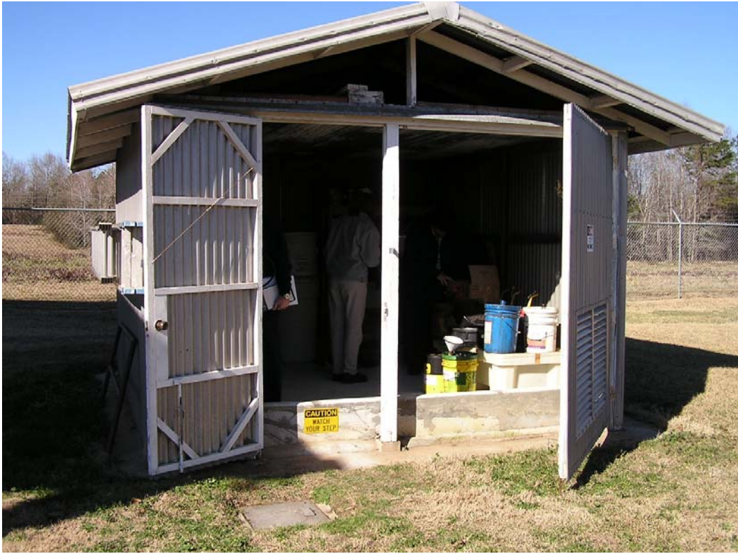
Photo 1: Hazardous Materials Storage Shed to be Demolished
