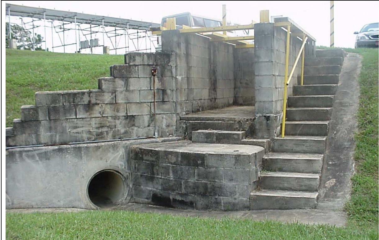
Photo 3: Oil Change Pit to be Demolished
