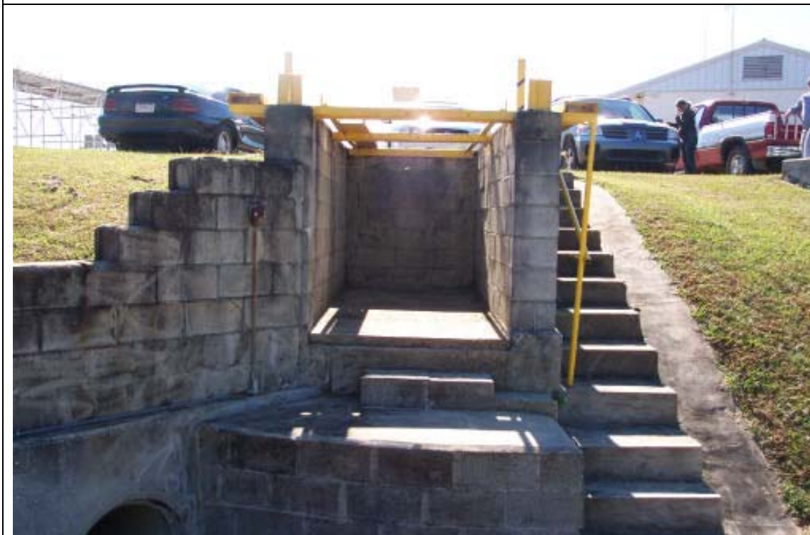
Photo 4: Oil Change Pit to be Demolished
