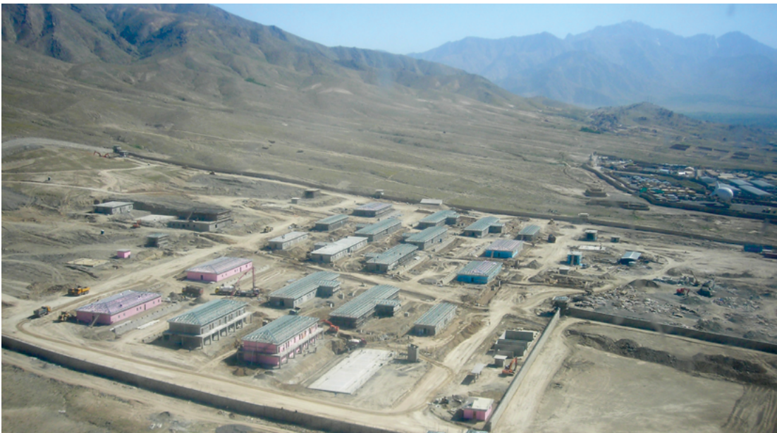
Figure 5: Facilities Construction at the National Logistics Center Source: DoD IG-SPO
