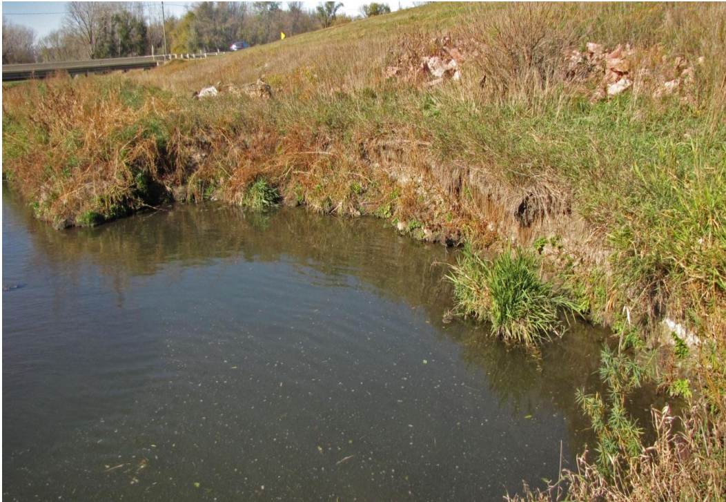
Figure 7. Right bank scour and vegetation located downstream of sheet pile control structure. Photo taken October 31, 2014.
