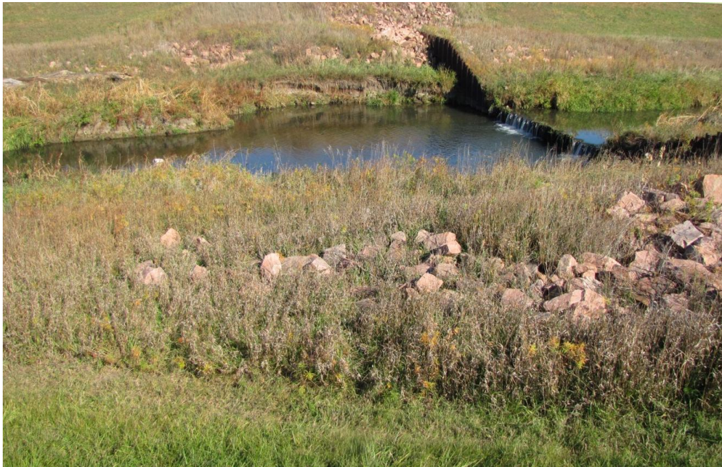
Figure 8. Upland vegetation of both left and right banks in areas previously disturbed by rock. New riprap will be placed in areas where rock once existed to restabilize the banks. Photo taken October 31, 2014.
