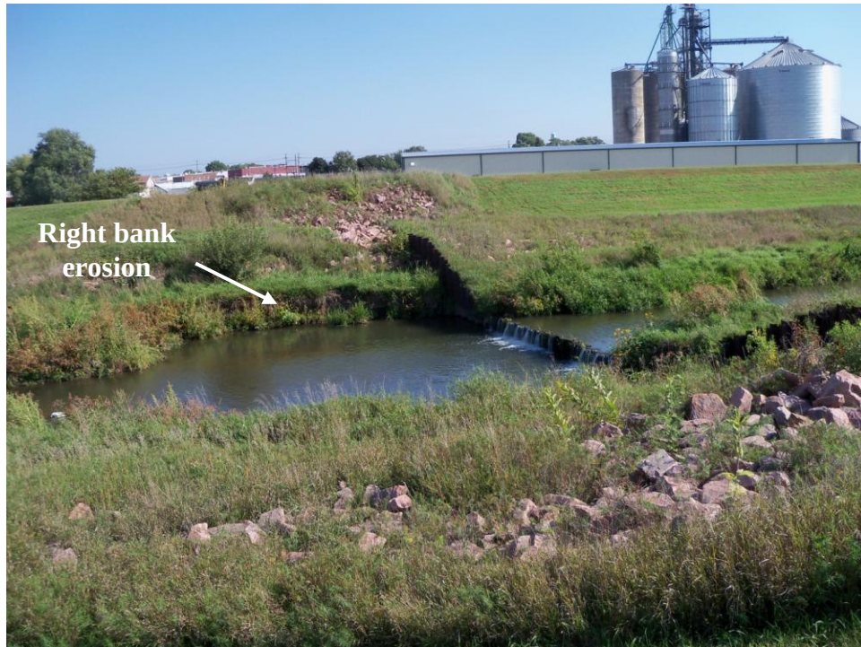
Figure 4. Right bank erosion downstream of the sheet pile control structure at Dry Creek.
