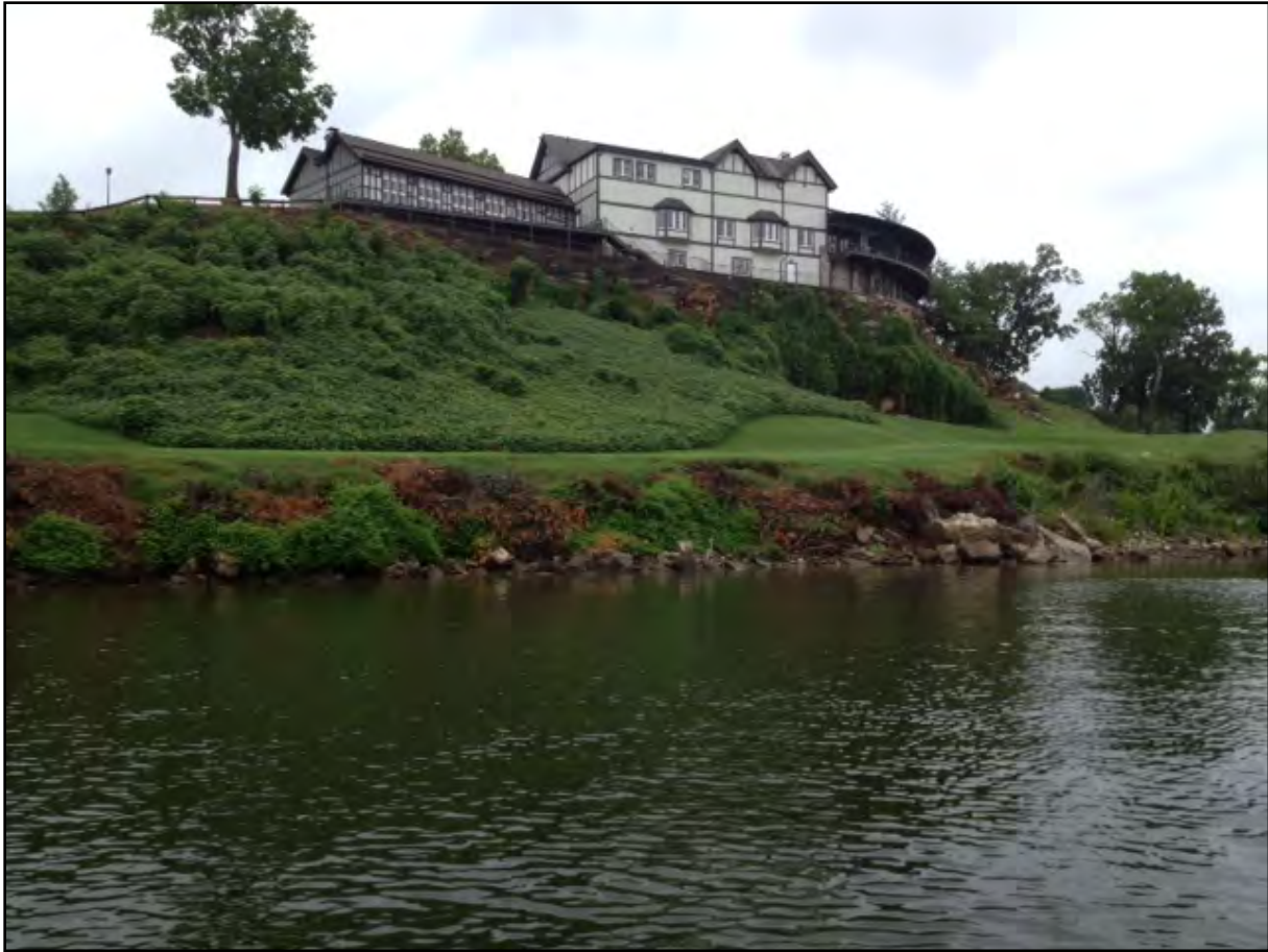
Figure 7 – Riverbank at Approximate TRM 466
