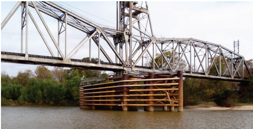
Figure 4. Left pier, cell, and fender structure intended to protect against vessel impacts, looking upstream at the Norfolk Southern railroad bridge near Jackson, AL.
