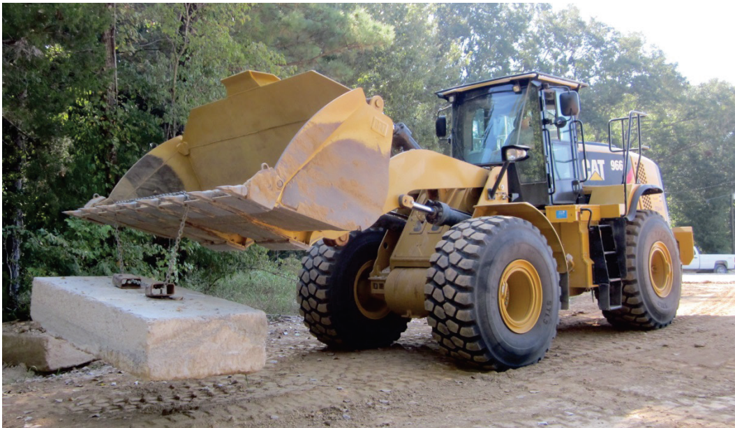
Figure 57. Successful lifting of PCC using the teeth on the front-end loader.
