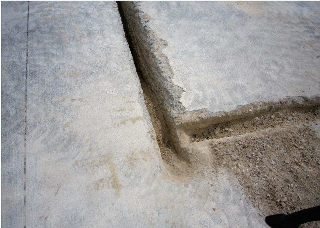
Figure 47. Crater 2, not fully sawed at corners.
