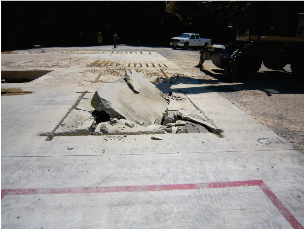
Figure 49. Crater 9 with 3-in. to 8-in. overcuts and PCC attached at corners.
