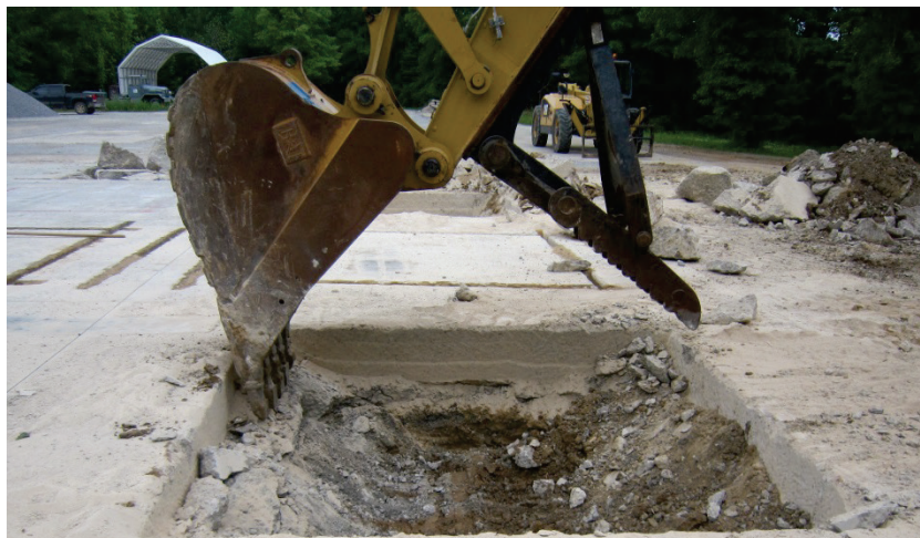
Figure 15. Excavator 36-in.-wide bucket.
