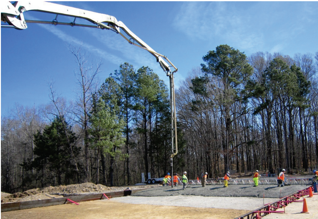
Figure 3. PCC placement using pump truck.
