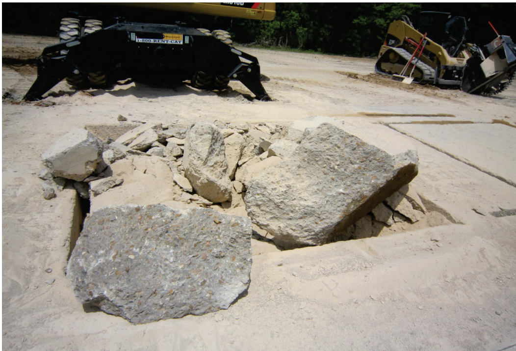
Figure 43. Crater 10, with no overcuts and less-than-full-depth cuts.
