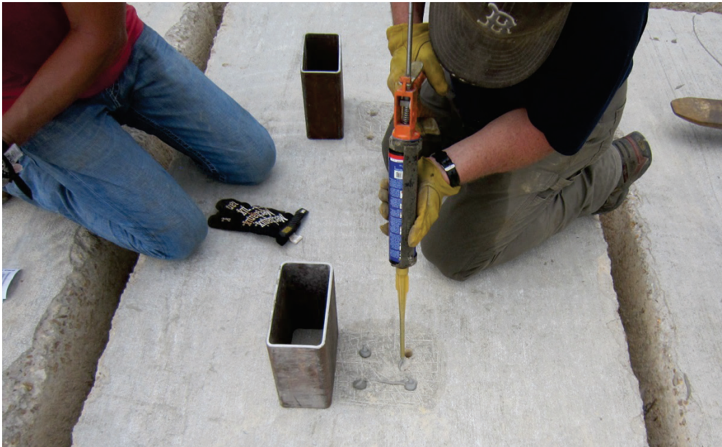
Figure 52. Four drilled holes filled with epoxy.
