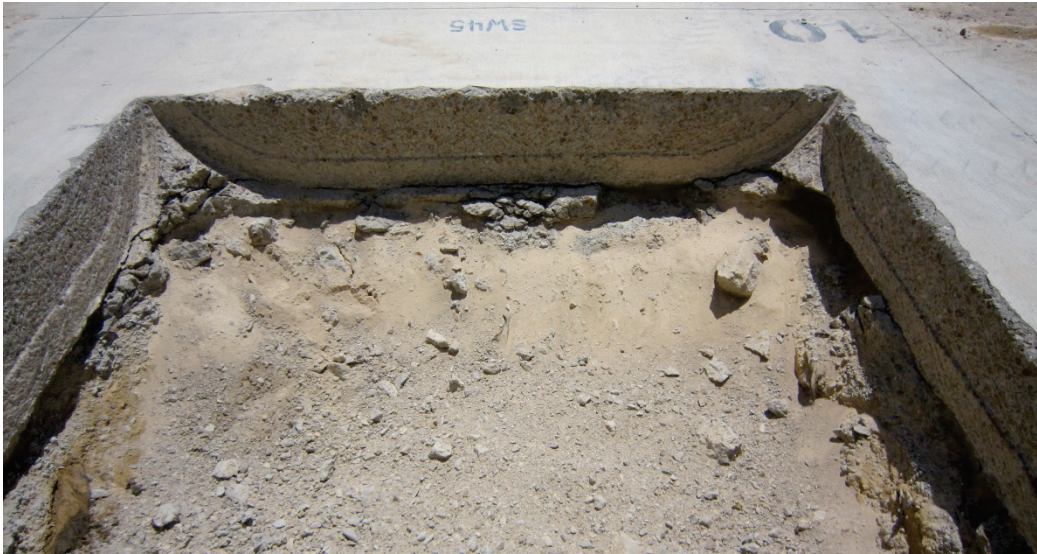
Figure 44. Crater 10, with attached PCC at the corners.
