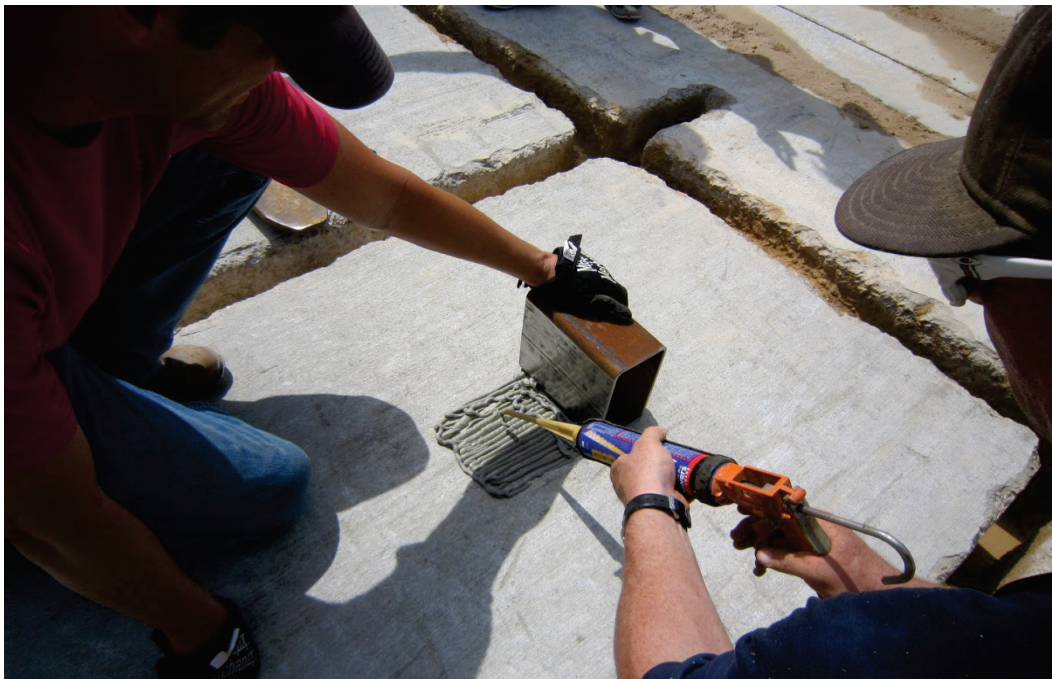
Figure 50. Application of epoxy below steel box beam.
