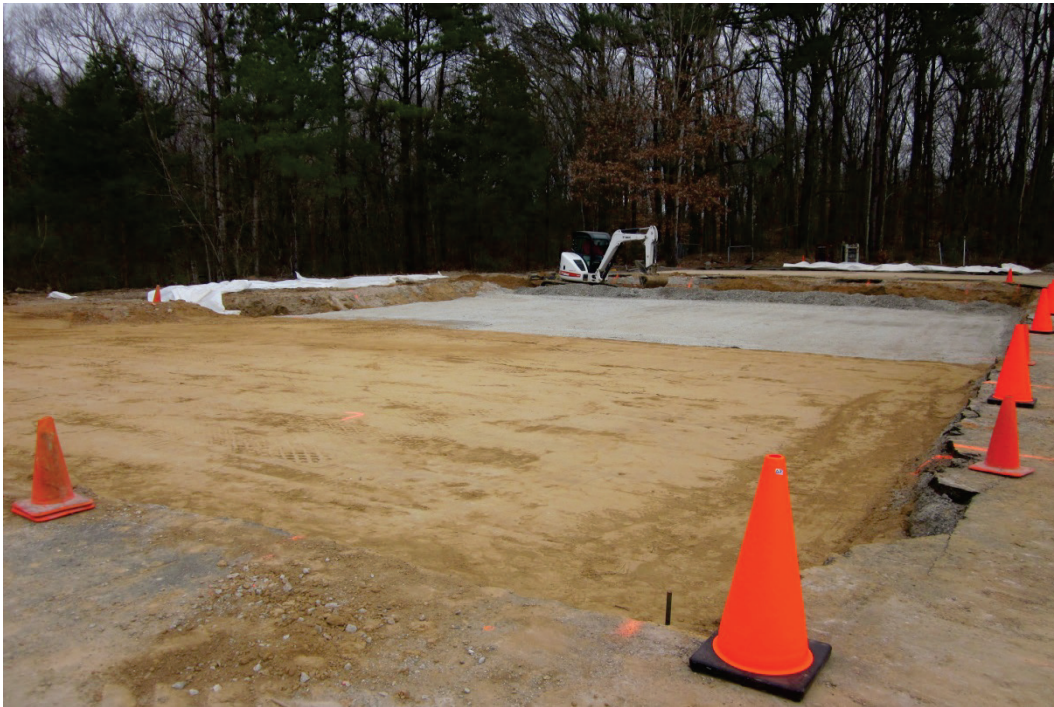
Figure 2. Test site construction preparation.
