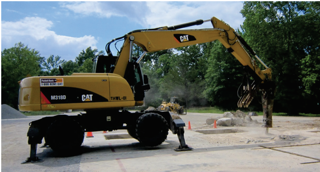
Figure 14. Caterpillar M318D excavator with H120E hammer.
