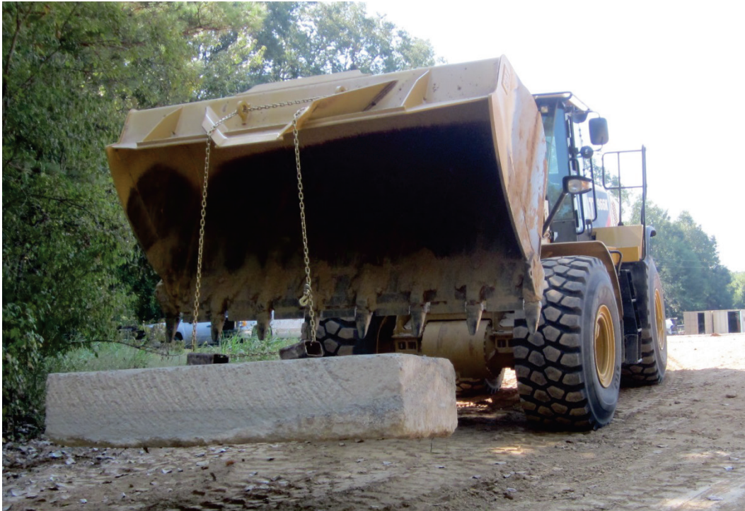
Figure 56. Successful lifting of PCC using eye holes on the front-end loader.
