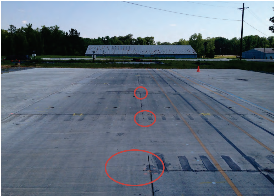
Figure D.5. Saw cuts at corners of panels.
