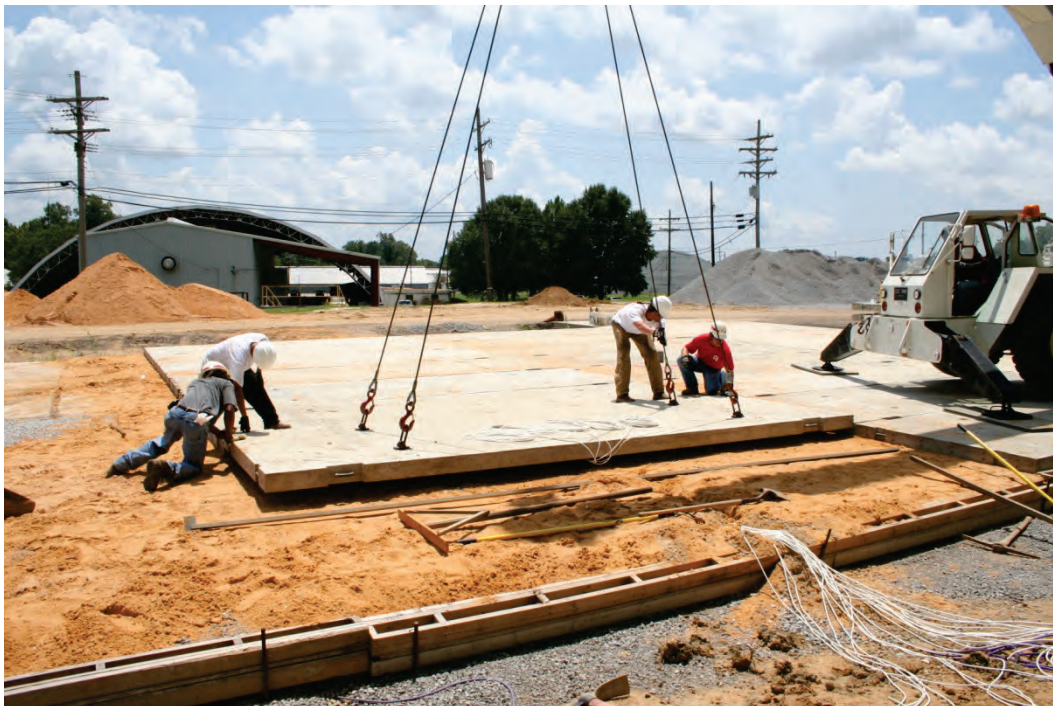
Figure A.3. Placement of a precast panel.
