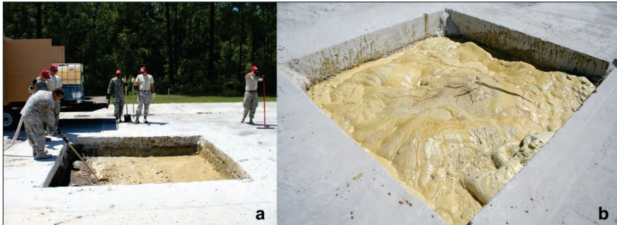
Figure 6.4. (a) Placing foam backfill and (b) hardened foam backfill after 15 min.
