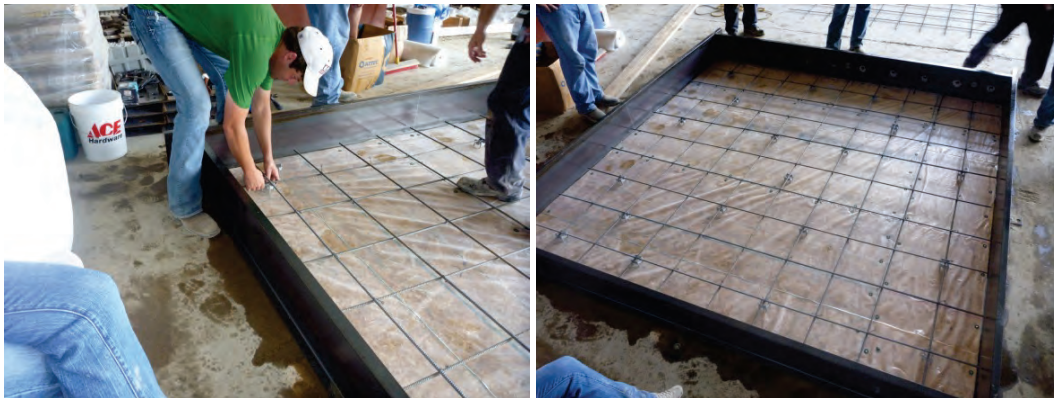
Figure B.9. Installation of rebar grid on chairs.
