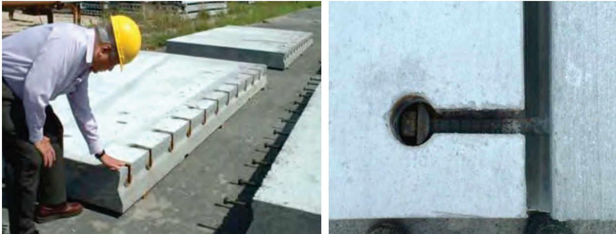
Figure A.8. (left) precast panel and (right) Kwik Joint connection (Kwik Slab 2011).
