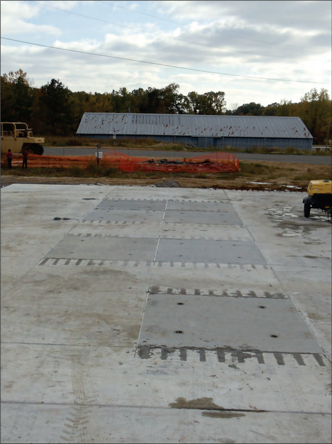
Figure 6.2. Precast PCC panel repairs.
