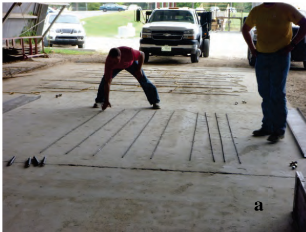
Figure B.8. Assembling #3 rebar grid: (a) spacing bottom layer of rebar, (b) spacing top layer of rebar, (c) tying rebar, (d) tightening ties, (e) tied grid, and (f) placing rebar grid in form.
