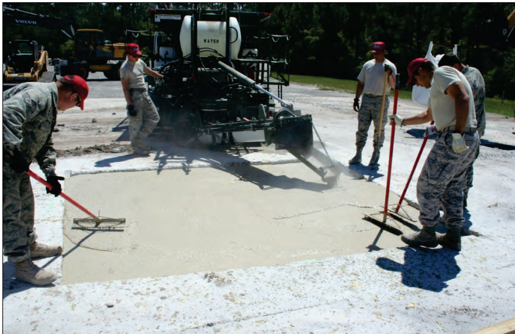
Figure 6.1. Placing rapid-setting cap.
