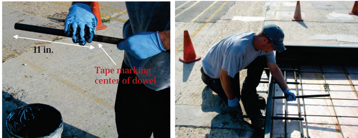
Figure B.10. Installation of the dowel bars.
