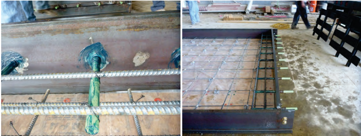
Figure B.11. Locations of the #5 rebar.
