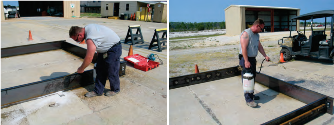
Figure B.7. Spraying release agent on forms.
