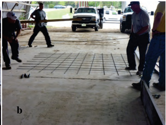
Figure B.8. Assembling #3 rebar grid: (a) spacing bottom layer of rebar, (b) spacing top layer of rebar, (c) tying rebar, (d) tightening ties, (e) tied grid, and (f) placing rebar grid in form.
