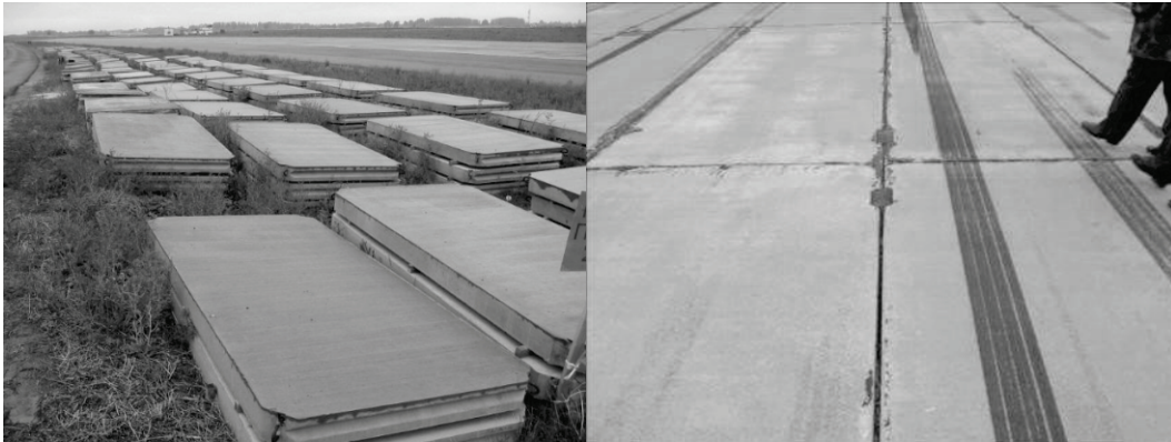
Figure A.2. (left) Stockpiled precast panels at a Soviet airfield and (right) precast concrete panel runway still in service.
