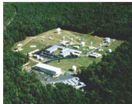
Blossom Point Satellite Tracking and Command Facility.
