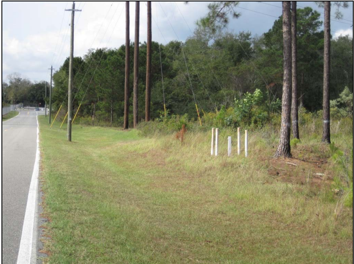
Figure 3-4 View of western end of Stone Road showing inactive power line adjacent to the roadway and larger, guyed poles associated with the Georgia Power easement, which would need to be relocated under the Proposed Action. Also shown is a groundwater monitoring well surrounded by four stakes.
