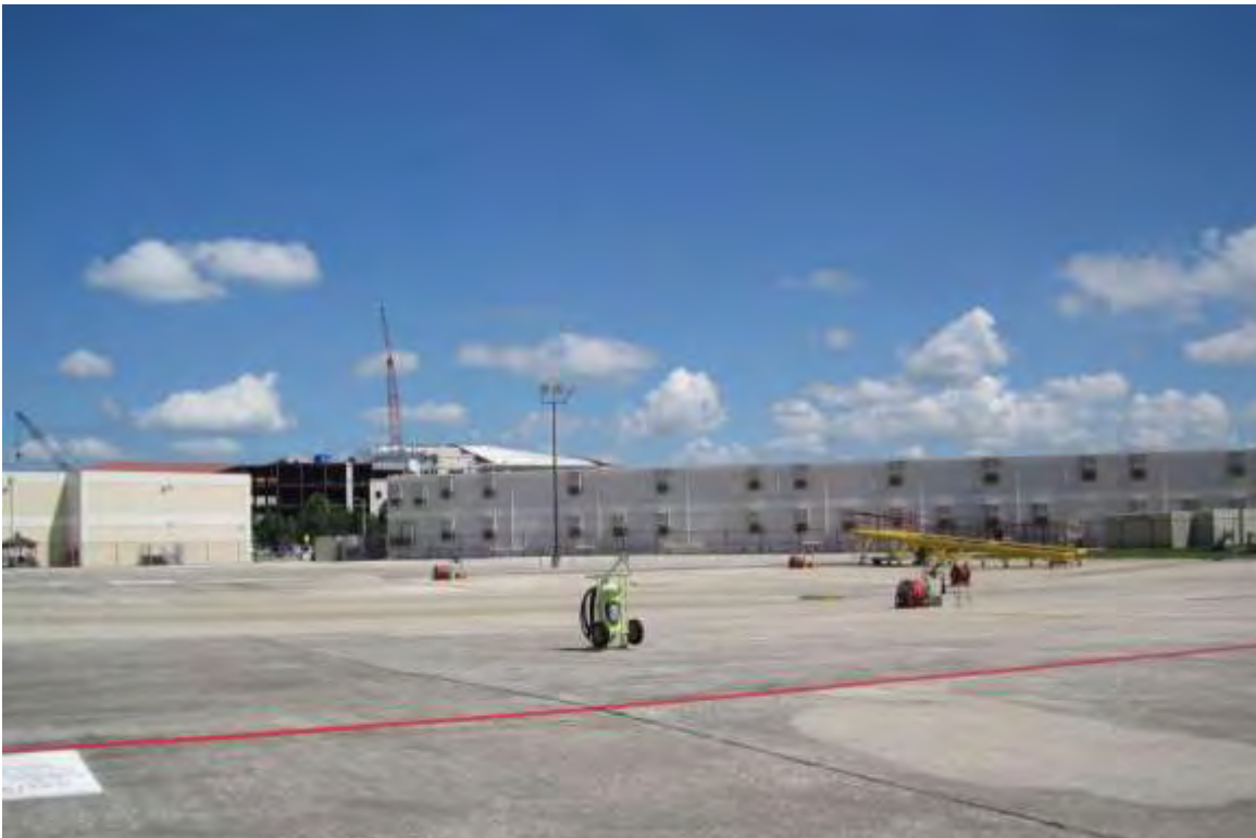
Photo #6: View of the proposed Great Egret Avenue Extension area and Wash Rack looking west.
