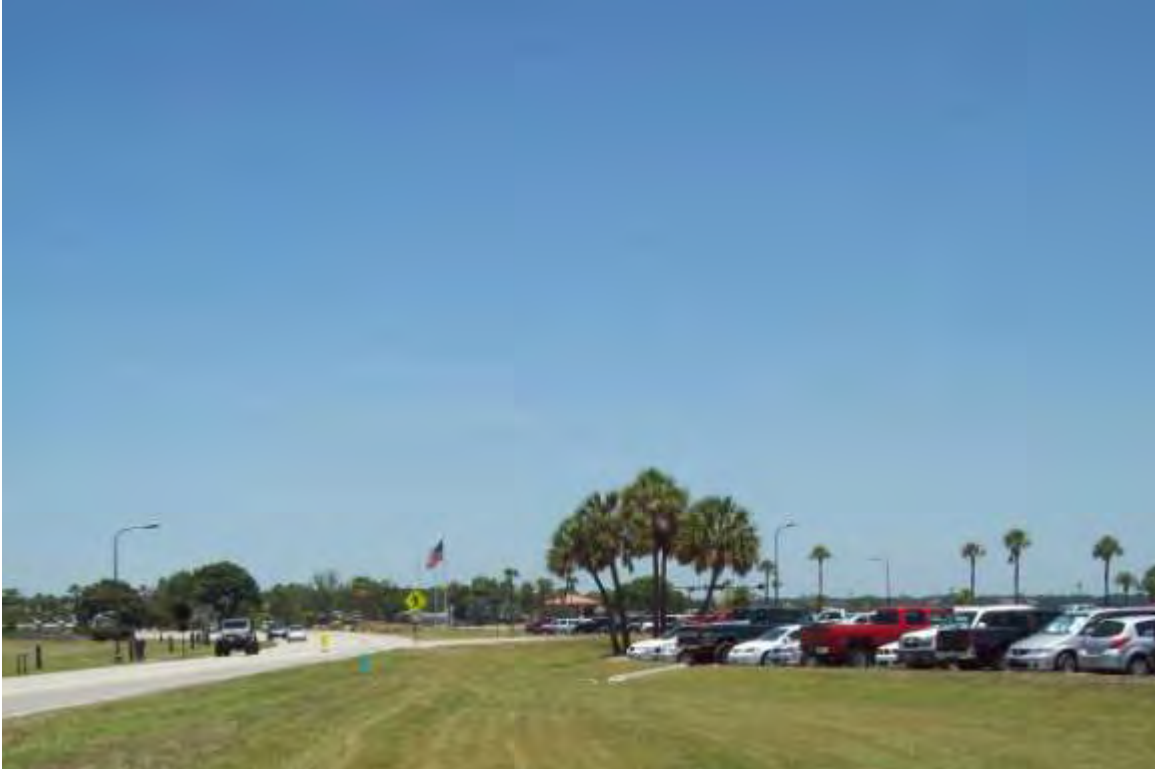
Photo #5: View of the proposed South Boundary Blvd Widening project area looking north.
