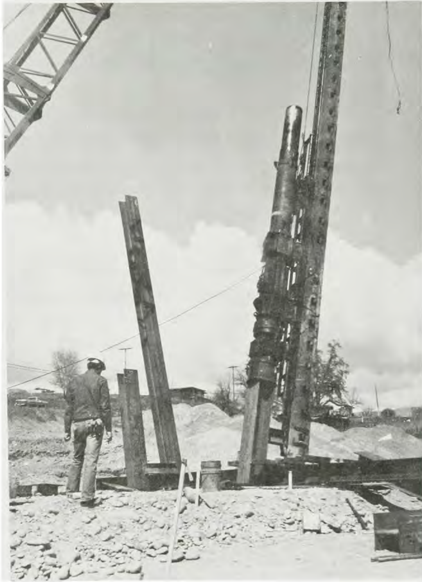
LEWISTON-CLARKSTON INTERSTATE BRIDGE UNDER CONSTRUCTION 1980
