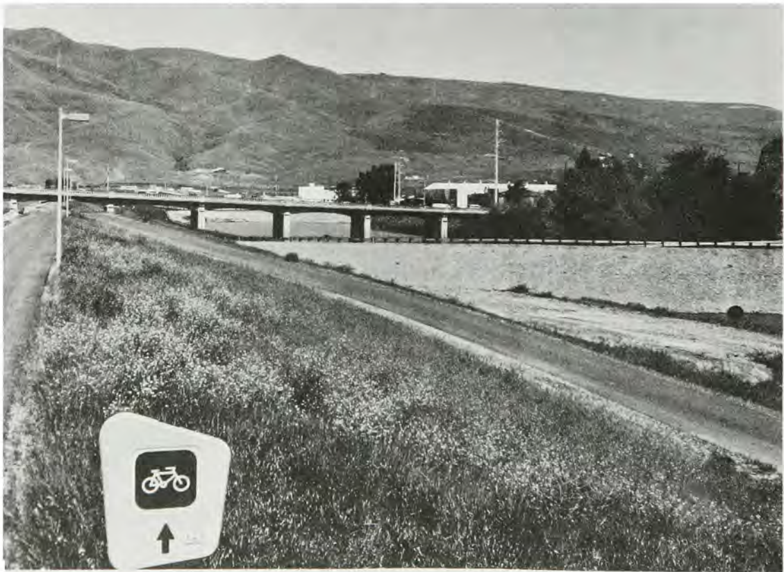
WEST LEWISTON LEVEE
