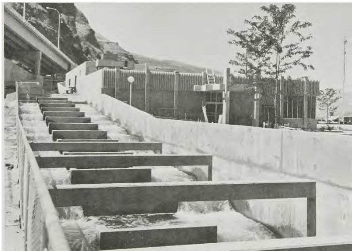
FISH LADDERS AT LOWER GRANITE DAM
