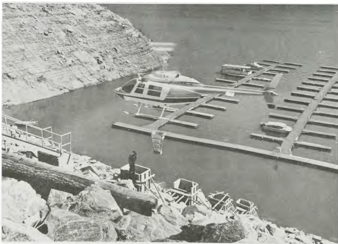
HELICOPTER CARRYING CONCRETE FOR STAIRWAY STEP EXPANSION AT BIG EDDY BOAT MOORAGE AREA DWORSHAK RESERVOIR, 1978
