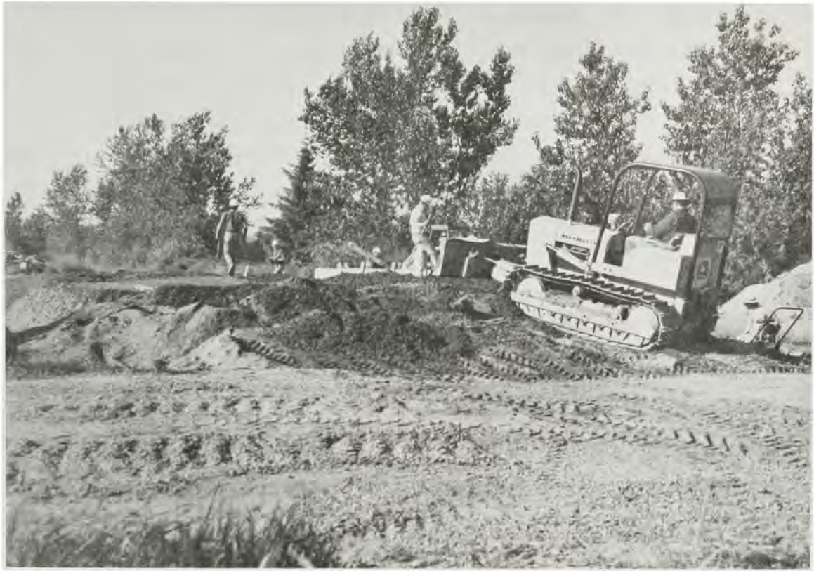
WILLOW CREEK DAM CONSTRUCTION JUNE 1980
