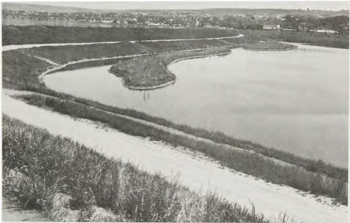
WEST LEWISTON LEVEE
