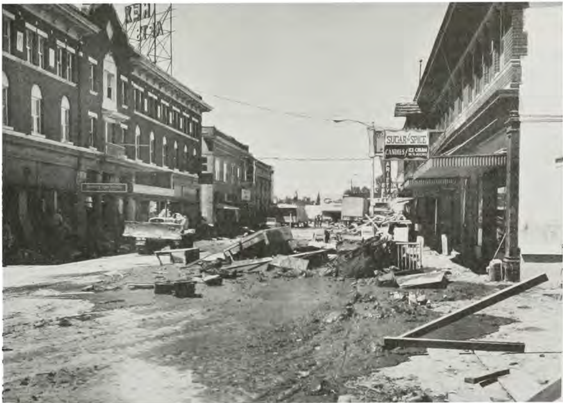
DEBRIS CLEANUP AT REXBURG
