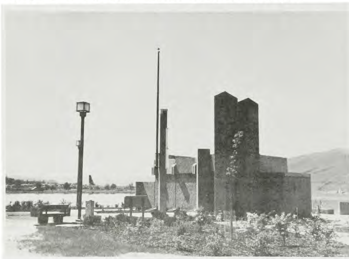
WEST LEWISTON LEVEE
