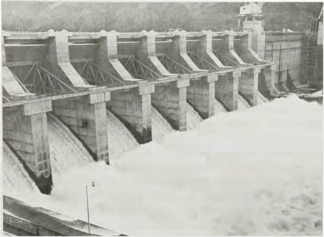
SPILLWAYS AT LOWER GRANITE DAM
