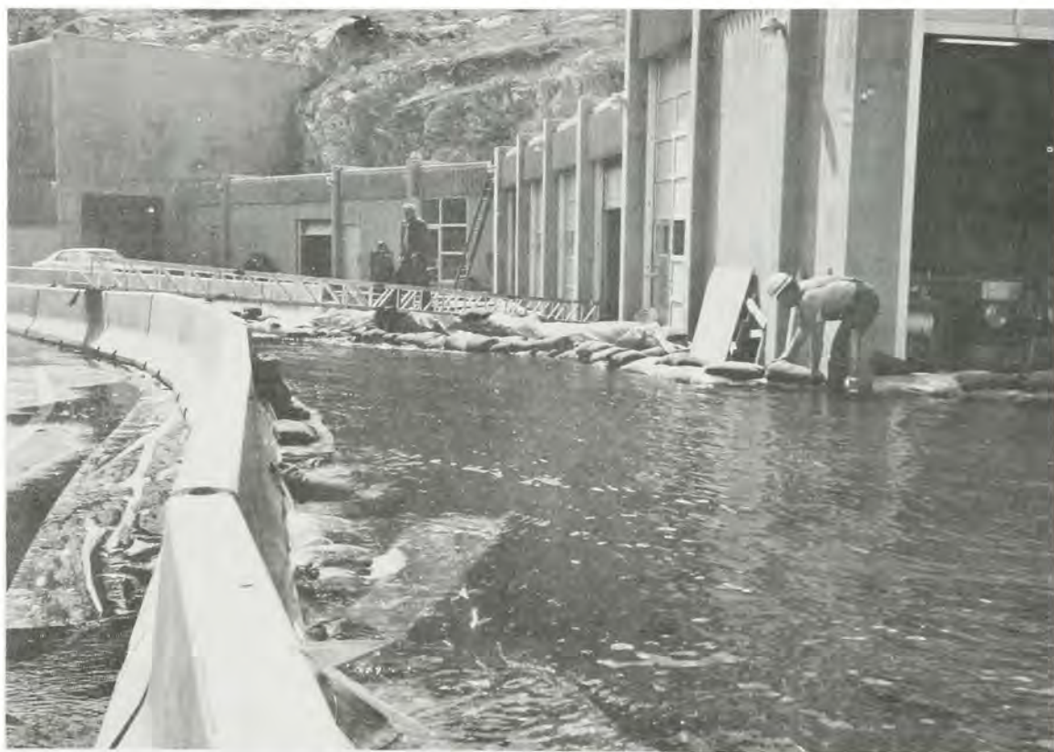
SANDBAGGING FOR TEMPORARY DIVERSION CANAL AT DWORSHAK
