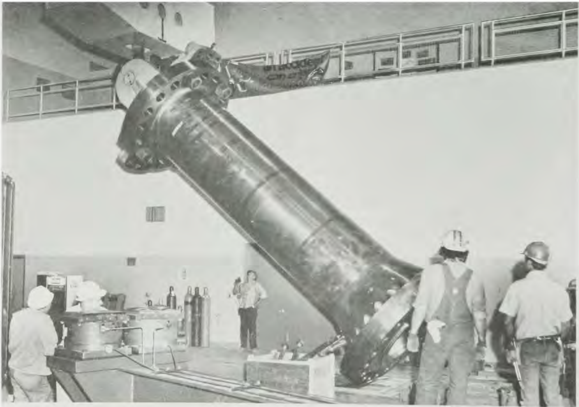
LOWERING THE UNIT 6 INTERMEDIATE TURBINE SHAFT, AT THE LITTLE GOOSE DAM SECOND POWERHOUSE
