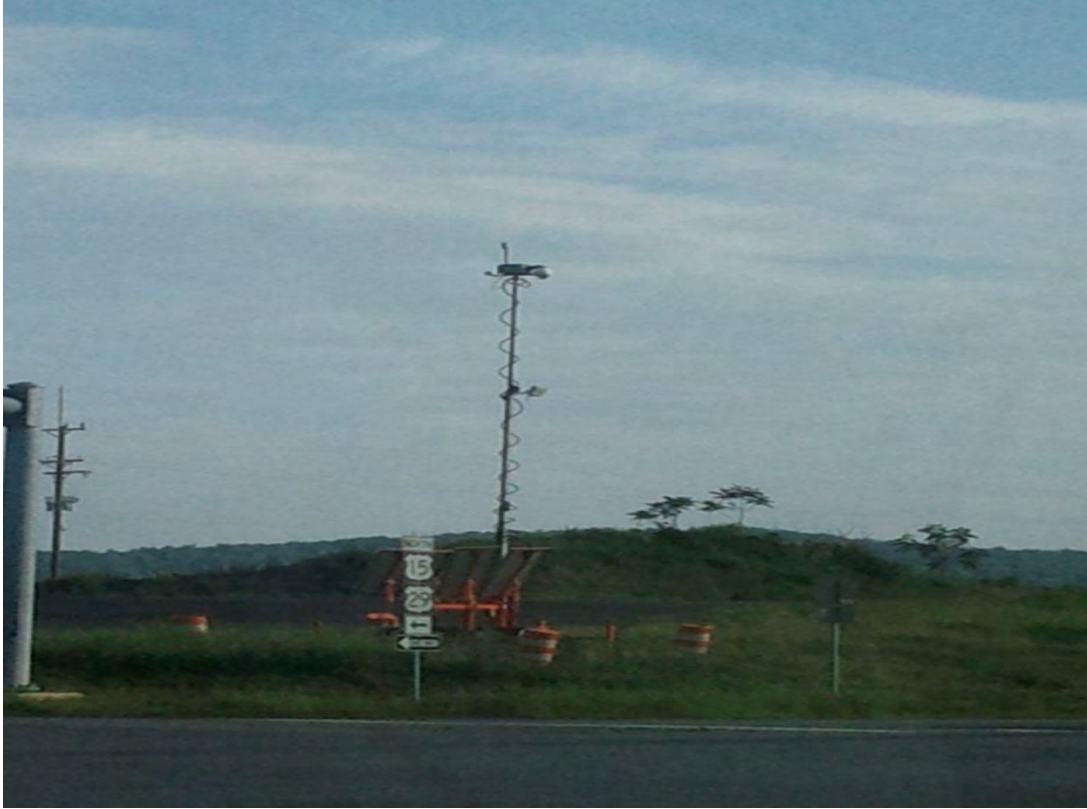
Figure 8. Department of Transportation Camera
