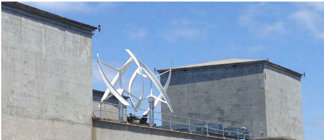
Figure 3. Urban Green Energy (UGE) VisionAIR5 Vertical Axis Wind Turbines on the TPL.
