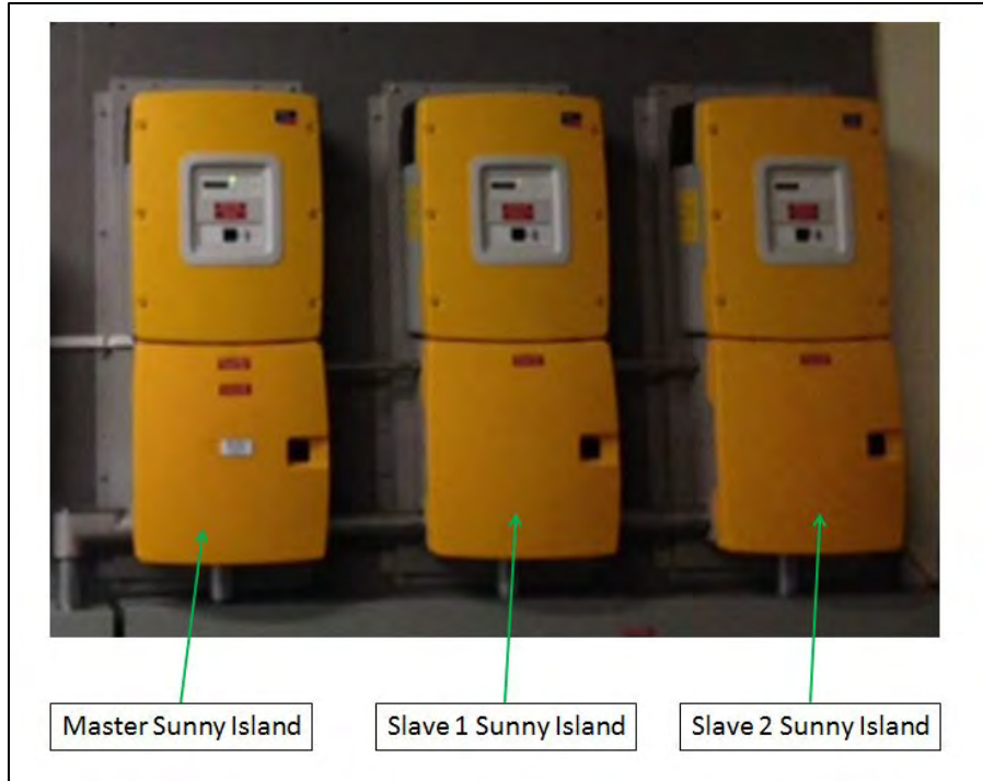
Figure 9. Layout of the 3 Sunny Islands Inverters.
