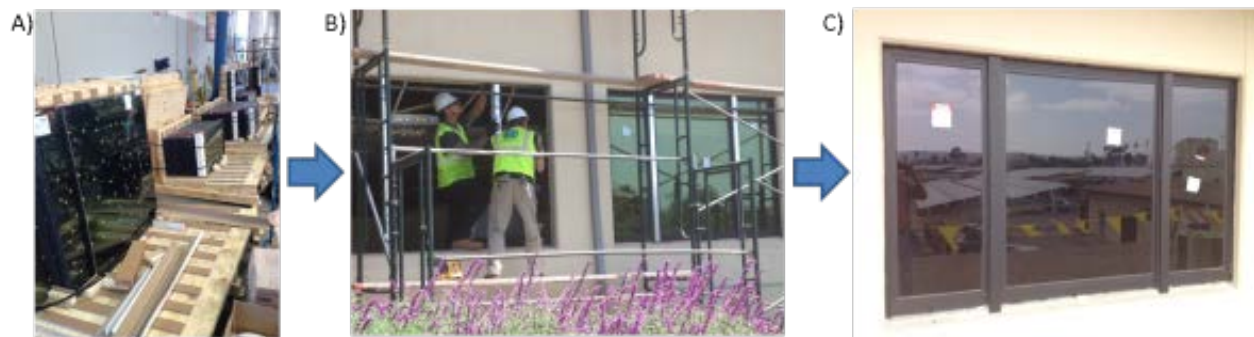
Figure 5. A) View dynamic glass IGUs received at Miramar. B) Construction crew removing old window frames. C) Final installed dynamic windows.
