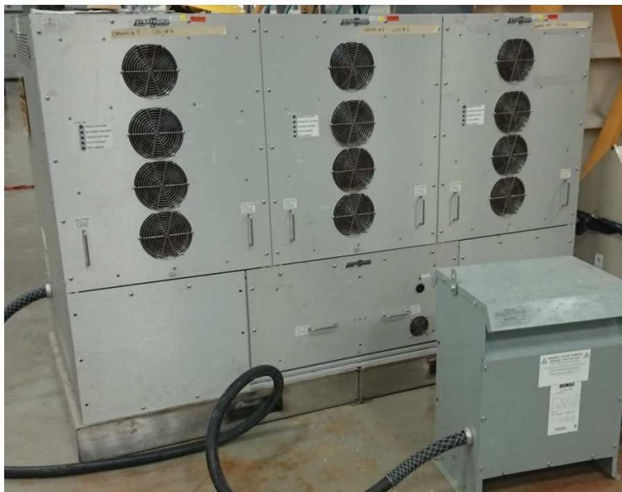
Figure 4-17: Image of 100kW LFP power supply; up to 3 independent channels
