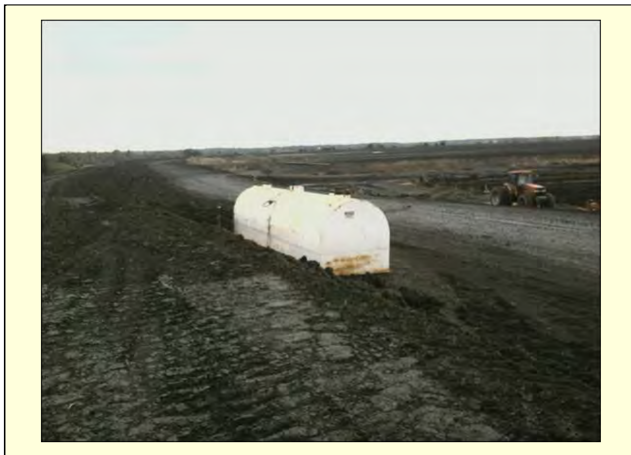
Figure 3-1. Photo of NWS Spoil Area
