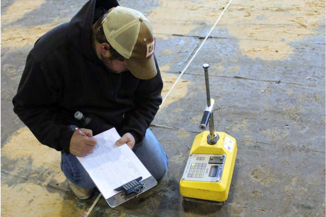
Figure 13. Nuclear moisture-density gauge test.
