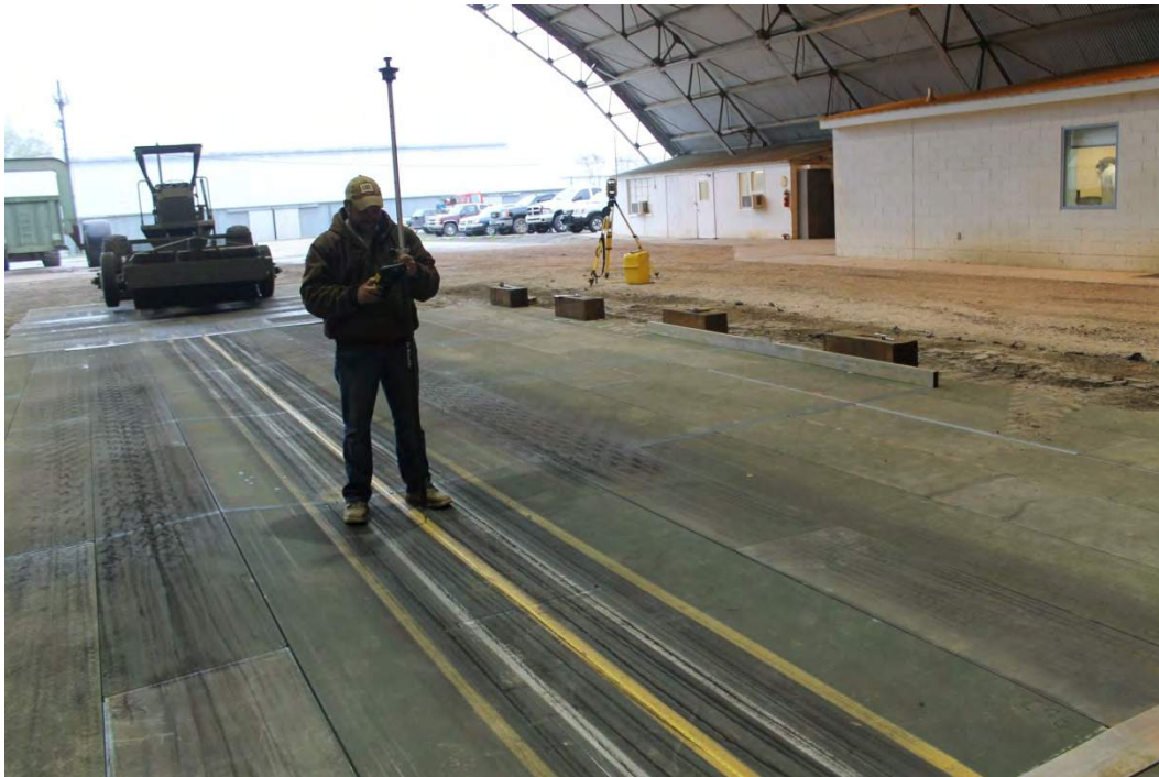
Figure 29. Surveying centerline profile.
