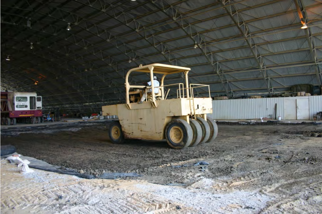
Figure 12. Compacting CH subgrade with pneumatic roller.
