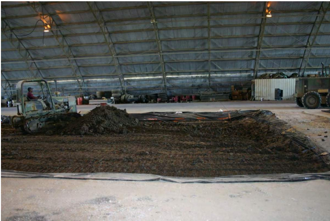
Figure 11. Leveling CH material in test pit prior to compaction.
