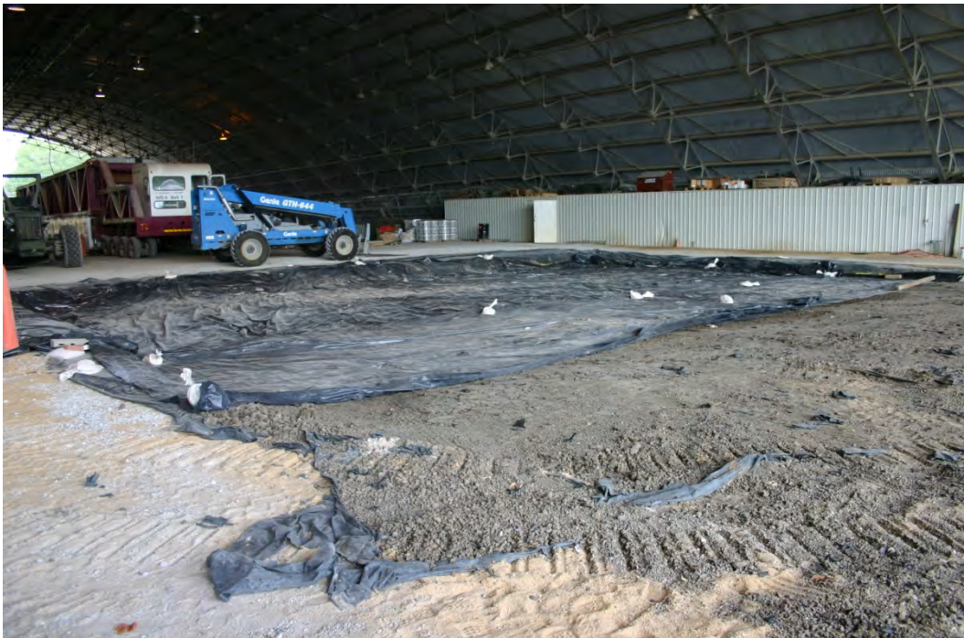
Figure 8. Test pit lined with impervious sheeting.
