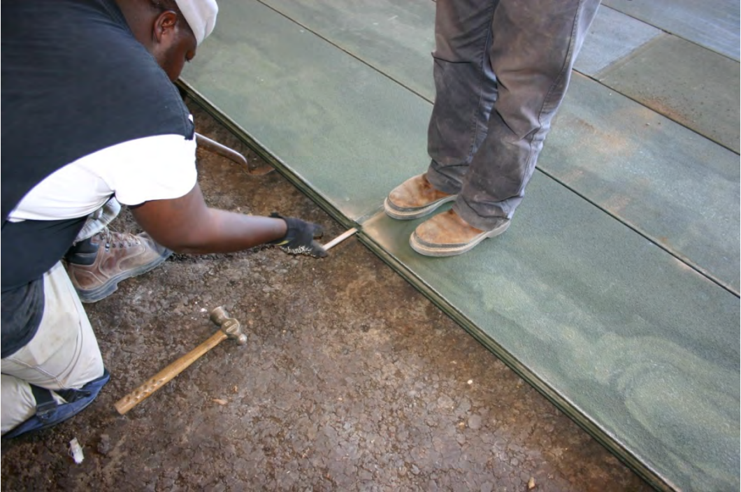
Figure 21. Insertion of aluminum locking bar between adjacent panels.
