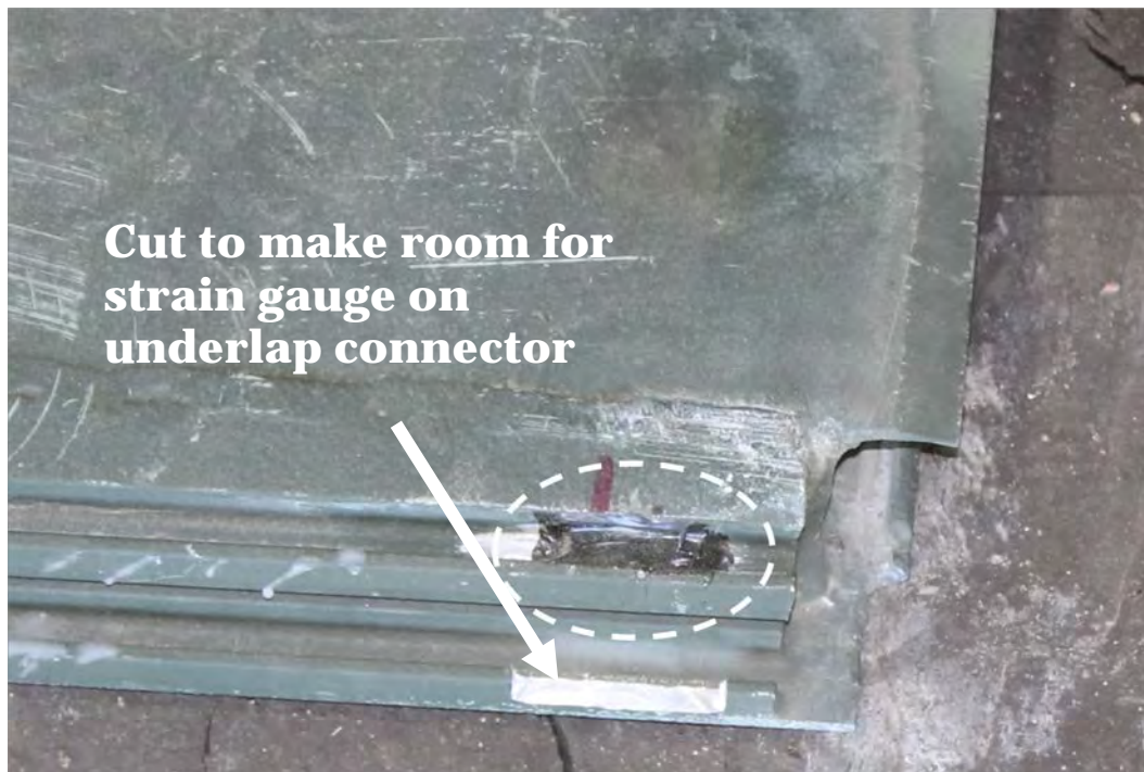
Figure 15. Strain gauge on lower overlap region of AM2 panel end connector.
