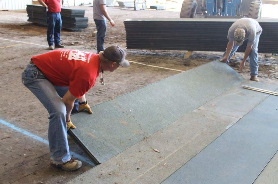
Figure 22. Installation of AM2 panel on the test section subgrade.
