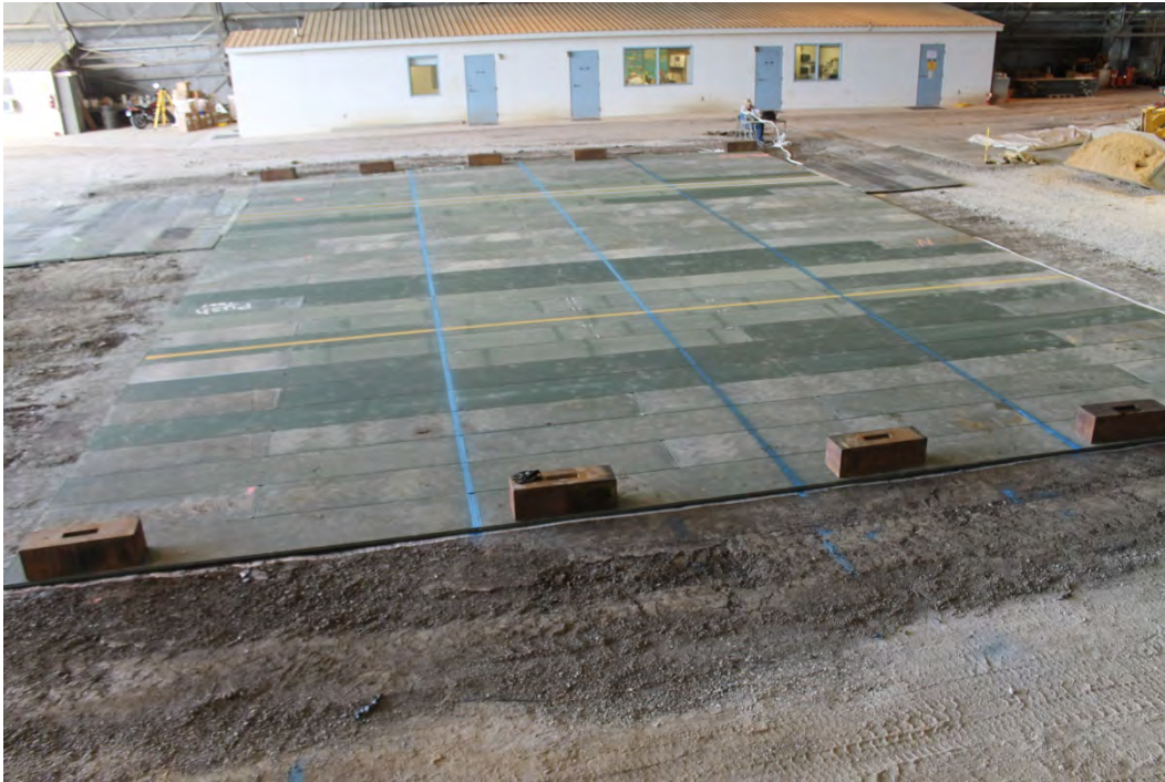
Figure 23. Final assembled test section.
