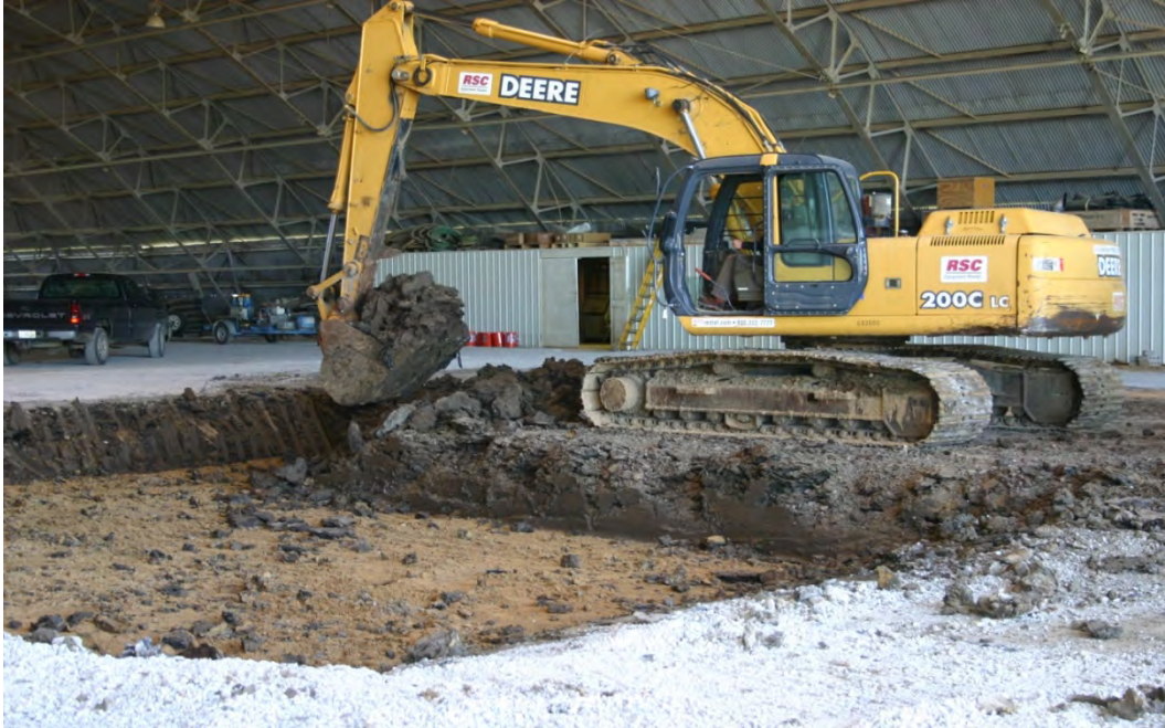
Figure 7. Test section excavation.
