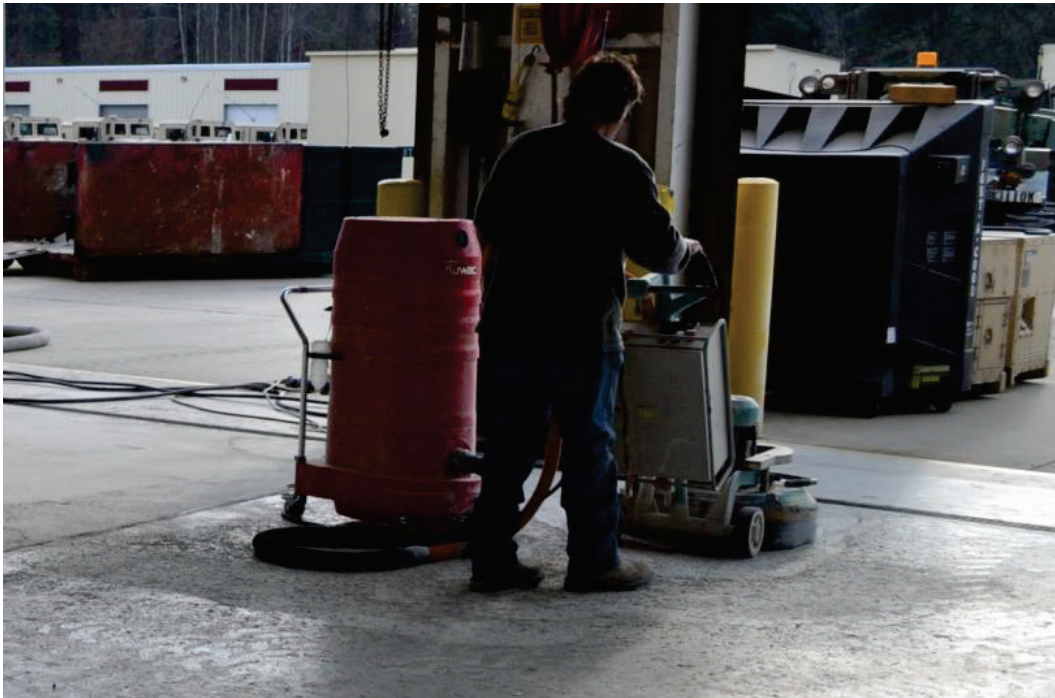
Figure 7. Planetary grinder removing paint.
