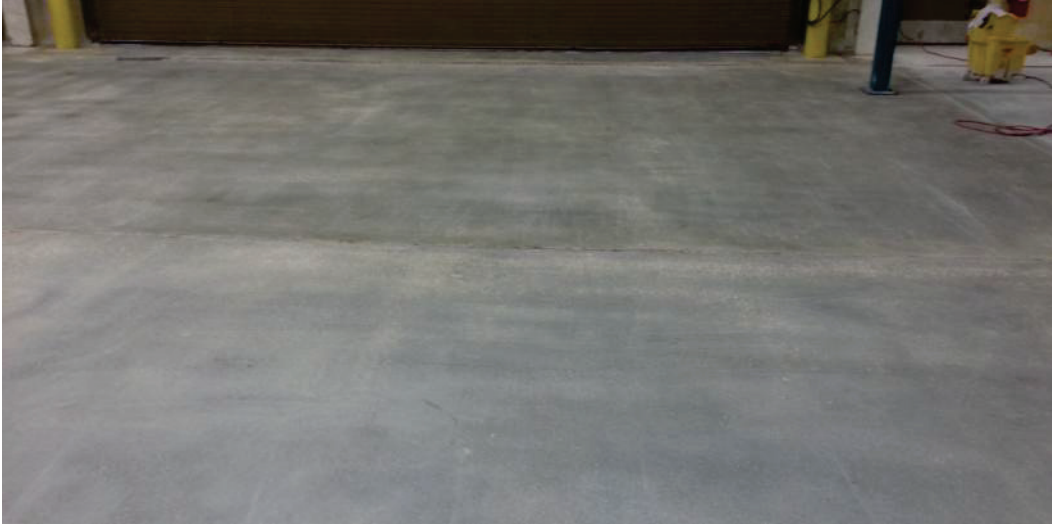
Figure 10. Floor after grinding with 200 grit abrasive.
