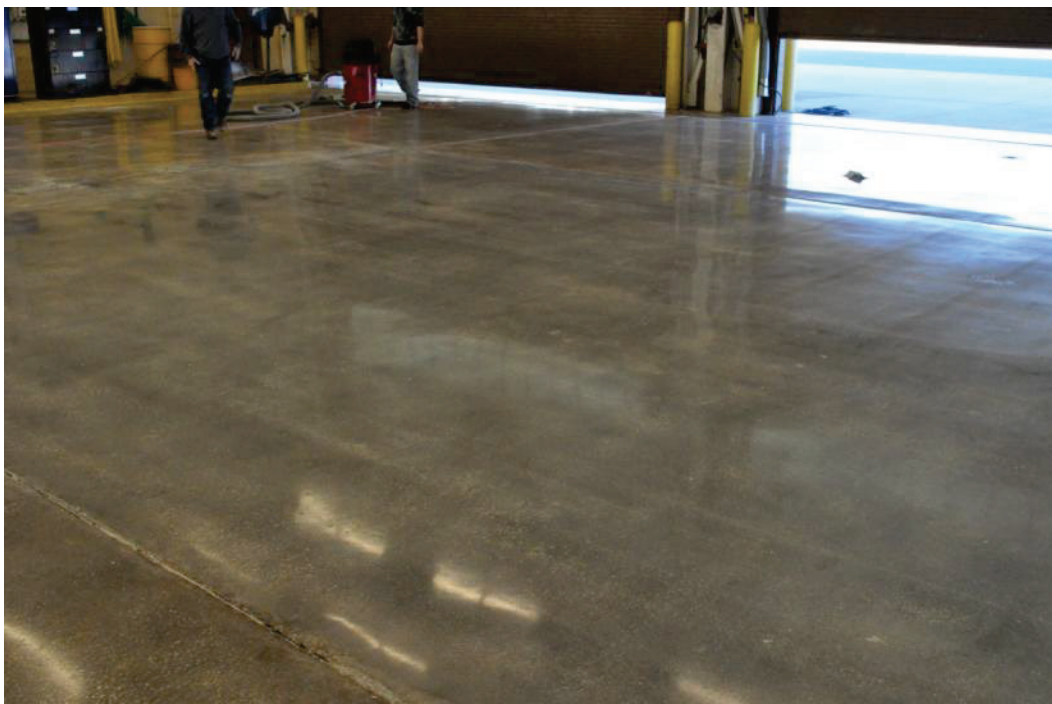
Figure 18. Far-end completed vehicle maintenance bay.
