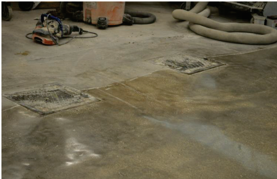
Figure 13. Uneven floor area ground by hand.
