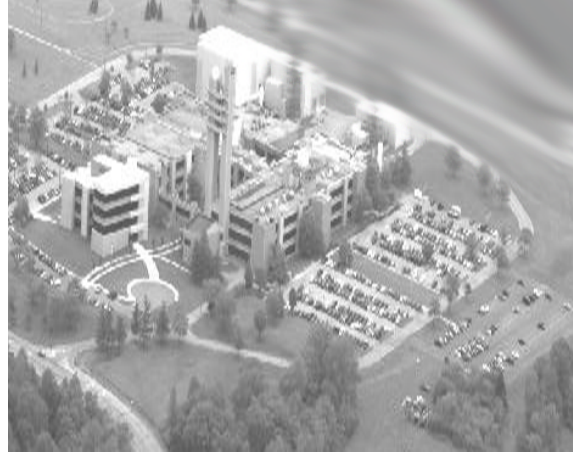
(b) EO Buildings
