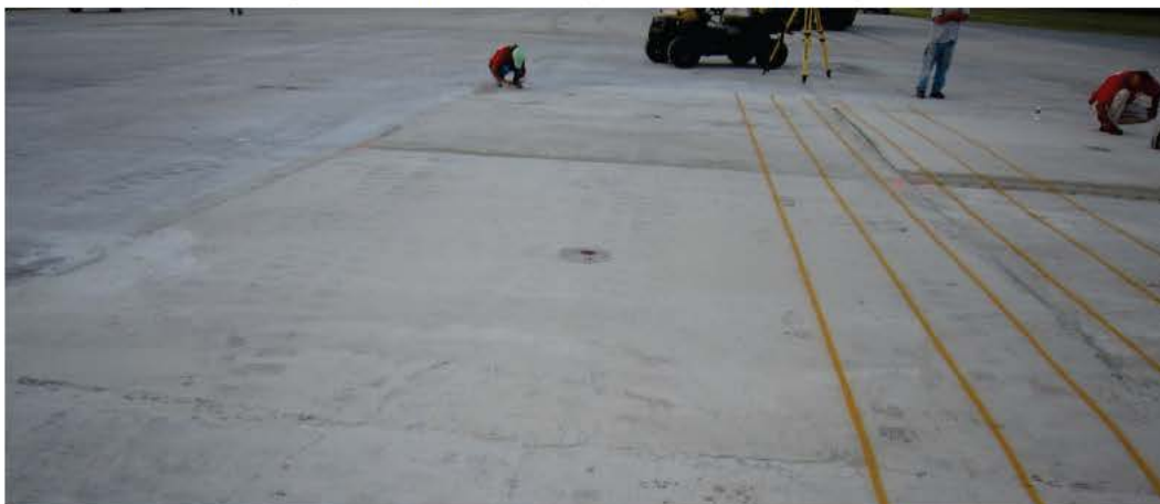
Figure 54. Crater 1, west quadrants, finished repair.
