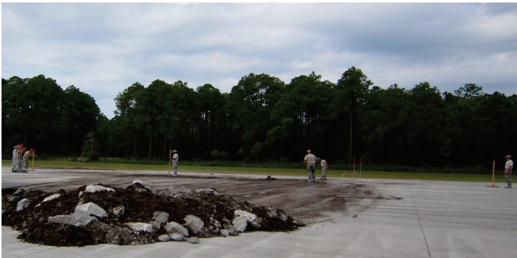
Figure 28. Simulating use of stanchions for marking repair area.
