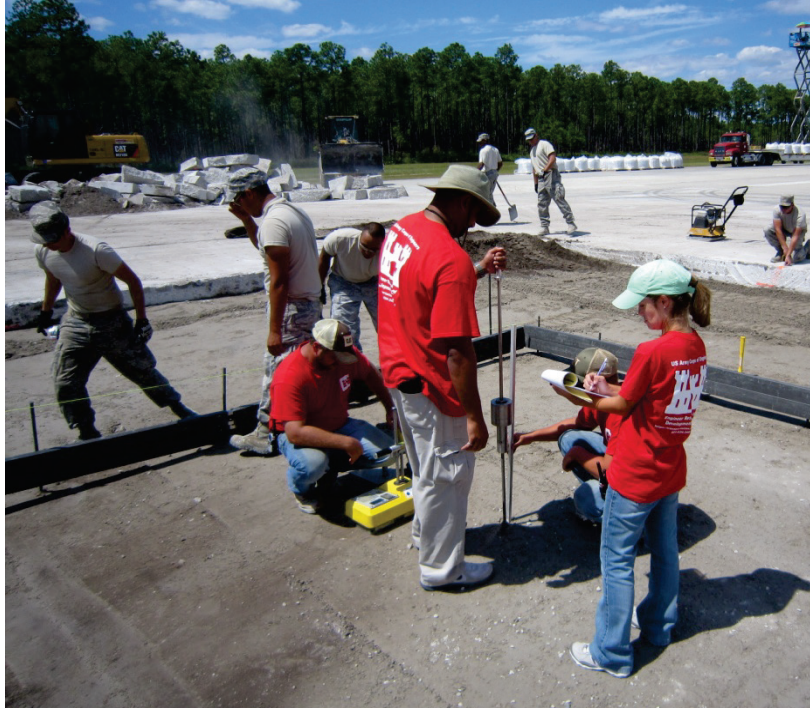
Figure 51. Crushed stone backfill data collection.
