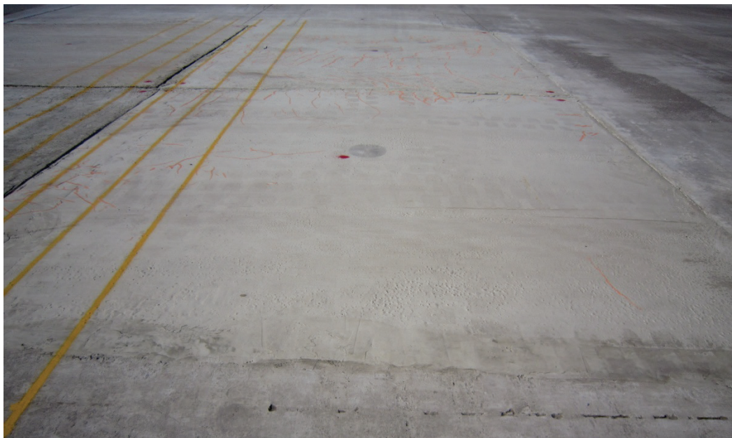
Figure 57. Crater 2, east quadrants, finished repair.
