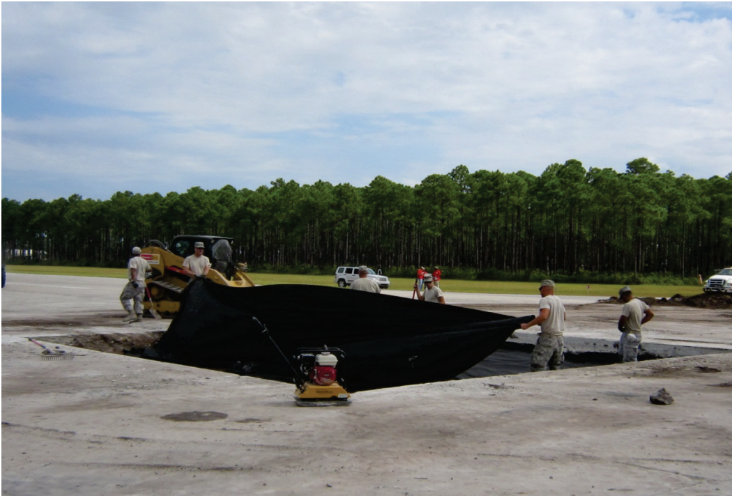
Figure 23. Placement of geotextile.
