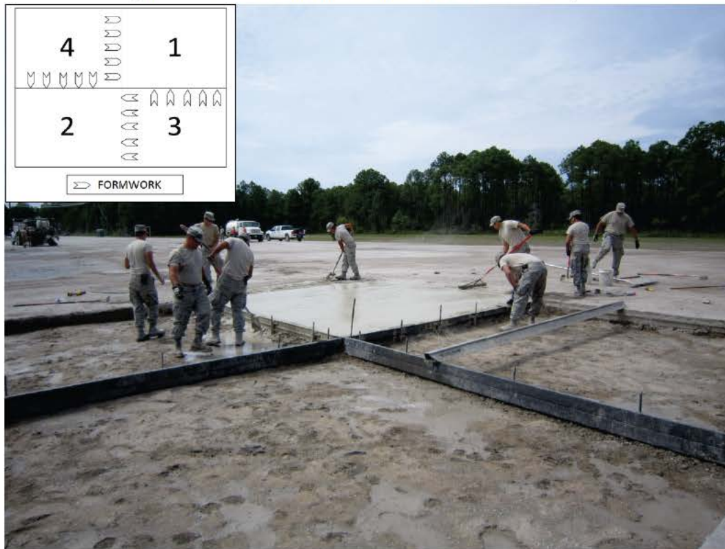
Figure 36. Installed formwork for one of the demo crater repairs.
