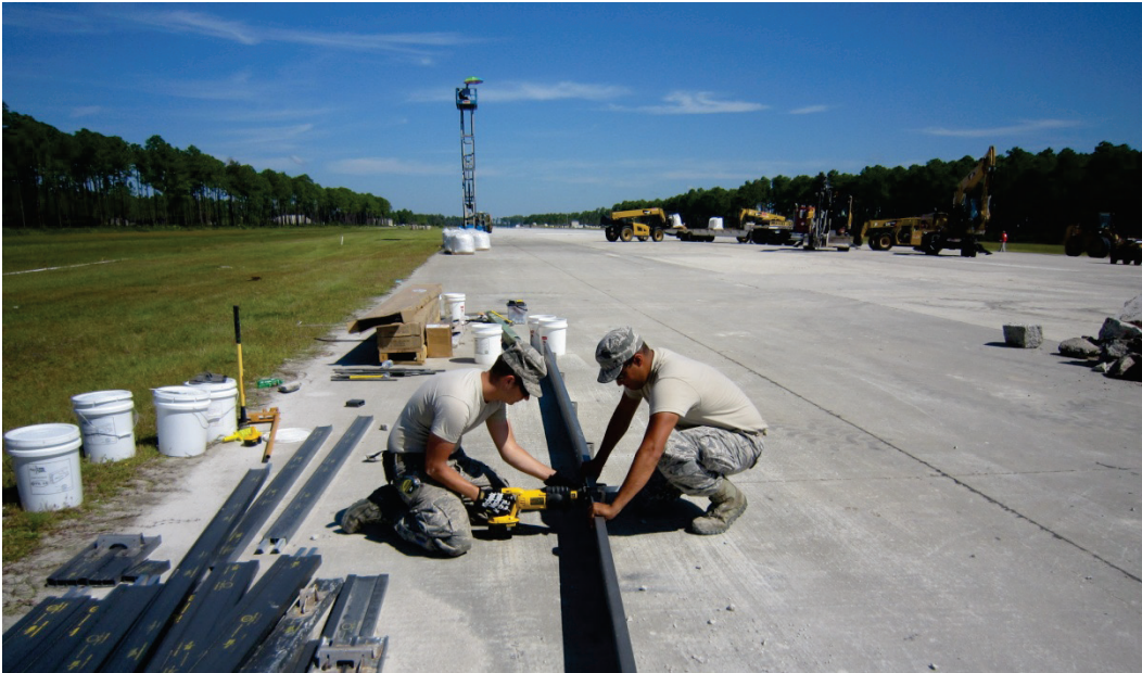
Figure 33. Form team cutting forms to proper length.
