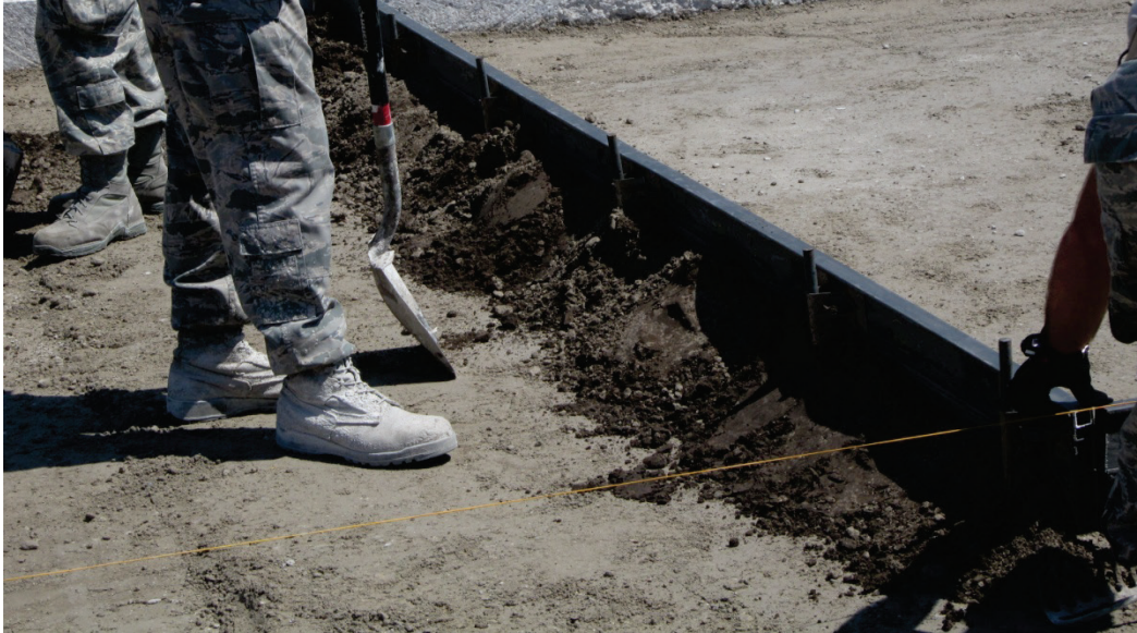
Figure 20. Plastic concrete forms.
