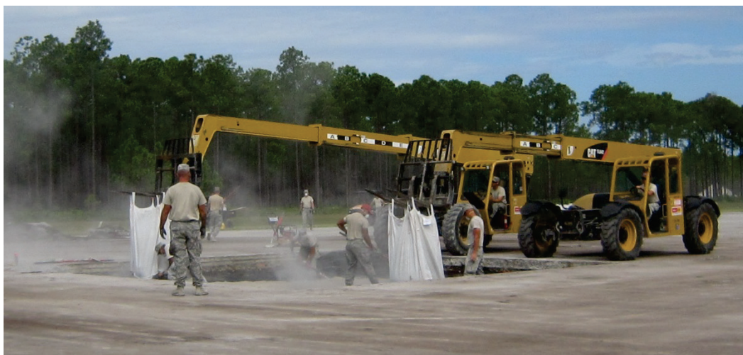
Figure 31. Dry flowable fill placement.
