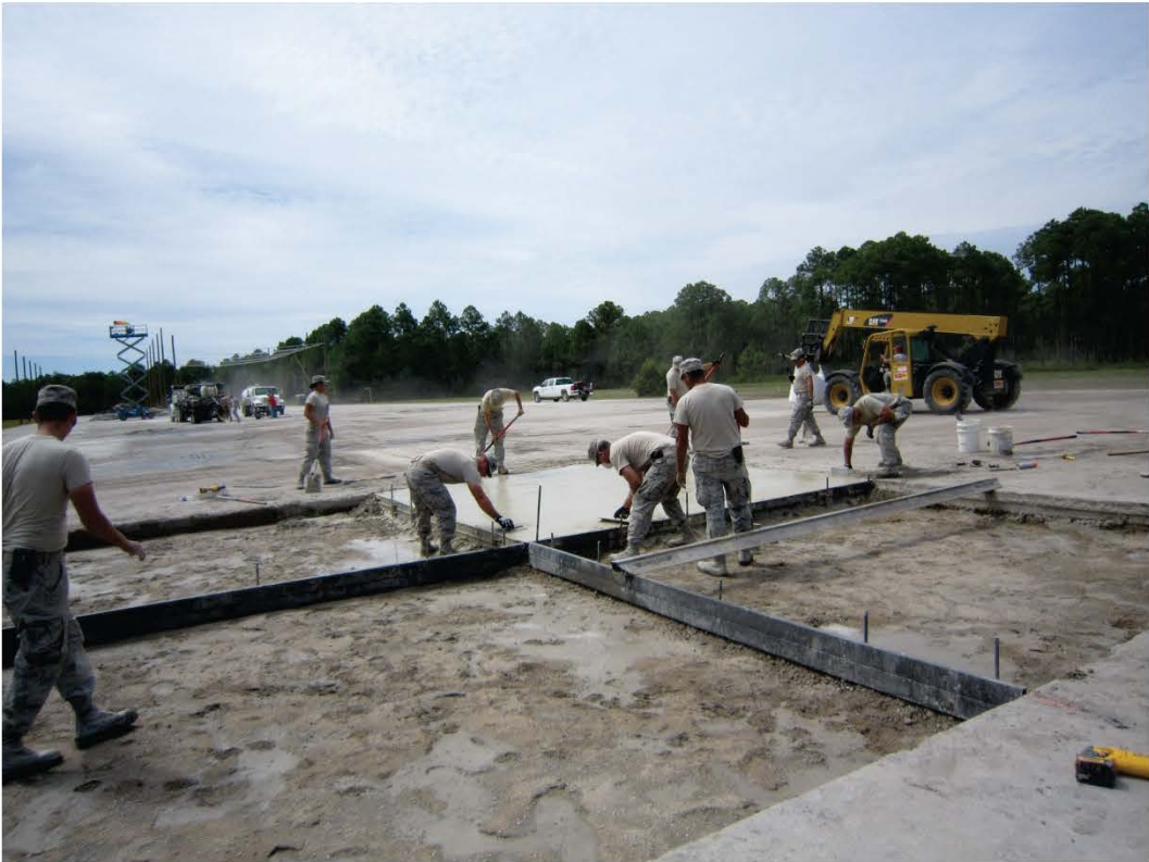
Figure 40. Finishing repair edges with hand tools.
