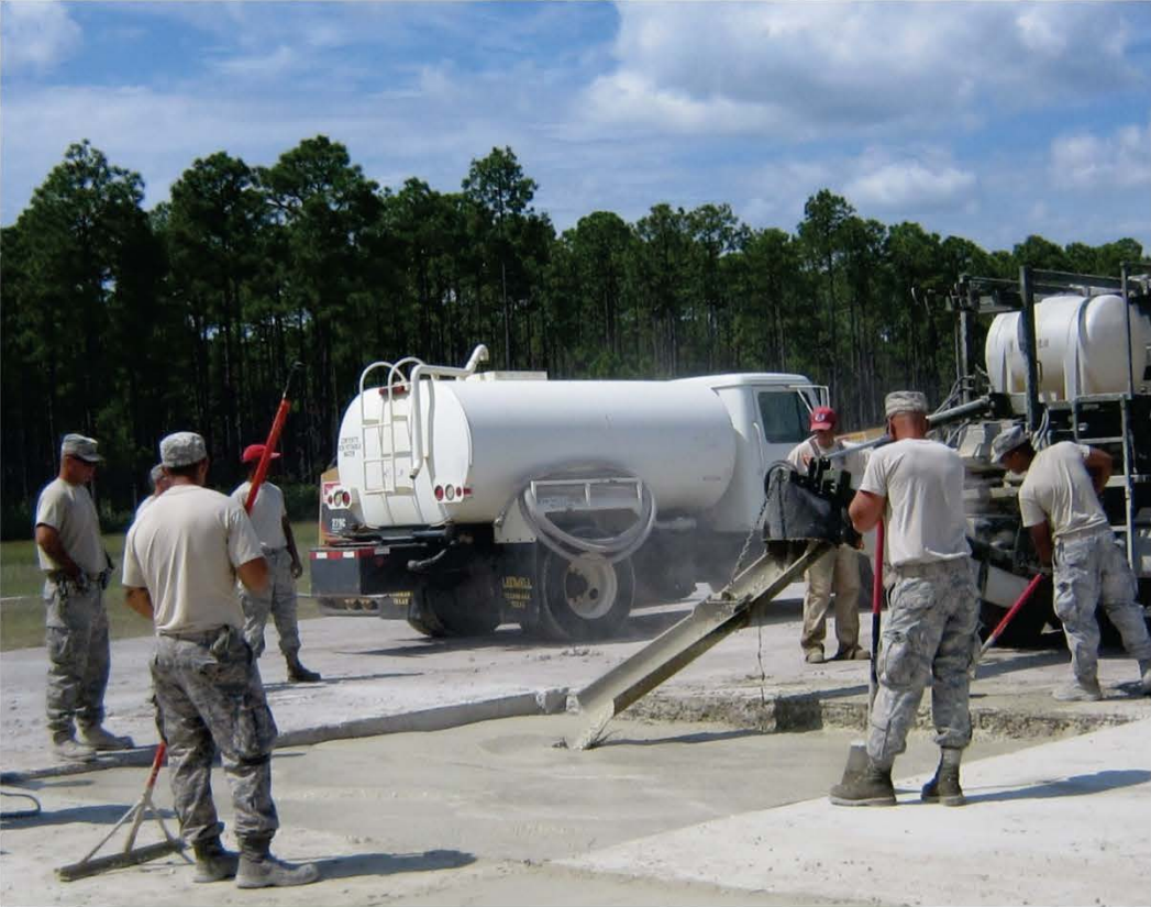
Figure 26. Rapid-setting concrete placed using volumetric mixer.
