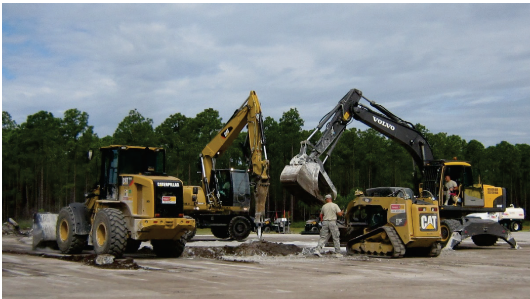
Figure 30. Breaking and excavating PCC and base material simultaneously.
