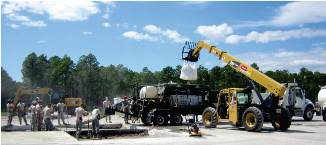
Figure 37. Loading the simplified volumetric mixer during capping.
