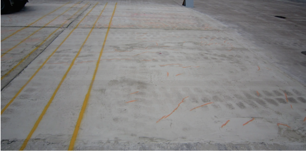
Figure 59. Crater 3, east quadrants, finished repair.
