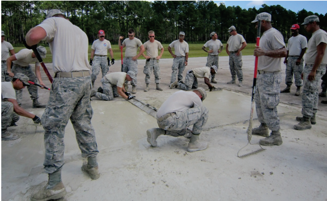
Figure 45. Capping of Training Crater 1.
