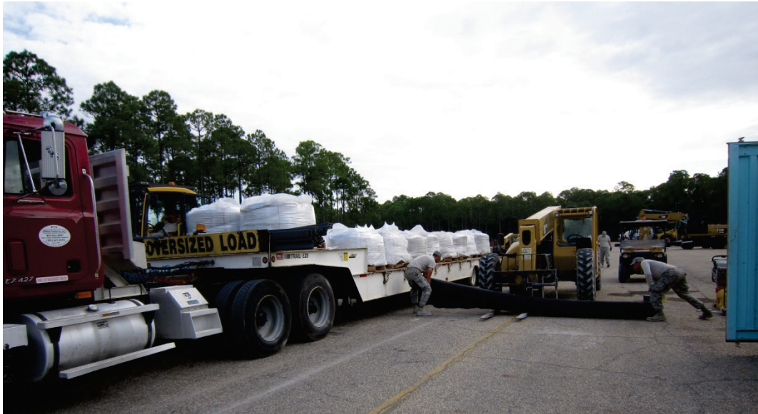
Figure 18. Supersacks and geotextile roll loaded on lowboy trailer.
