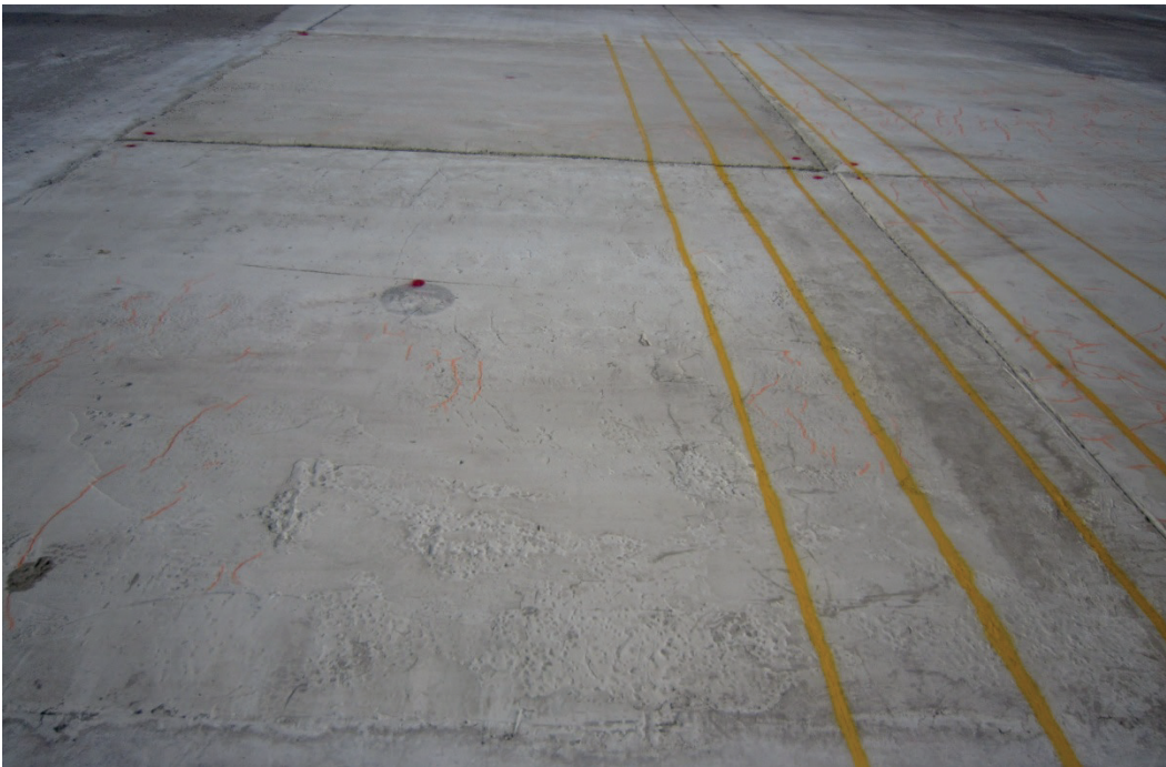
Figure 56. Crater 2, west quadrants, finished repair.
