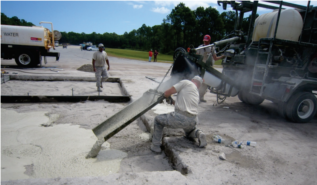
Figure 38. Placement of rapid-setting concrete cap with volumetric mixer.
