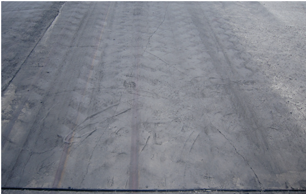
Figure 63. Crater 1, 400 passes, shattered slab in southwest quadrant.
