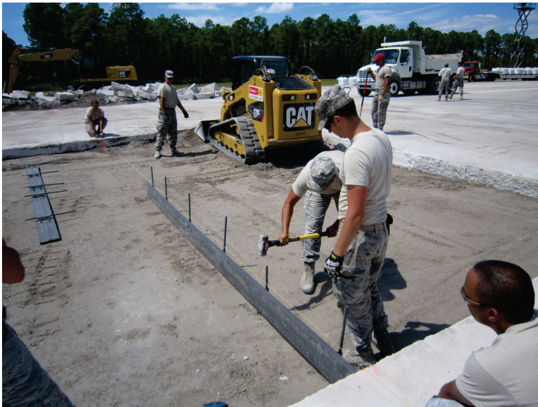
Figure 35. Installation of form pins.
