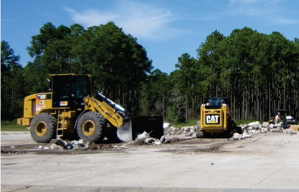
Figure 27. Debris removal team operating CTL and front-end loader.
