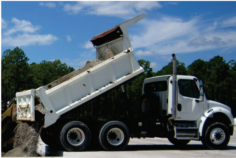
Figure 21. Dump truck unloading crushed stone backfill.
