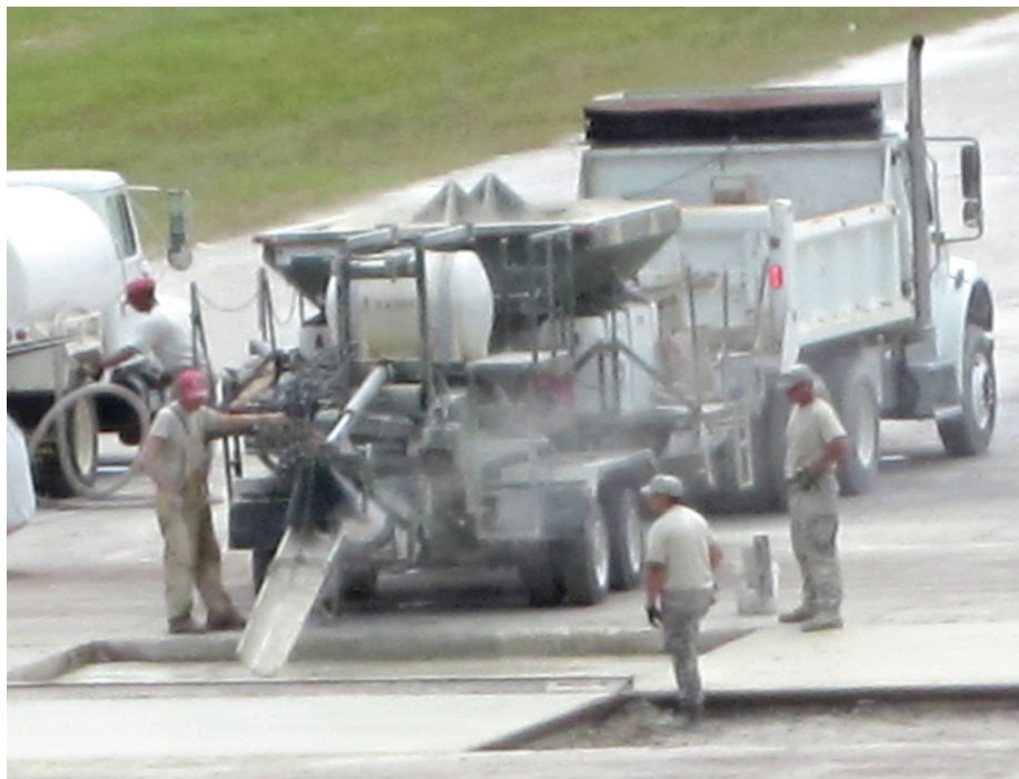
Figure 19. Simplified volumetric mixer towed by a dump truck.
