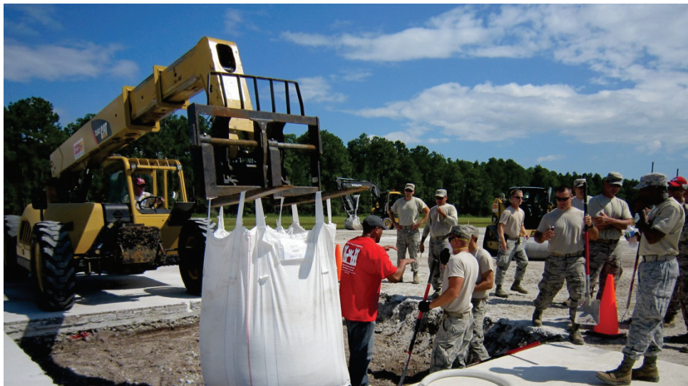
Figure 42. Backfill training with ERDC personnel.
