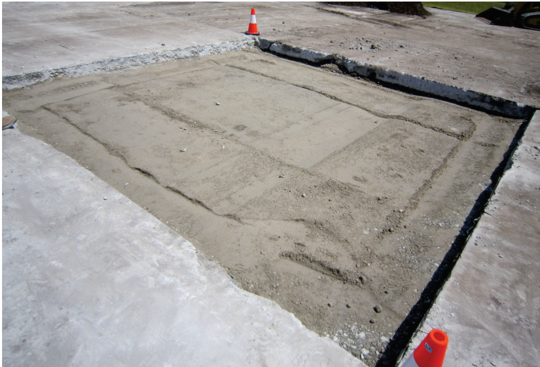
Figure 44. Completed crushed stone backfill - Training Crater 1.
