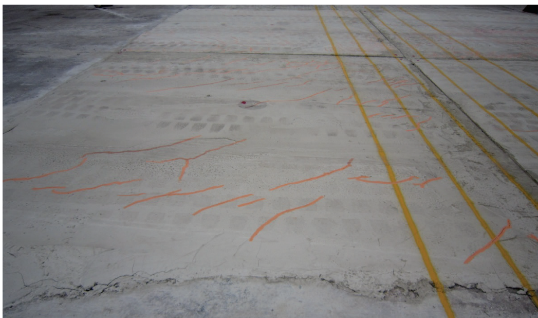
Figure 58. Crater 3, west quadrants, finished repair.
