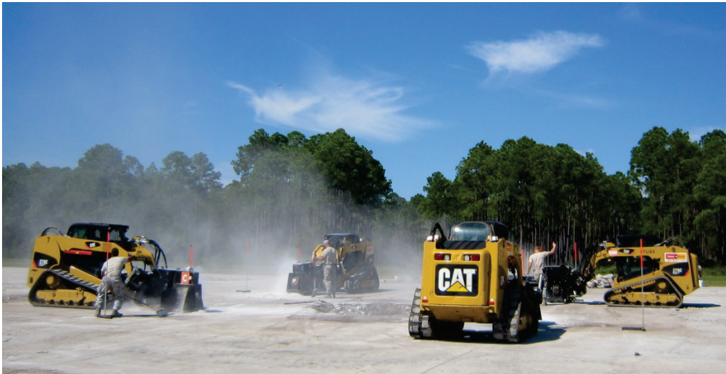
Figure 29. Saw cutting with four CTLs equipped with wheel saws and two spotters; Crater chief shown in center.
