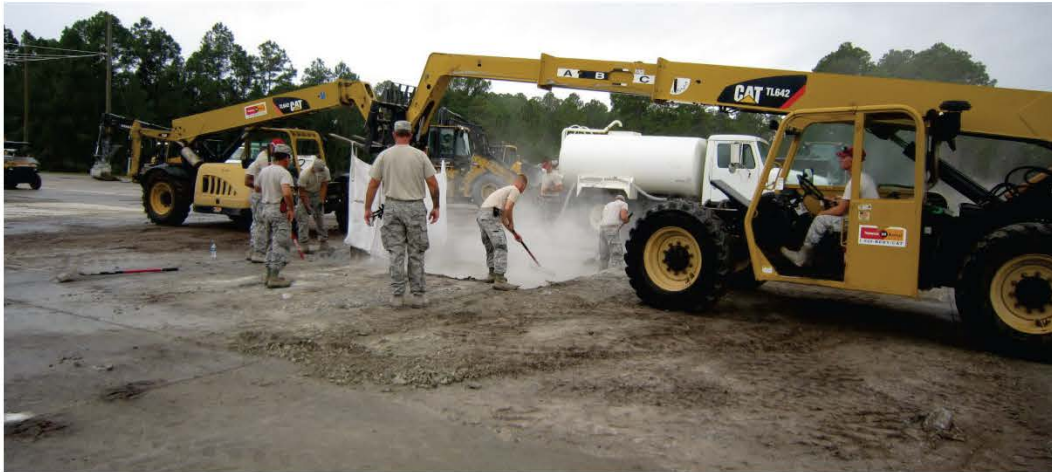
Figure 46. Flowable fill backfill construction - Training Crater 2.
