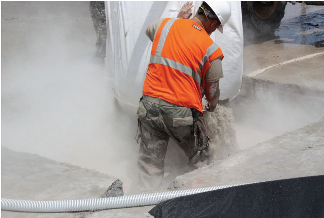
Figure 25. Dumping flowable fill packaged in super sacks prior to adding water, according to the dry method.
