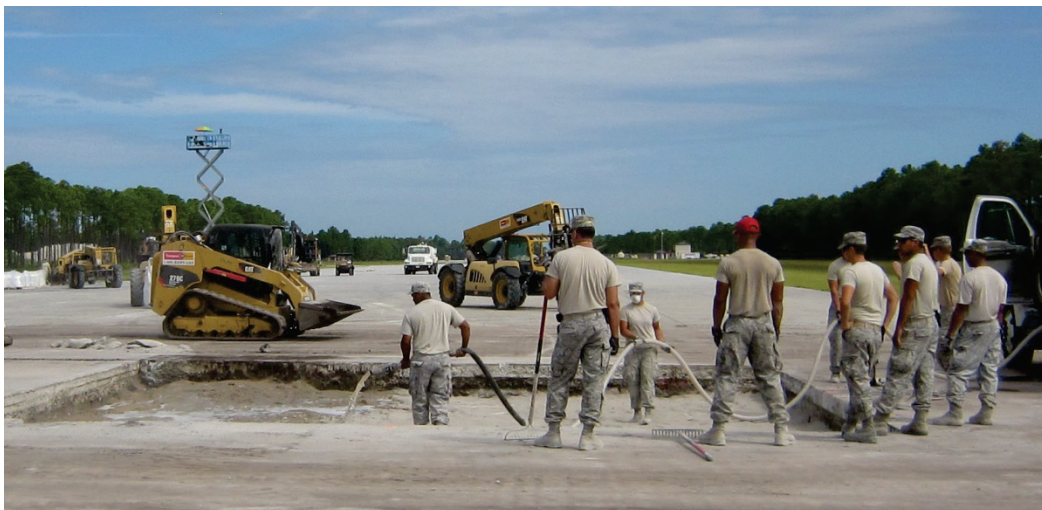
Figure 32. Water addition to flowable fill backfill.
