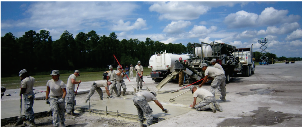
Figure 39. Finishing using the magnesium screed bar.
