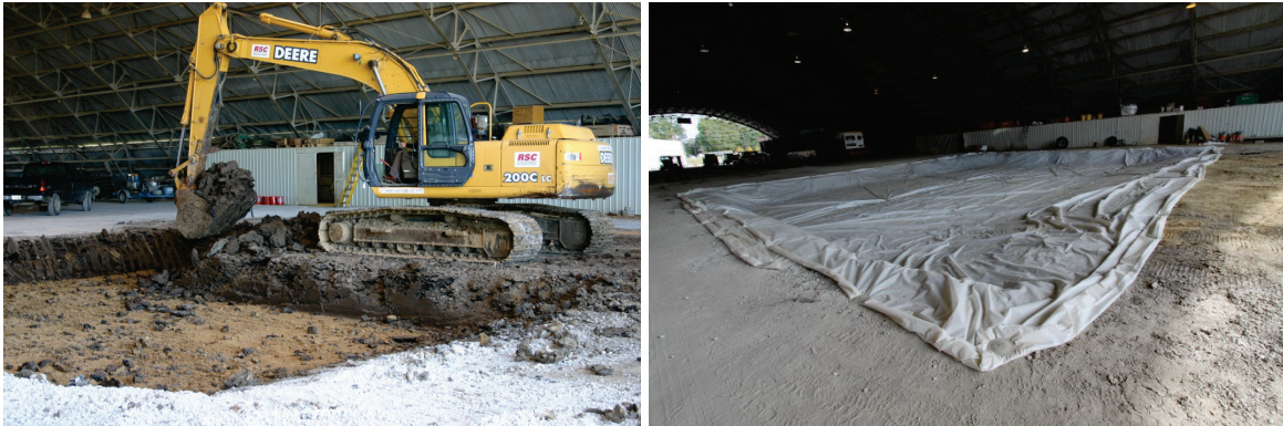
Figure 10. Test section excavation (left) lined with impervious sheeting (right).
