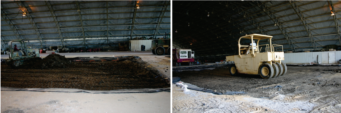
Figure 12. Leveling (left) and compacting (right) CH.
