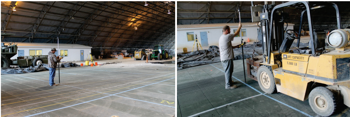
Figure 24. Surveying an unloaded (left) and a loaded (right) cross section.
