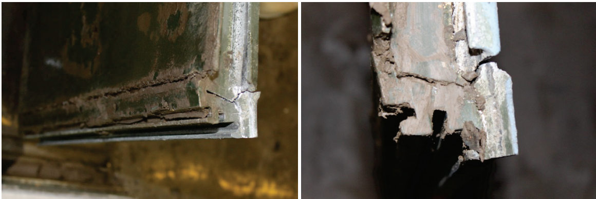
Figure 30. Detached end connector at I-51 (left) and I-69 (right).
