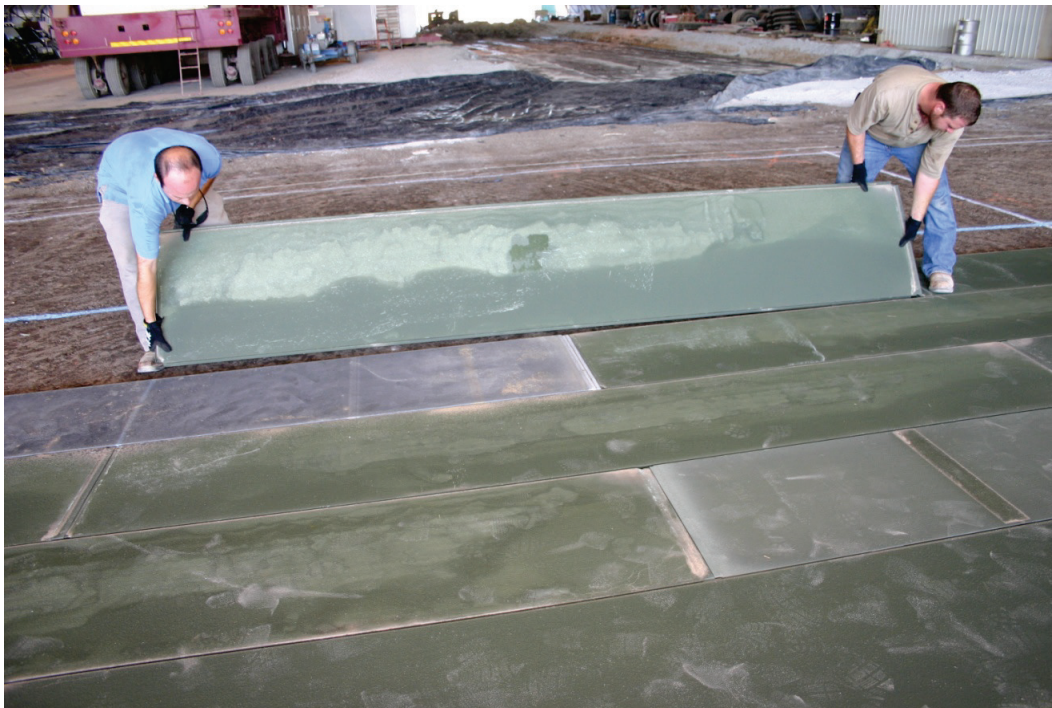
Figure 16. Installation of AM2 panels on the test section subgrade.
