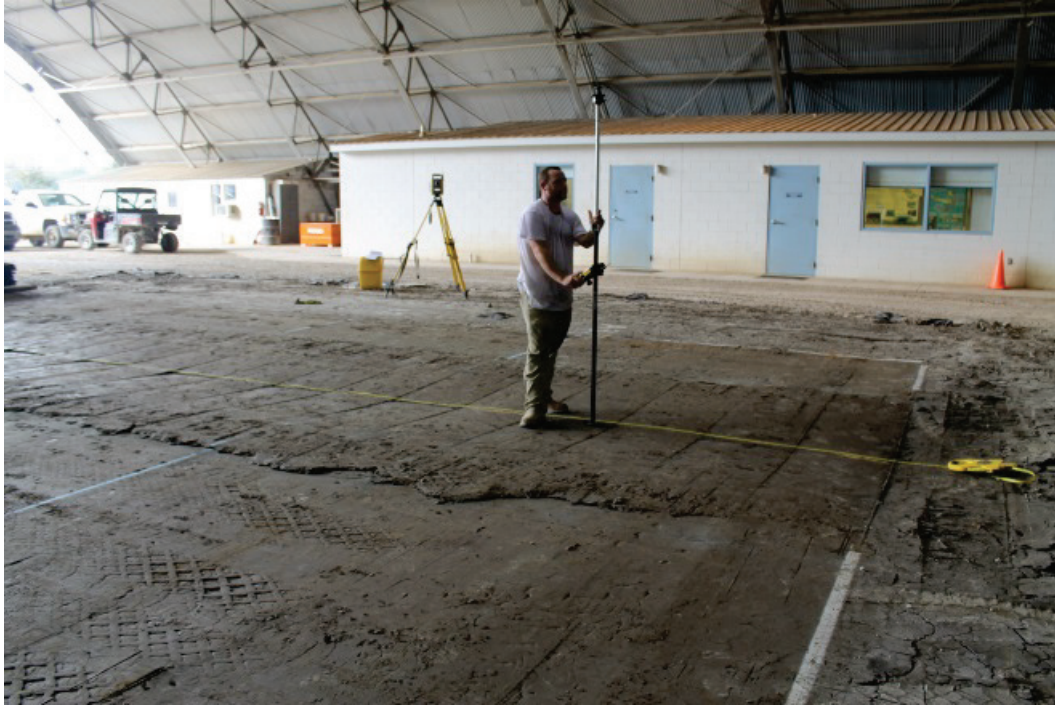
Figure 23. Surveying the subgrade after completing trafficking.
