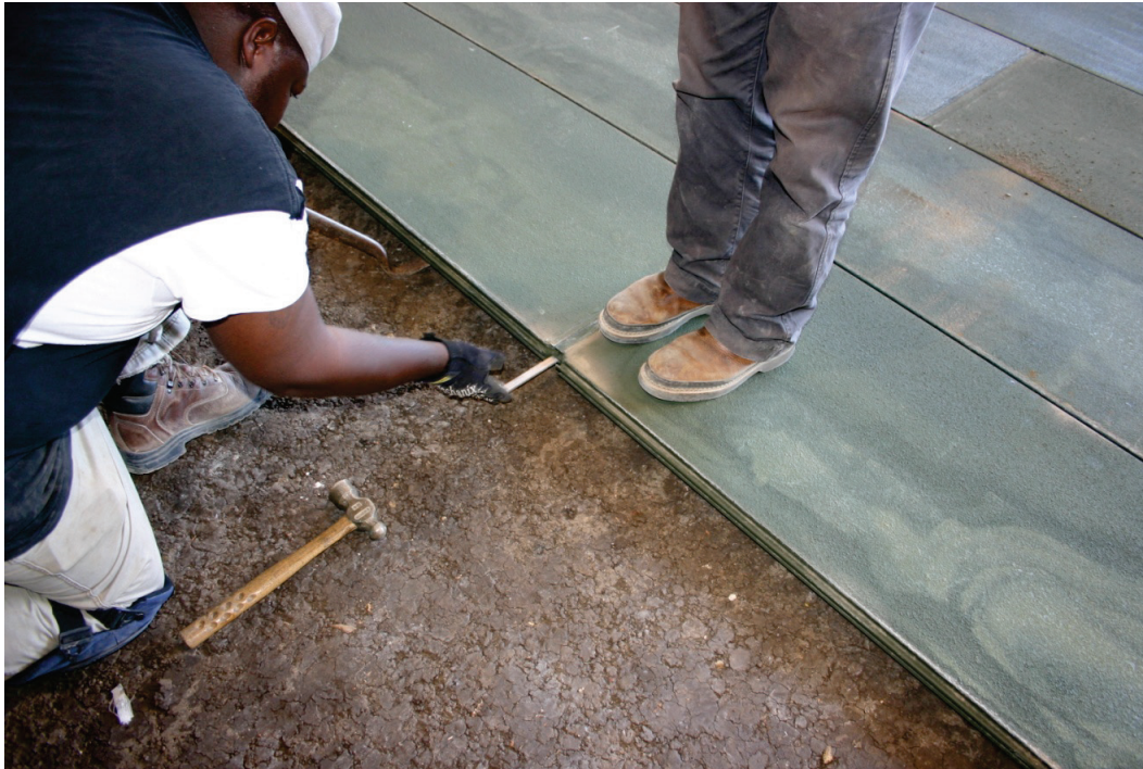
Figure 15. Insertion of aluminum locking bar between adjacent panels.
