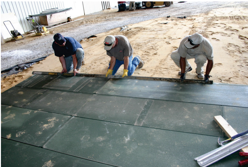
Figure 18. Typical installation of male keylock.
