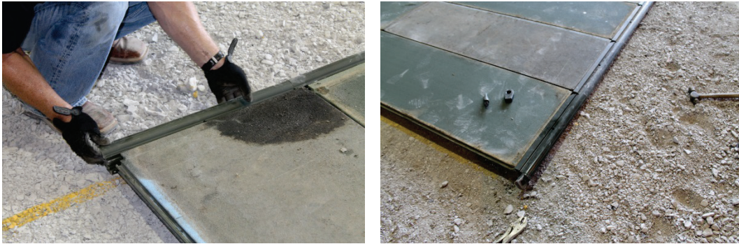
Figure 17. Typical installation of towing tubes to the edges of the test section.
