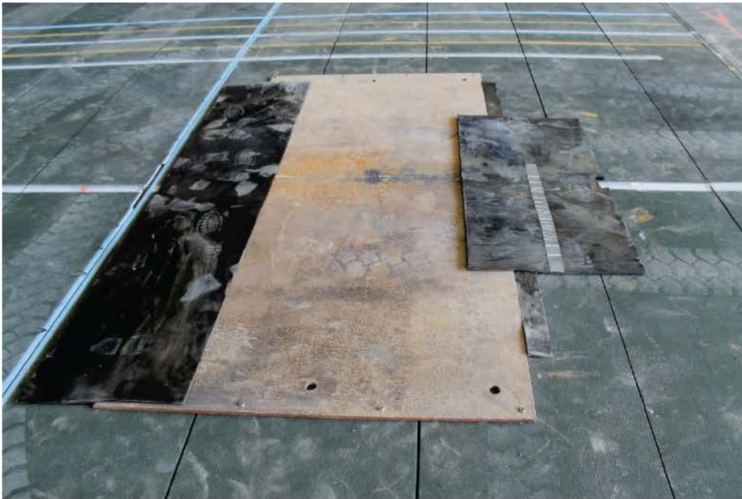
Figure 34. Metal plate placed above I-17 and I-18.
