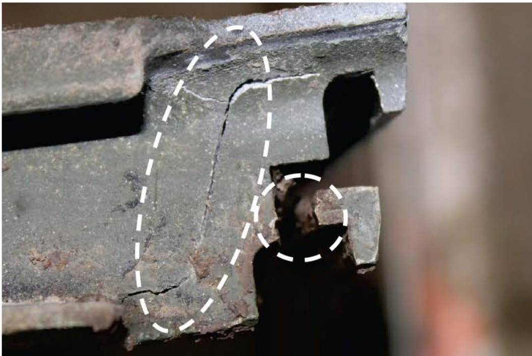
Figure 32. Crack at weld and broken lower overlap rail at I-42.
