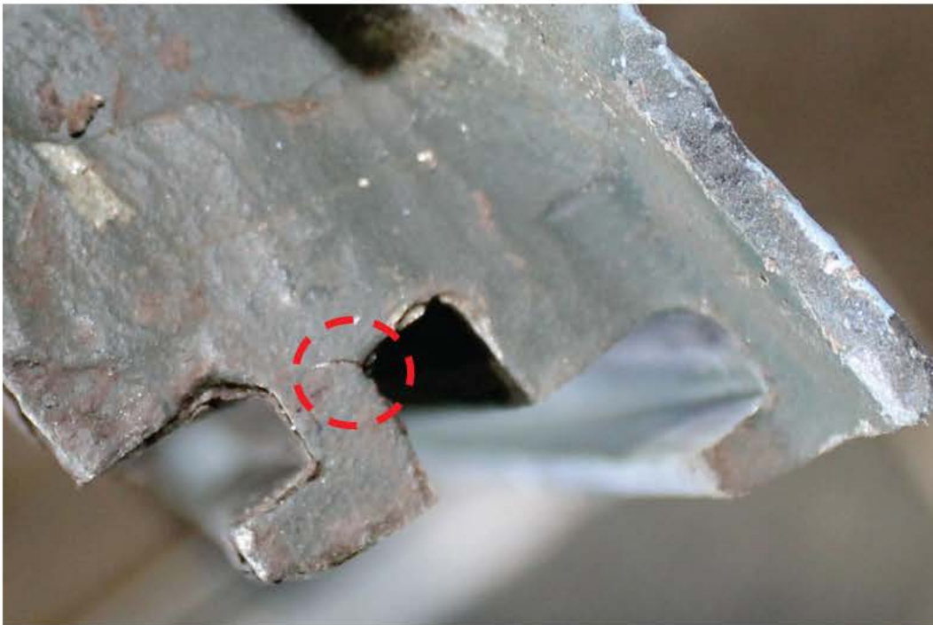
Figure 3. Crack initiation at lower overlap rail.
