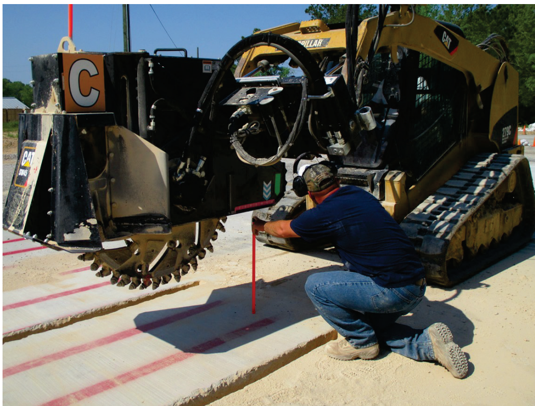
Figure 31. Spotter lining up Caterpillar SW45 saw to obtain 4- to 8-in-long overcut.
