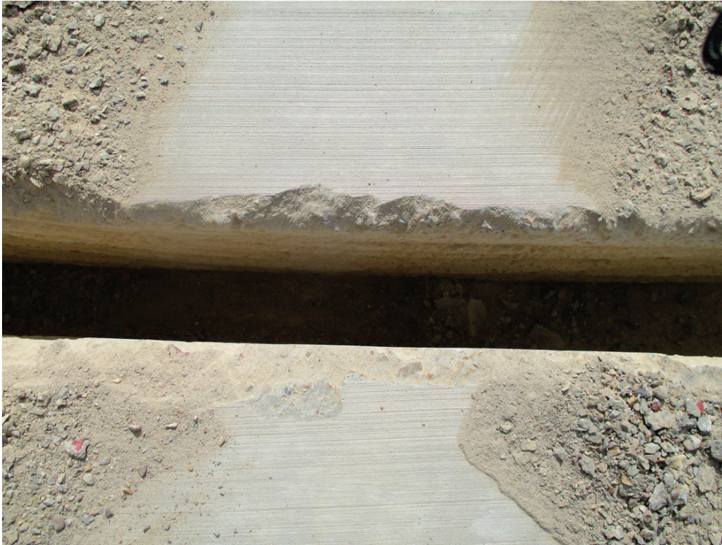
Figure 52. Spalling of chert PCC with Kenn SM04 teeth on Vermeer CC1531.
