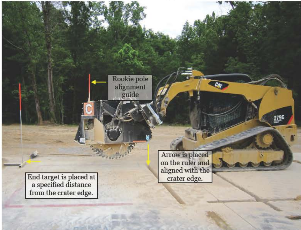
Figure 12. Wheel saw target setup (Edwards et al. 2015).
