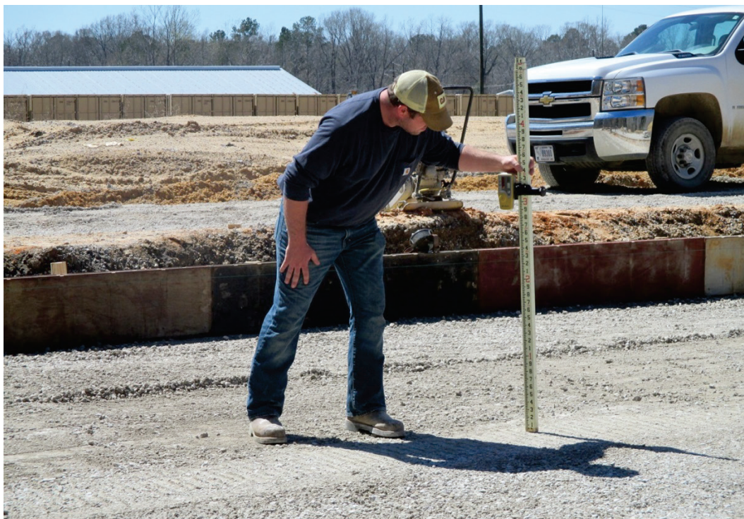
Figure 4. Surveying base layer.
