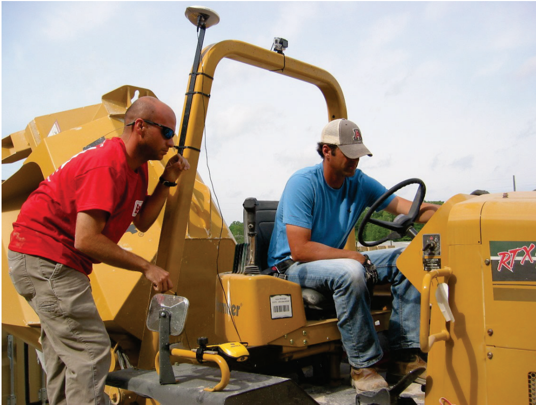
Figure 29. Checking electronics installed on saw before obstacle course.
