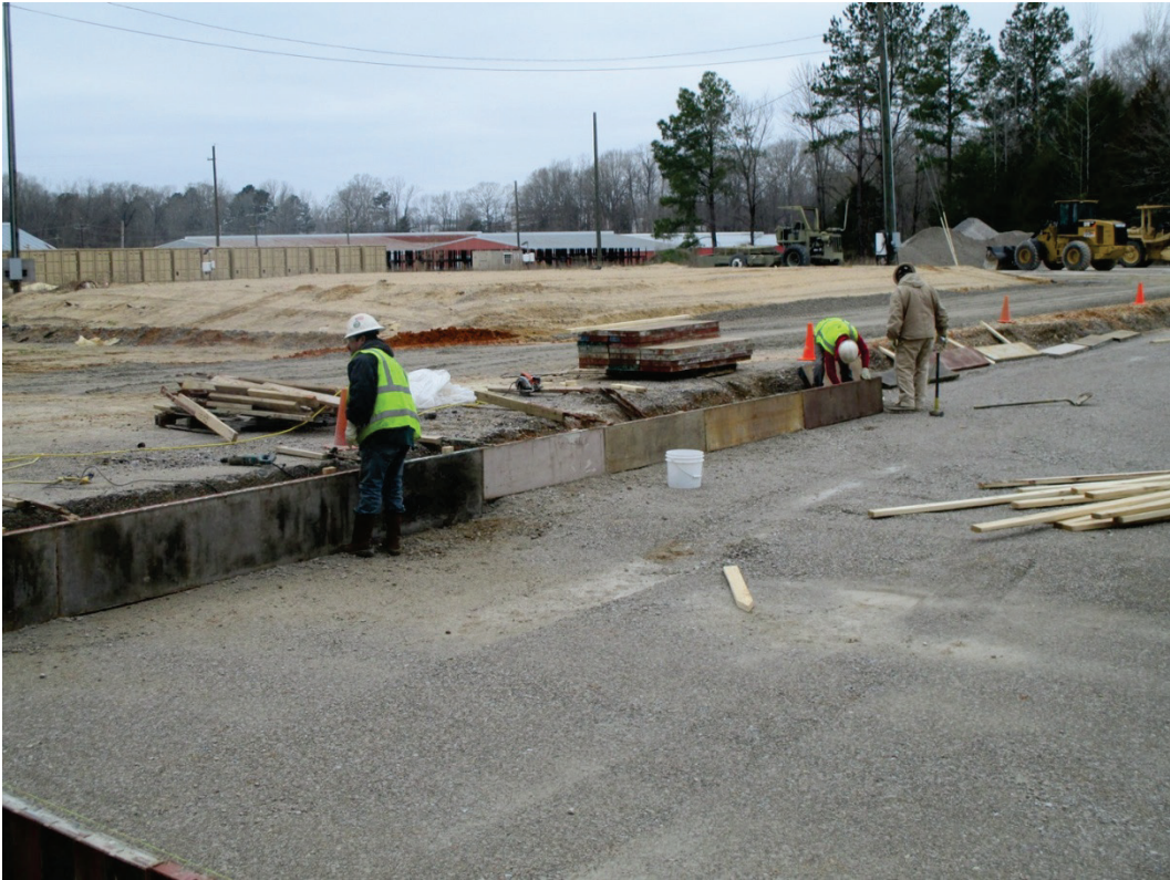
Figure 6. Installing steel forms around perimeter of test section.
