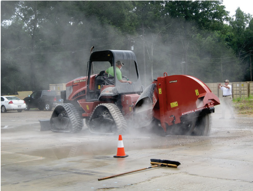
Figure 20. Ditch Witch RT120 Quad with H1140 rock saw.
