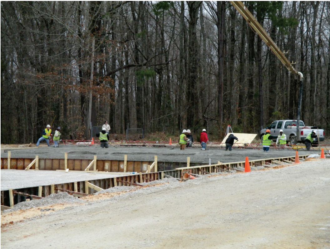
Figure 7. Placing PCC via pump truck.
