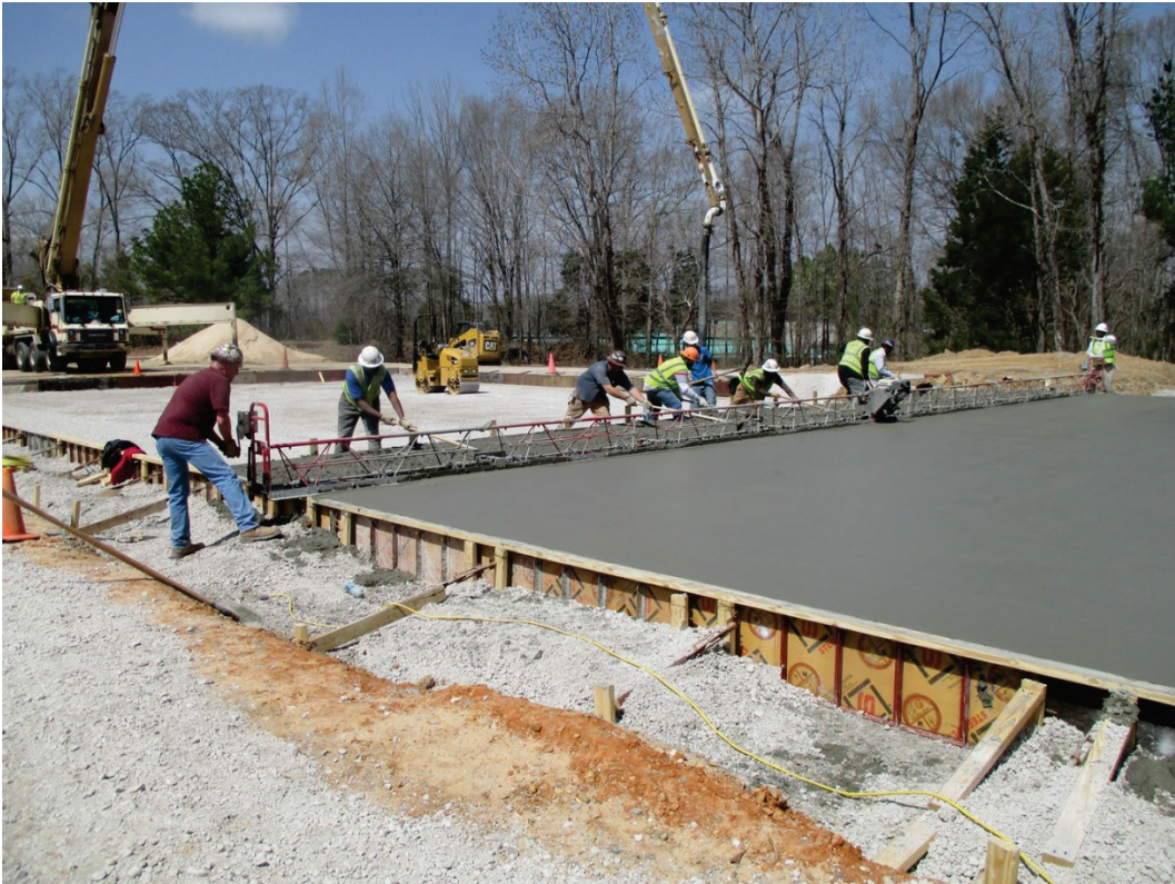
Figure 8. Screeding PCC by using vibratory truss screed.
