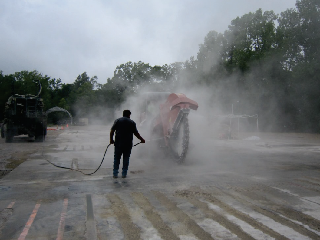
Figure 48. Misting water on Ditch Witch H1140 saw during saw cutting.
