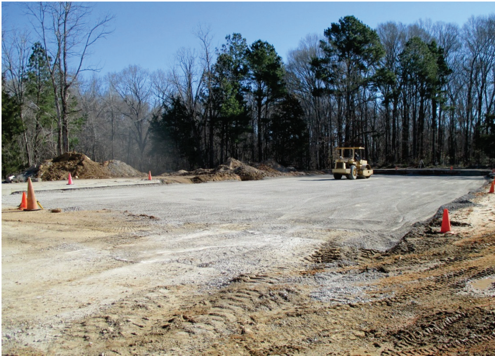
Figure 2. Compacting crushed limestone base material.
