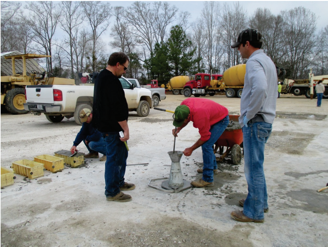
Figure 9. Casting PCC beams and measuring PCC slump.
