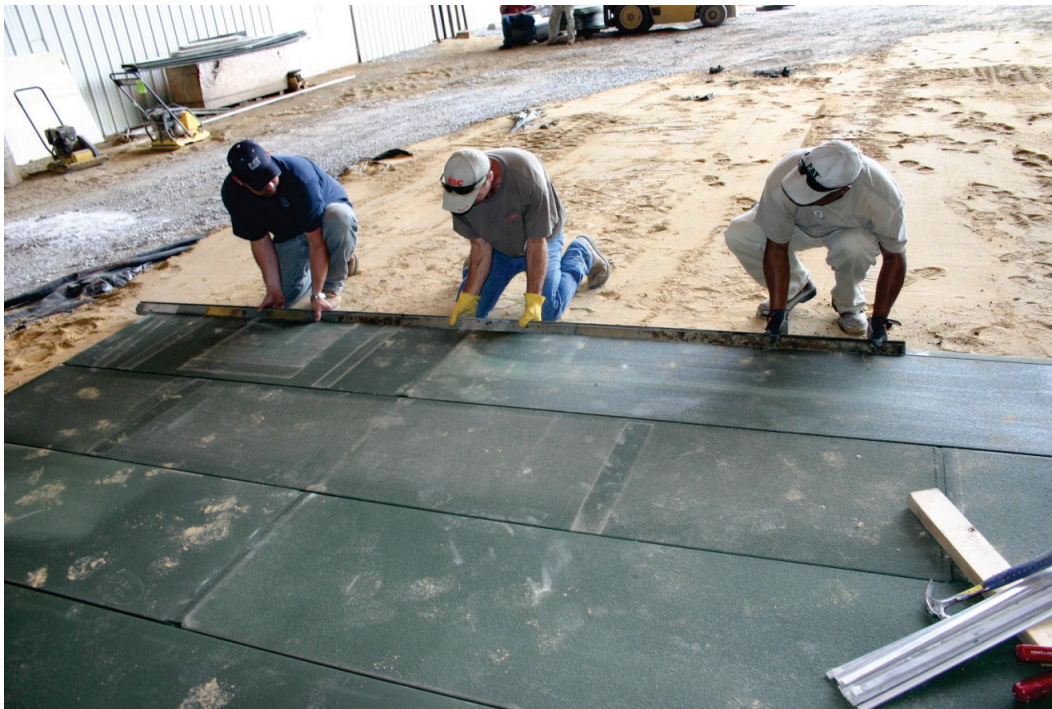
Figure 28. Typical Installation of male keylock.
