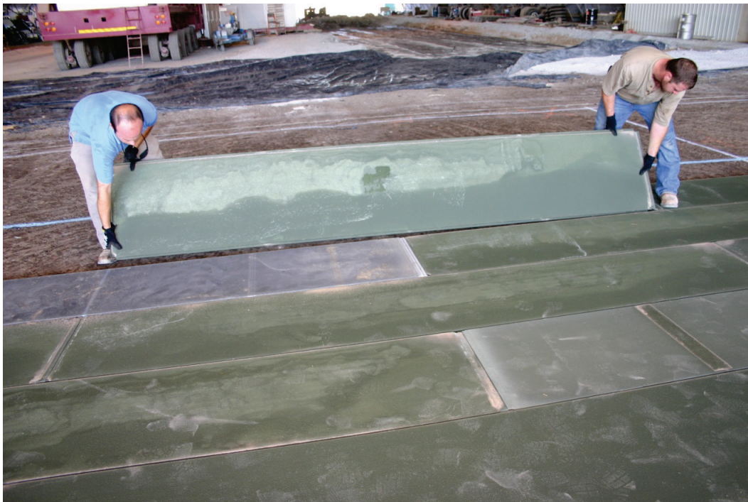
Figure 26. Installation of AM2 panels on the test section subgrade.
