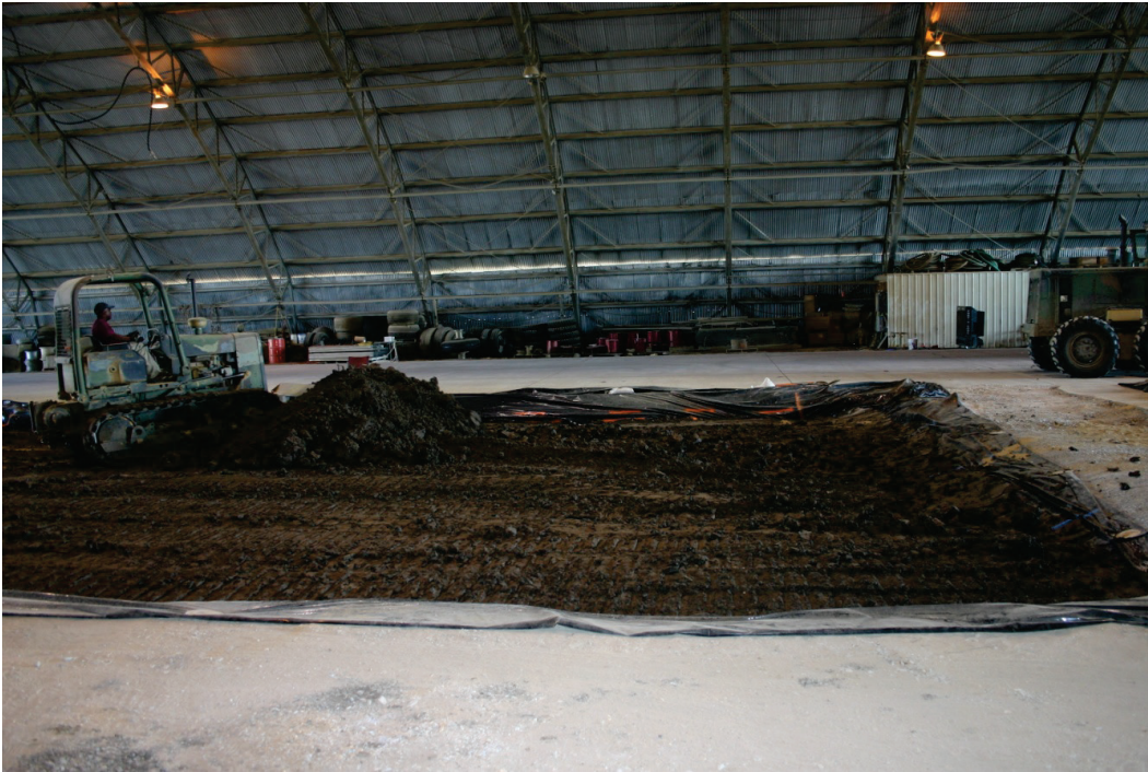
Figure 14. Leveling CH material in test pit prior to compaction.
