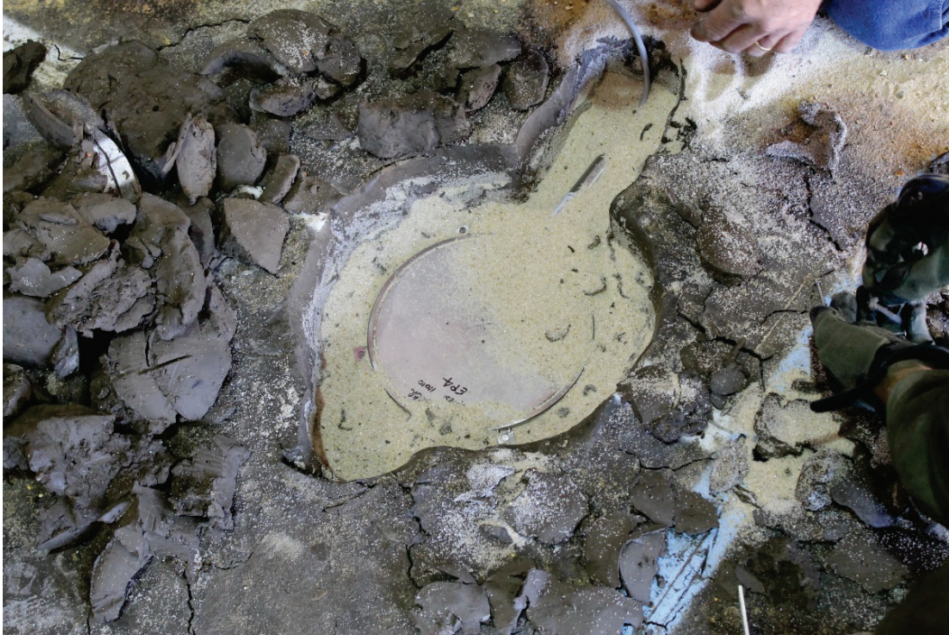
Figure 20. Installation of an EPC.
