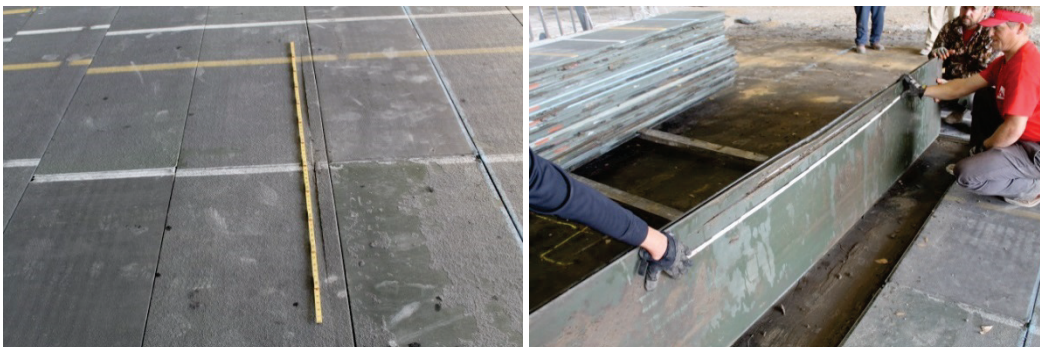
Figure 70. Damage in Panel 103.
