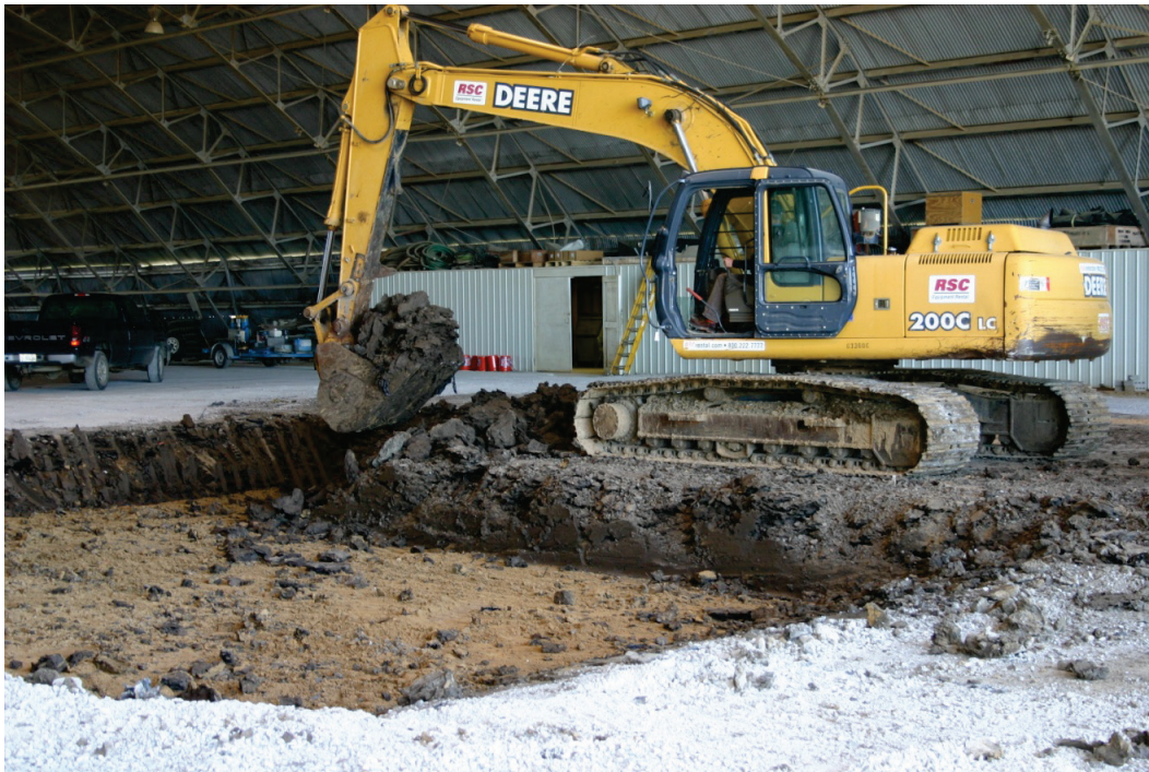
Figure 9. Test section excavation.
