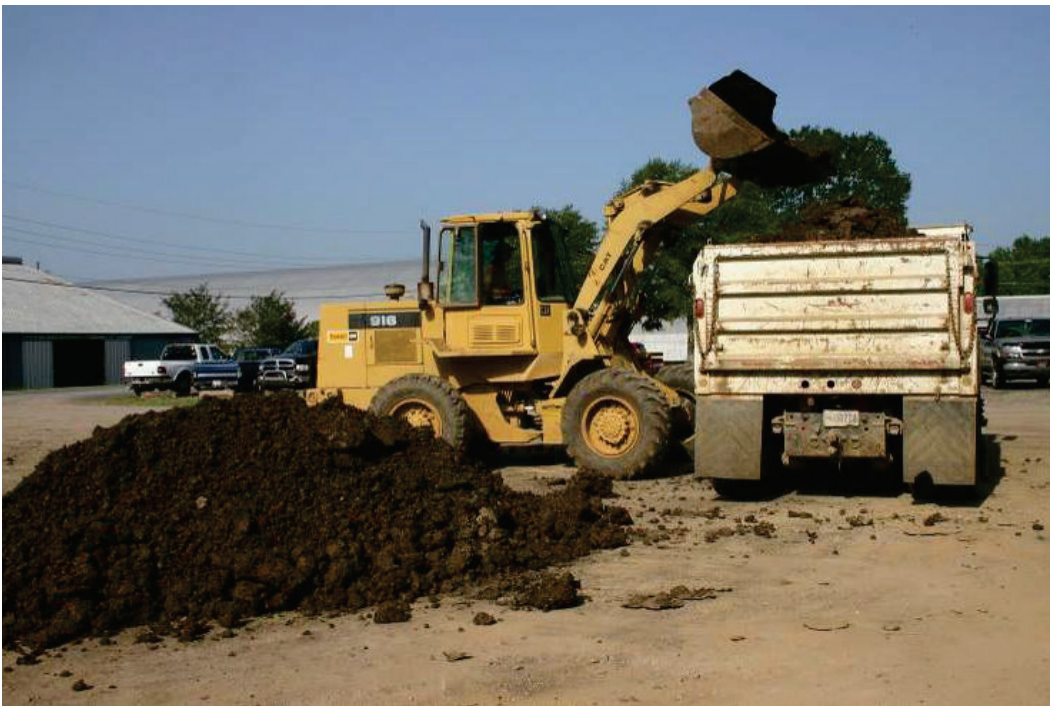
Figure 13. Loading processed CH into haul truck.
