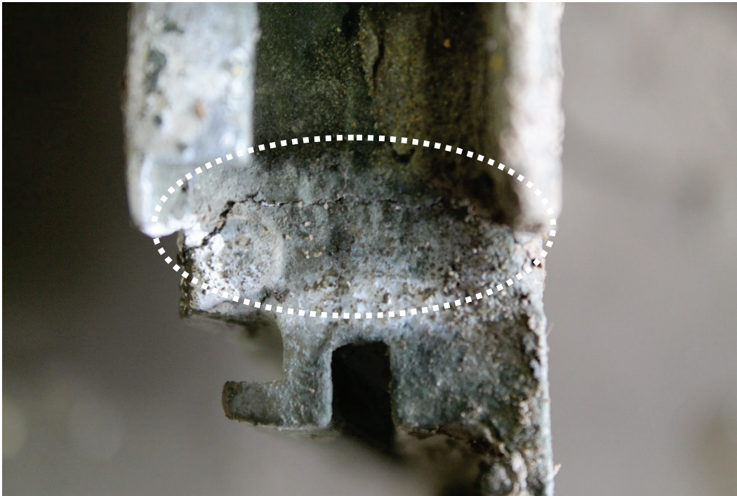
Figure 67. Damage noted in Panel 68 after removing from test section.
