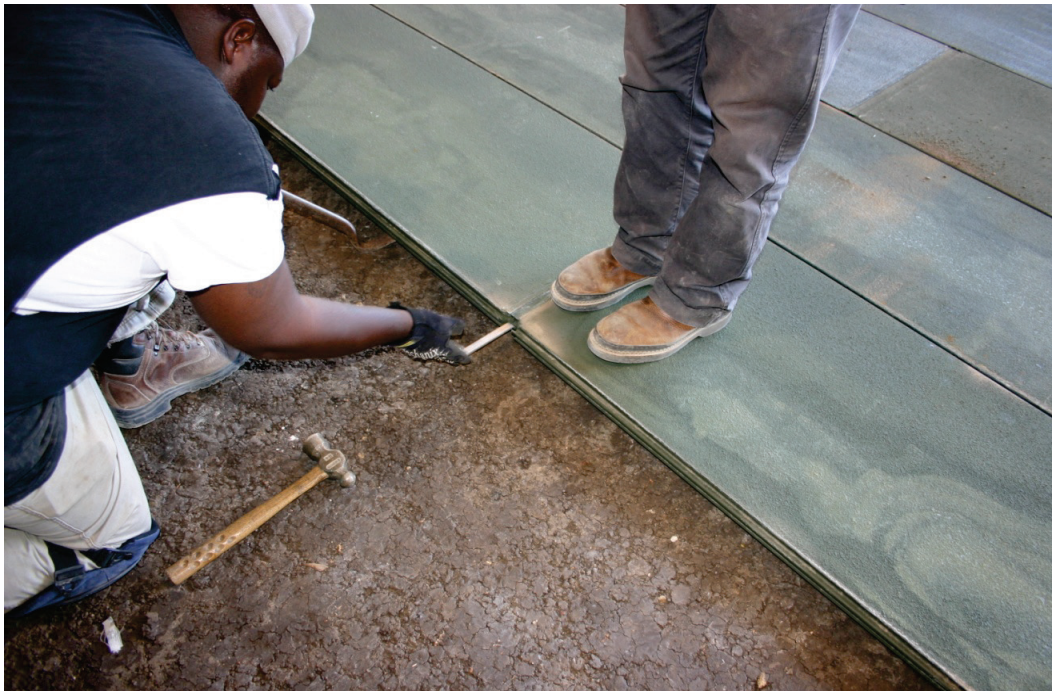
Figure 25. Insertion of aluminum locking bar between adjacent panels.
