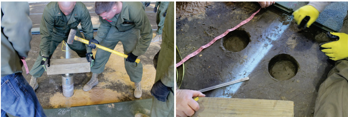
Figure 24. Void installation on subgrade surface.
