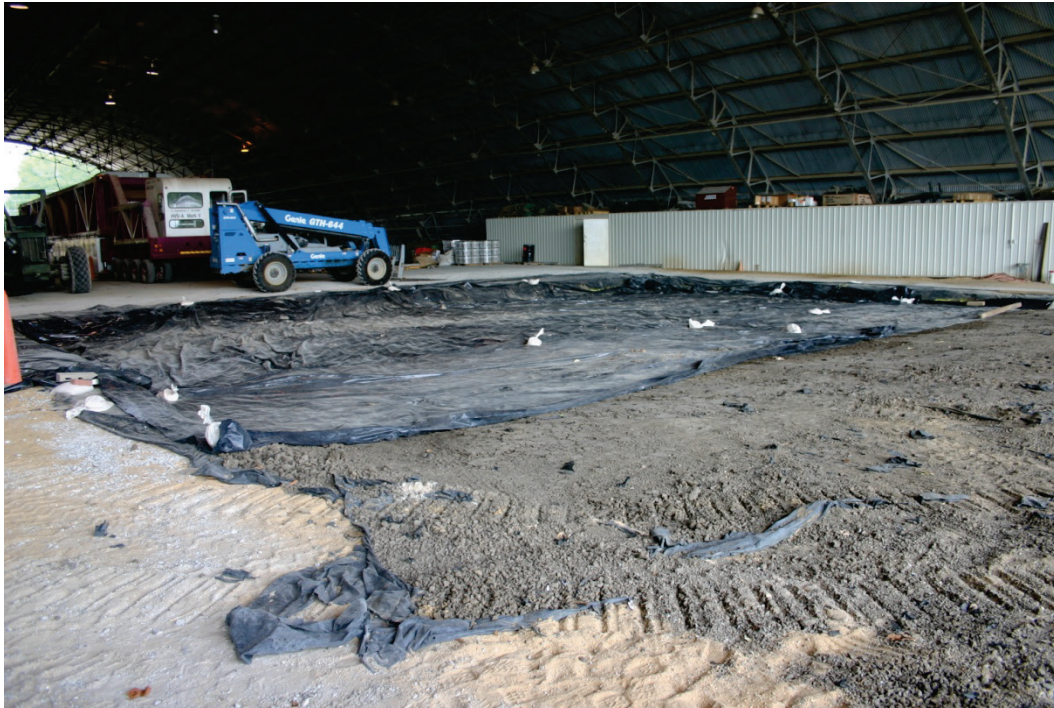
Figure 10. Test pit lined with impervious sheeting.
