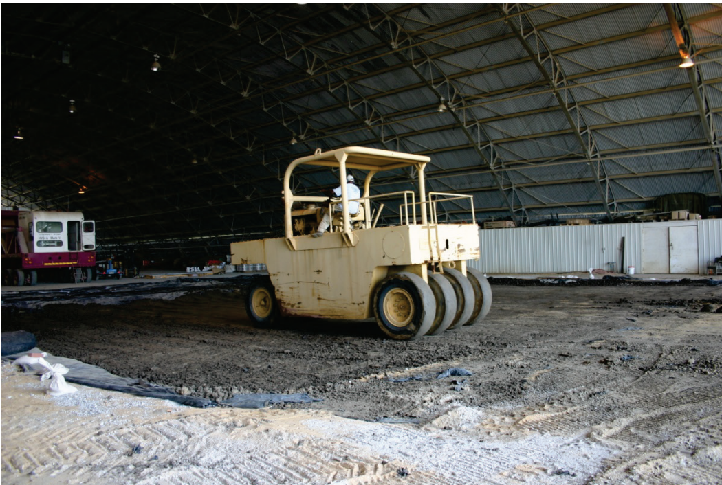
Figure 15. Compacting CH subgrade with pneumatic roller.
