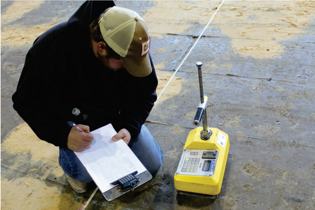
Figure 16. Nuclear moisture-density gauge test.
