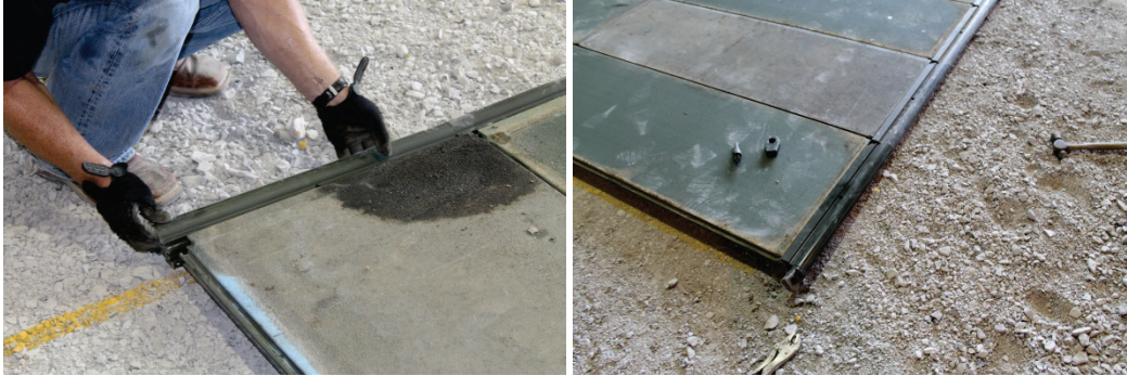
Figure 27. Typical installation of towing to the edges of the test section.
