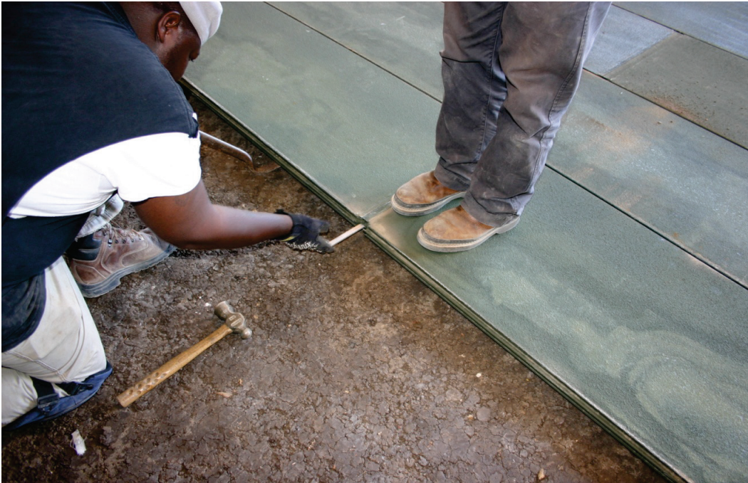
Figure 15. Insertion of aluminum locking bar between adjacent panels.
