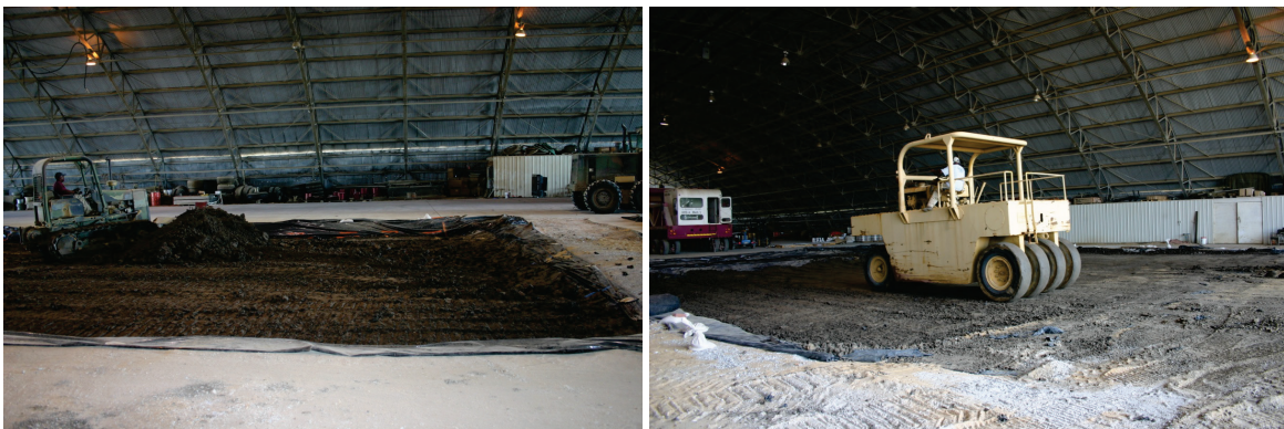
Figure 12. Leveling (left) and compacting (right) CH.
