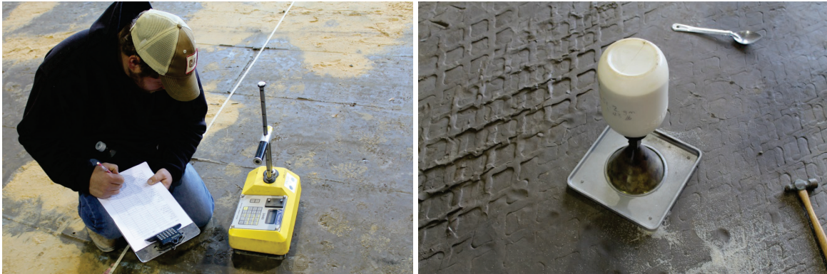
Figure 13. Nuclear gauge (left) and sand cone (right) test.
