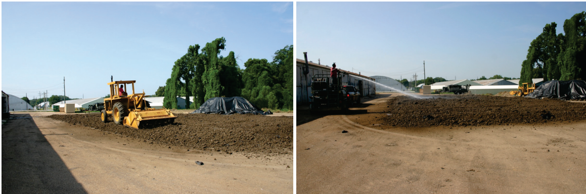
Figure 11. Pulverizing CH (left) and adding moisture (right).
