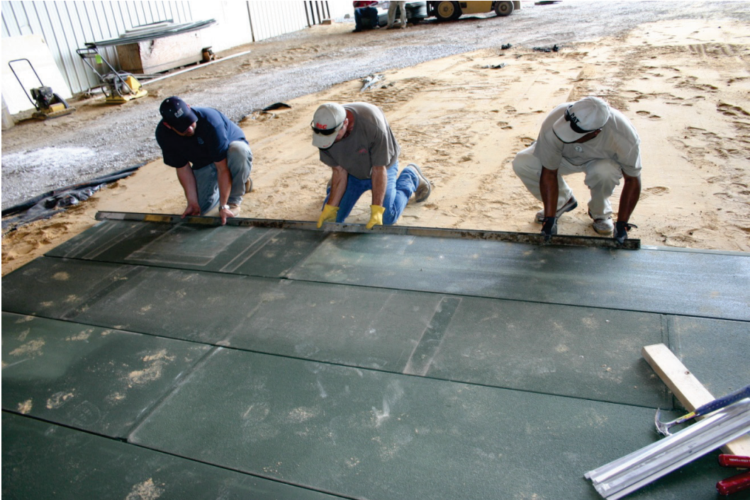
Figure 17. Typical installation of male keylock.
