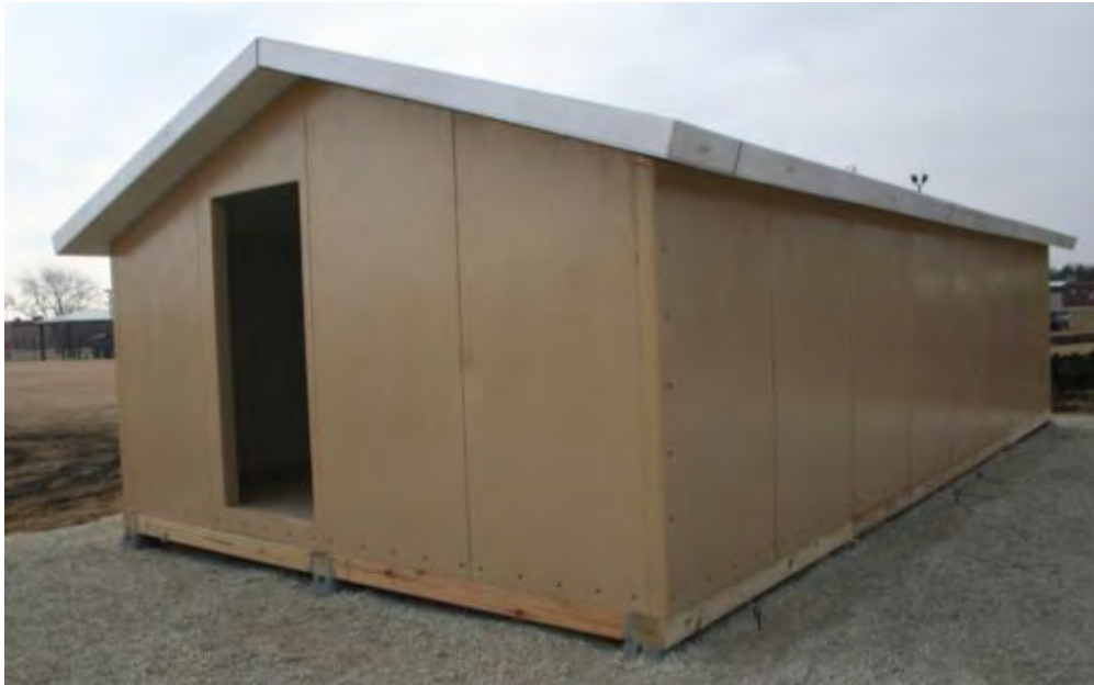
Figure 3-12. SIP hut before finishing.
