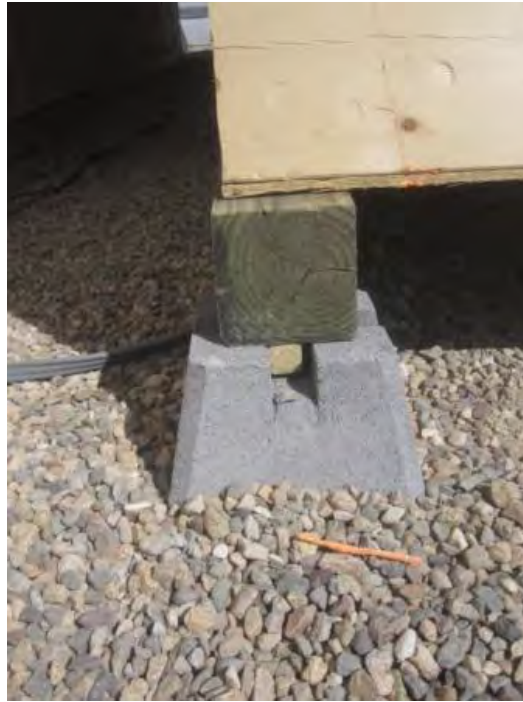
Figure 2-2. Site conditions at Camp Roberts.
