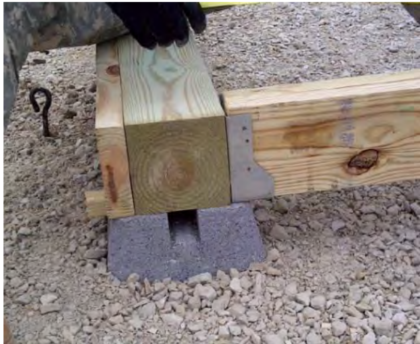
Figure 3-3. Foundation connection detail.
