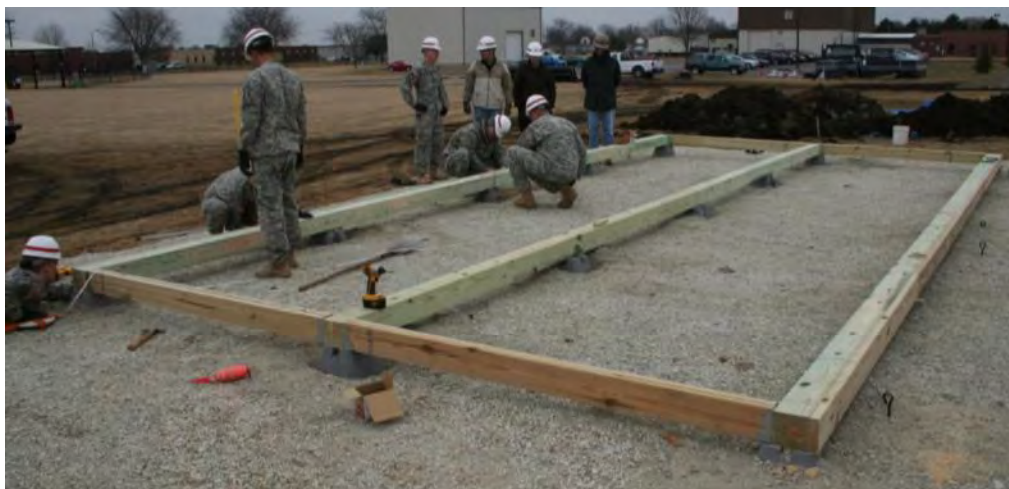
Figure 3-5. Finishing the foundation.
