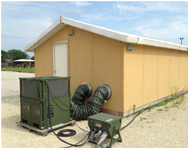
SIP hut and environmental control unit
