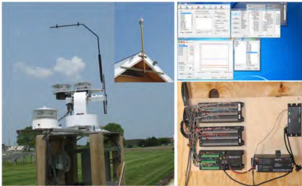
Figure 4-2. Weather station and data acquisition system with remote access capability.
