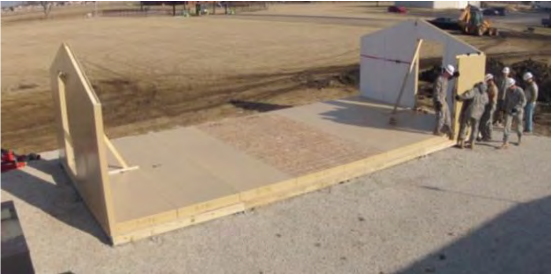
Figure 3-9. SIP hut wall construction.
