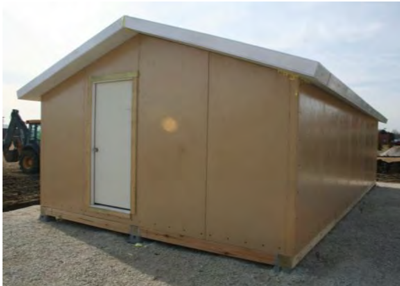
Figure 3-15. Completed SIP hut – north face.
