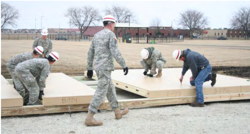
Figure 3-7. Placing floor panels and locking cam-lock.
