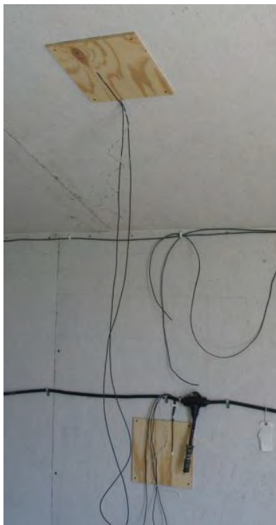
Figure 4-9. HFTs on wall and roof.
