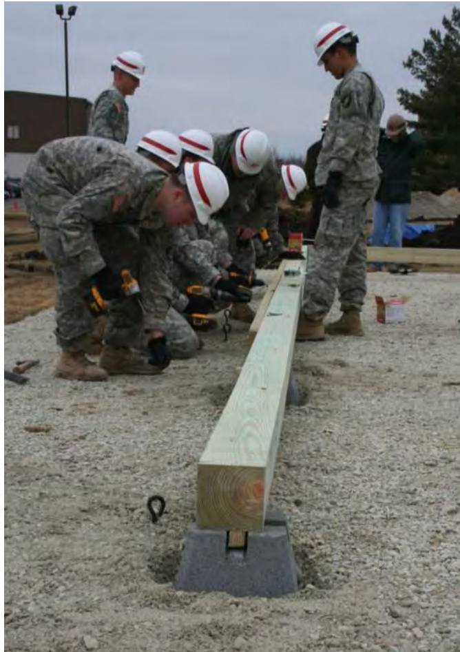
Figure 3-4. Foundation beam cleat.
