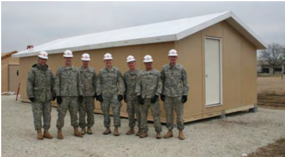
Figure 3-13. Completed SIP hut and partial build crew.
