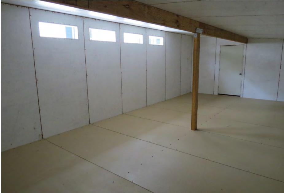
Figure 3-18. SIP hut 4.0 interior showing windows.
