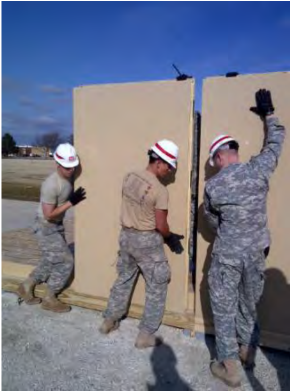
Figure 3-8. Wall panel placement.
