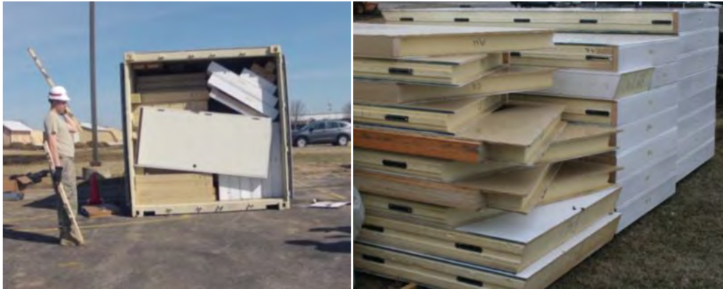
Figure 3-6. SIP unloaded/staged (right).
