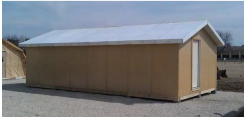
Figure 3-14. Completed SIP hut on CERL's EFOB-L.
