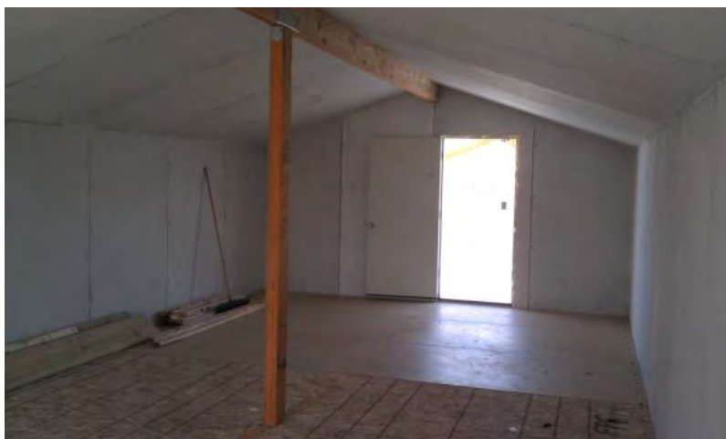
Figure 3-16. Completed SIP hut – Interior.
