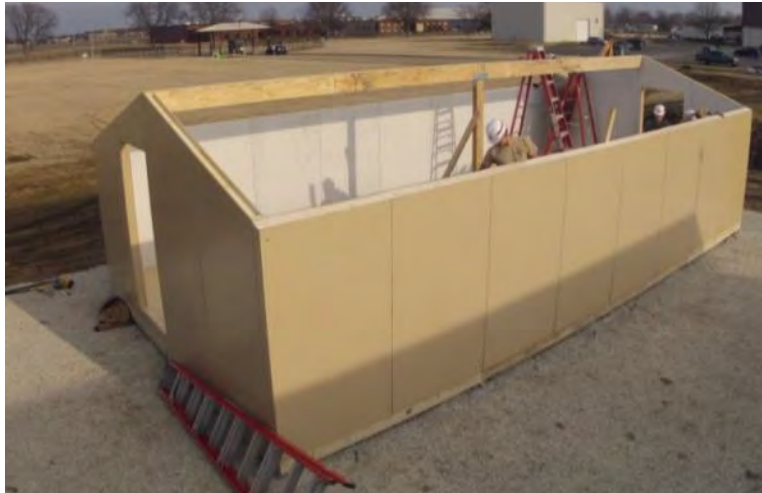
Figure 3-10. SIP hut pre-roof construction.
