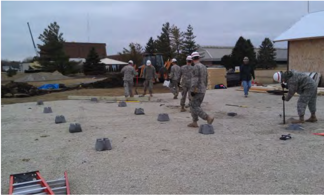
Figure 3-2. Setting up SIP hut foundation piers.
