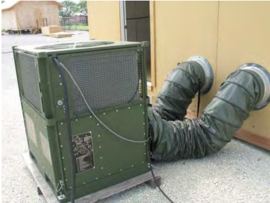
Figure 4-22. IECU serving the SIP hut and the flexible ducts used as supply and return ducts.
