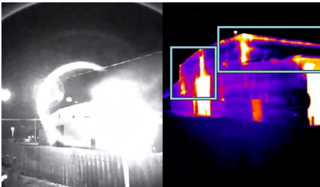
Figure D-46. NIR image (left) and thermal image (right) of Bldg 548, Scott AFB. The large door, upper corner and soffit areas appear to be thermally inefficient.
