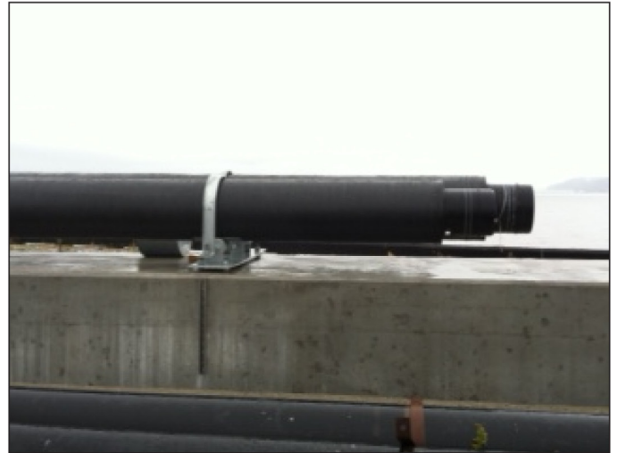
New, strengthened water lines being installed
