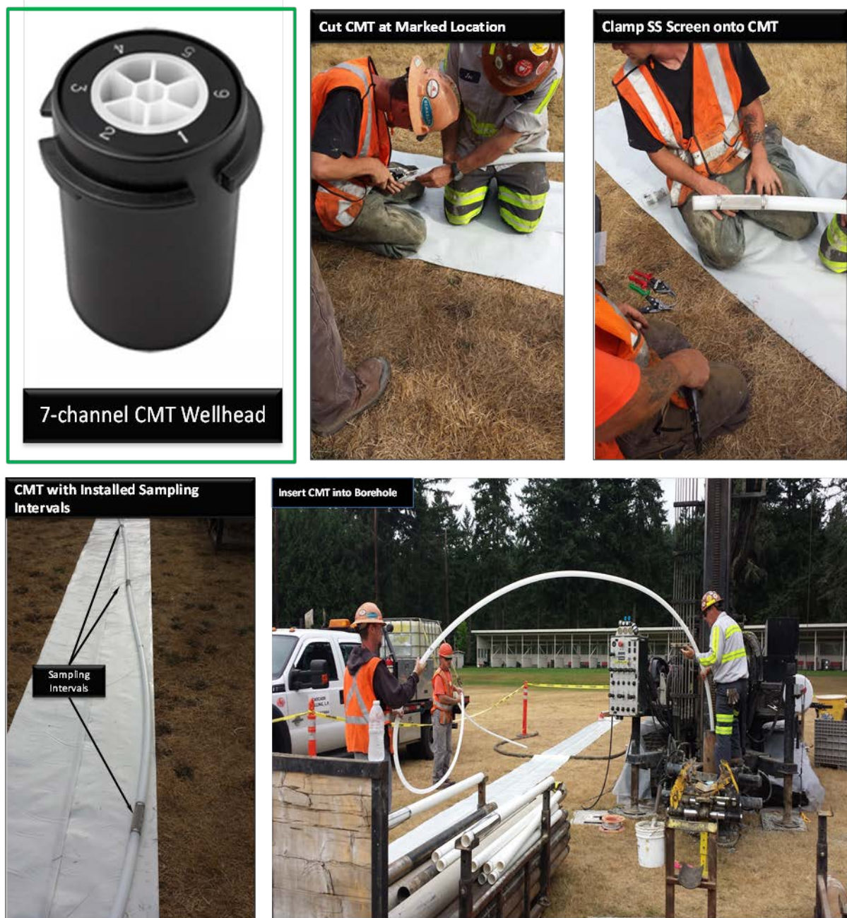
Figure 5.10. CMT well installation during field demonstration. Photos illustrate several key steps (not all steps shown).
