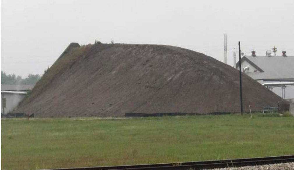
Figure 8. Berm 3A reconfigured, treated with biopolymer for soil stabilization, and seeded with fescue grass.
