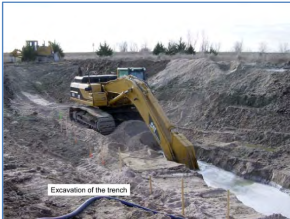
Installation of zero-valent iron (ZVI) PBR at Cornhusker Army Ammunition Plant (AAP), Nebraska (Johnson and Tratnyek, 2008).
