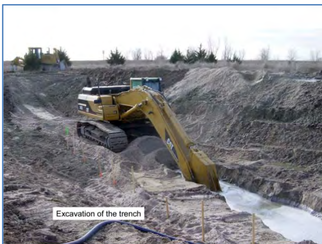
Installation of zero-valent iron (ZVI) passive in situ mitigation approach at Cornhusker Army Ammunition Plant (AAP), Nebraska (Johnson and Tratnyek, 2008).
