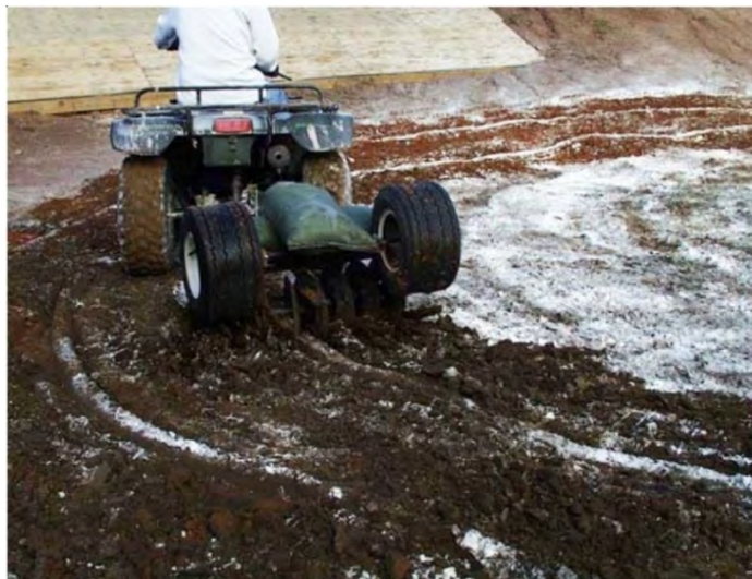
Figure 5-1. Lime incorporation using a disc at Fort Jackson (from Larson et al., 2007a).
