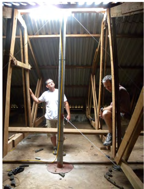
Figure 4 – Site ZNZB. (upper left) antenna on the self-center mounting device installed on the top of a mast; (right) mast inside of the roof solidly linked to the structure (wires used to tension the mast); (lower left) installation team with the antenna on the background.
