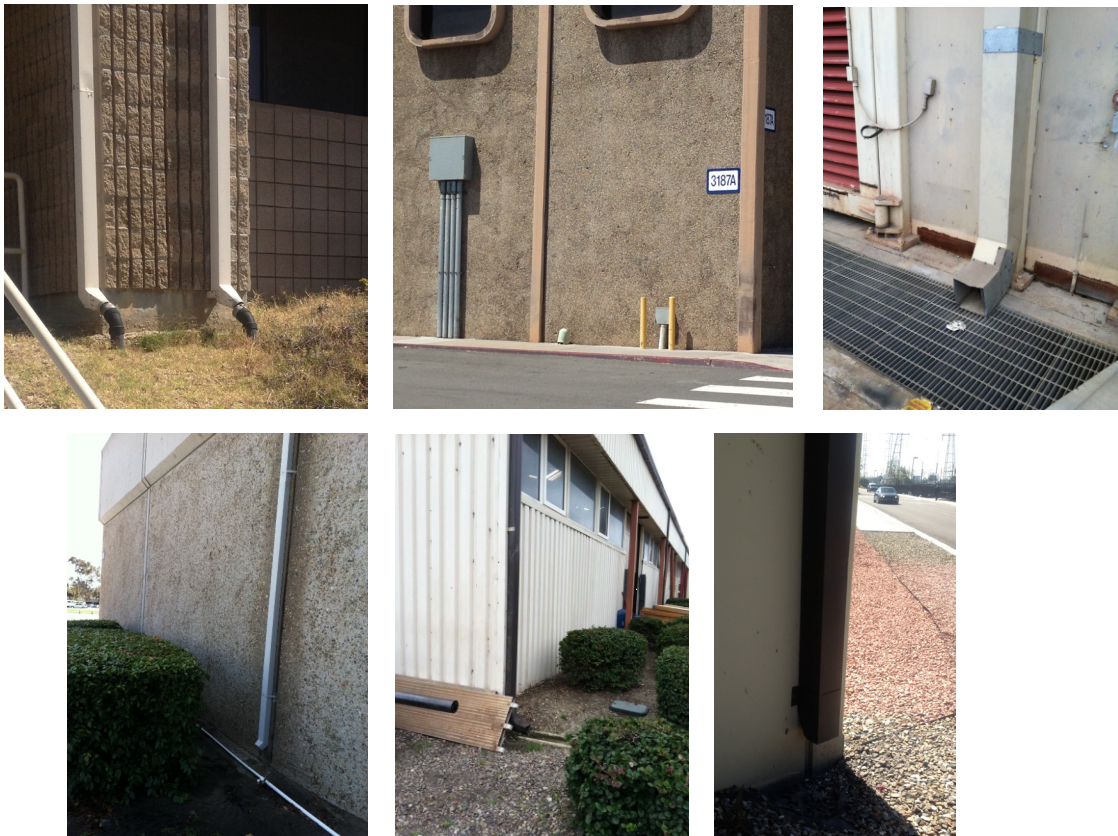
Figure 8. Examples of roofs directly connected to the storm-water conveyance system (top) and those disconnected that drain to vegetation, soil, or stone-filled infiltration areas like those shown in the bottom photos.
