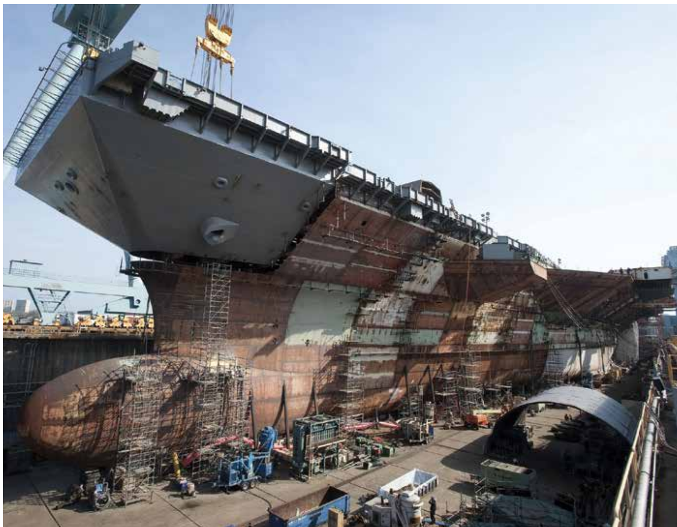
Increasing the amount of construction work done on CVN 79 prior to erection will lead to efficiencies and cost savings. NNS photo
