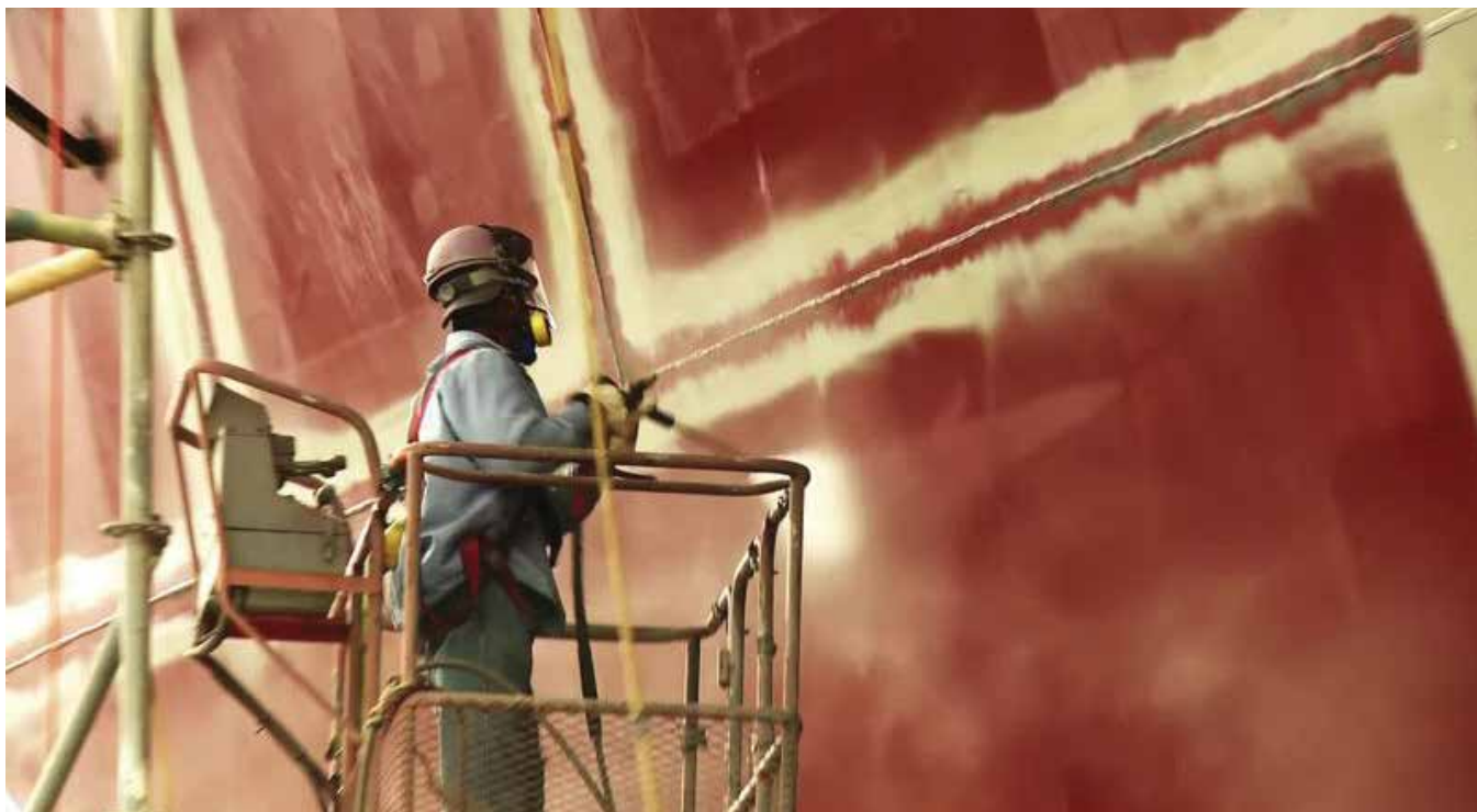
A motion-assisted positioning device used for the blasting process will reduce costs and worker fatigue, and increase throughput on multiple naval platforms. Ingalls photo
