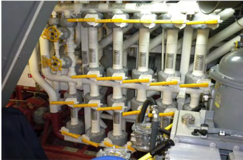
Figure 2. Fuel Management/handling System
