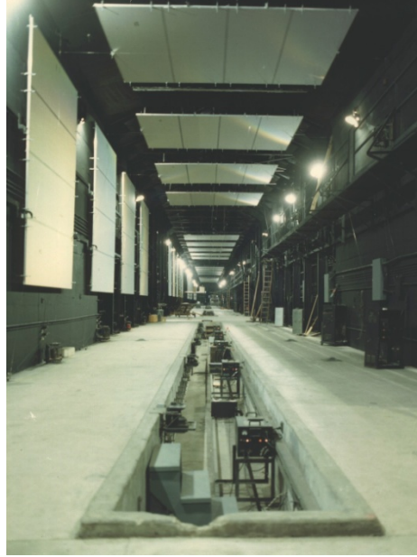
Fig. 3 Spark range facility
